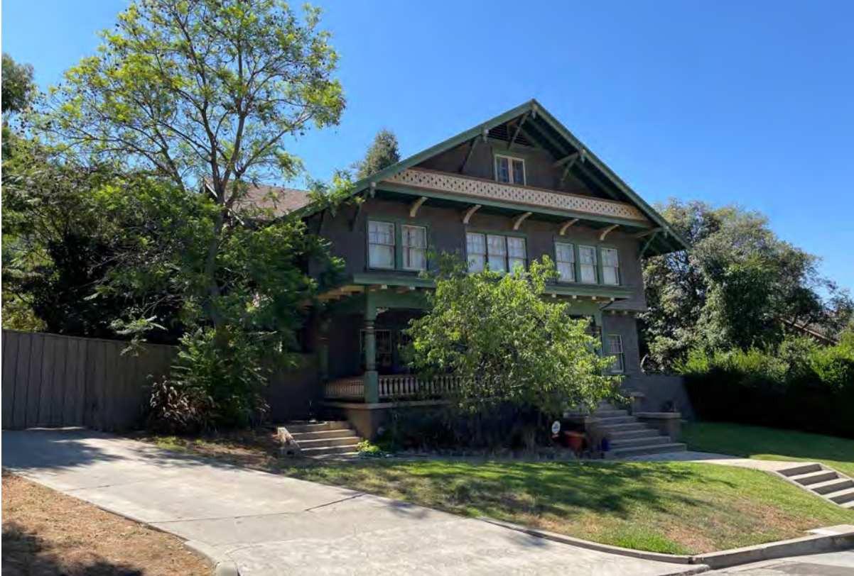
Figure 4 Overview of façade, southeast perspective
