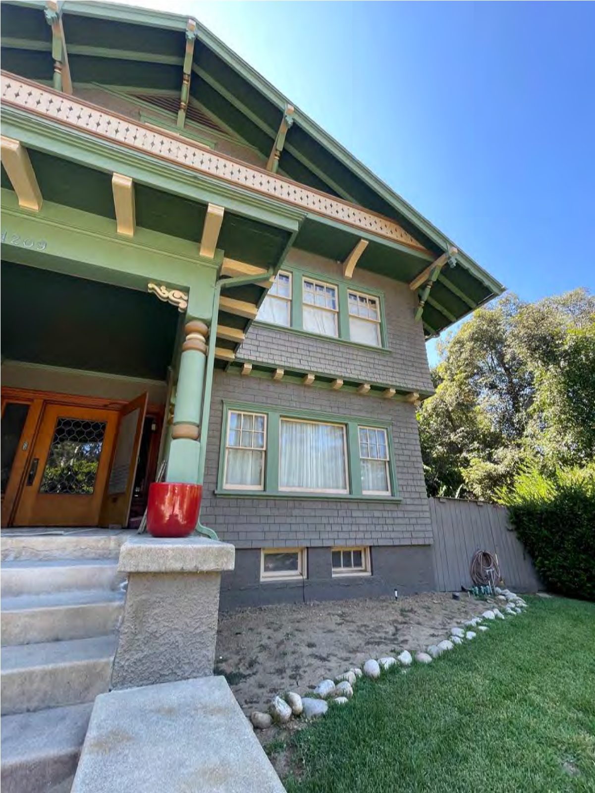
Figure 6 Façade detail, east perspective
