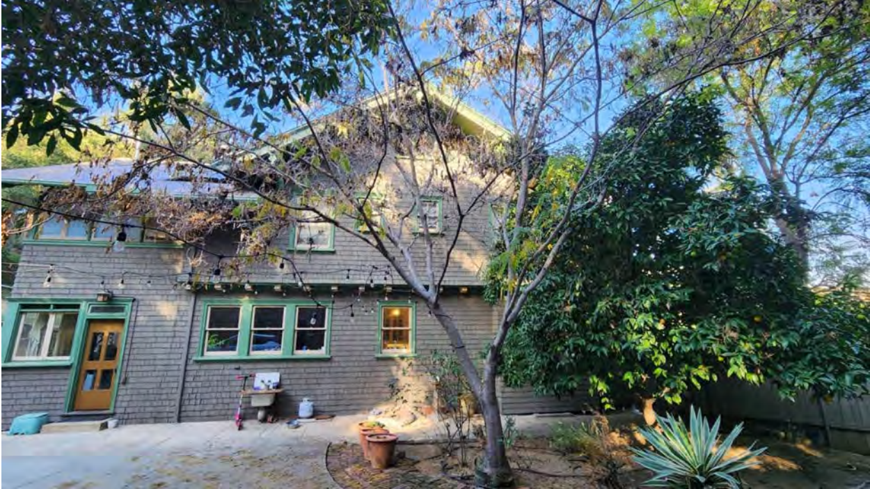
Figure 6 South elevation overview, southern perspective (shows roof cross-gable and addition)
