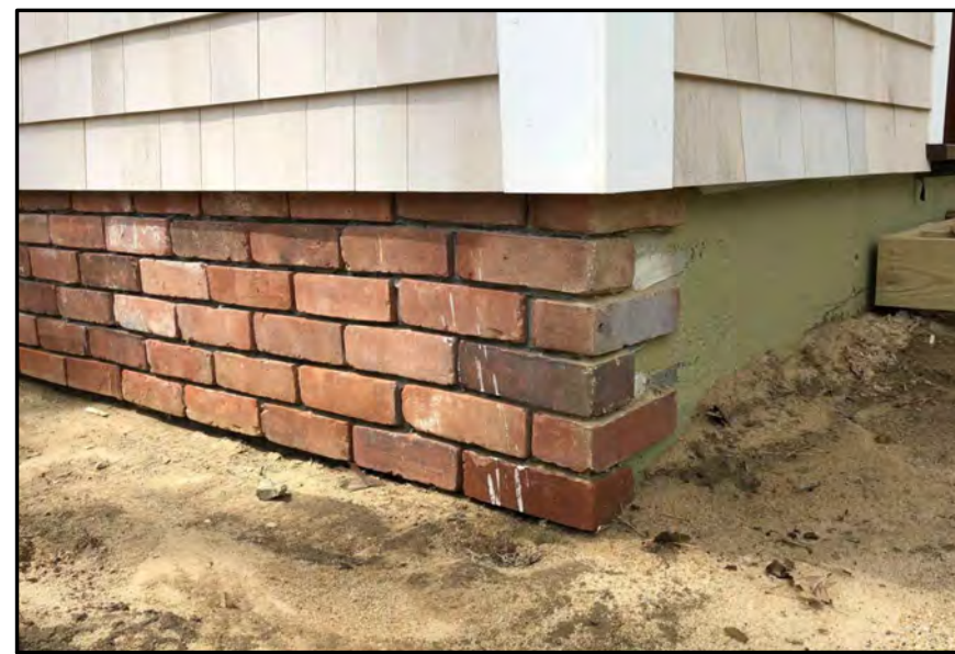
BRICK VENEER ON FOUNDATION WALLS TO MATCH EXISTING FOUNDATION
