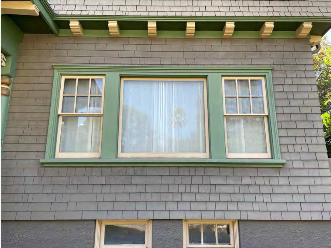
Figure 12 Tripartite wood windows and flared second-story base marked with faux, carved purlins, façade, east perspective
