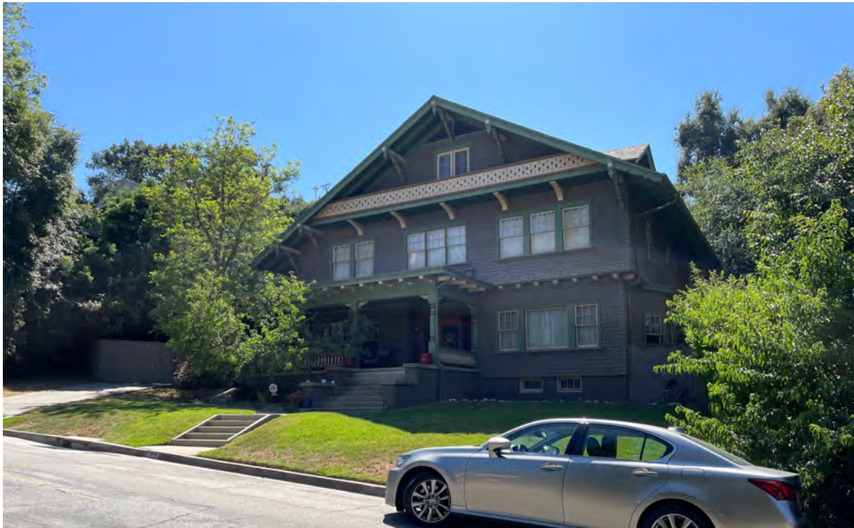
Overview of sloped, hillside parcel, façade, northeast perspective
