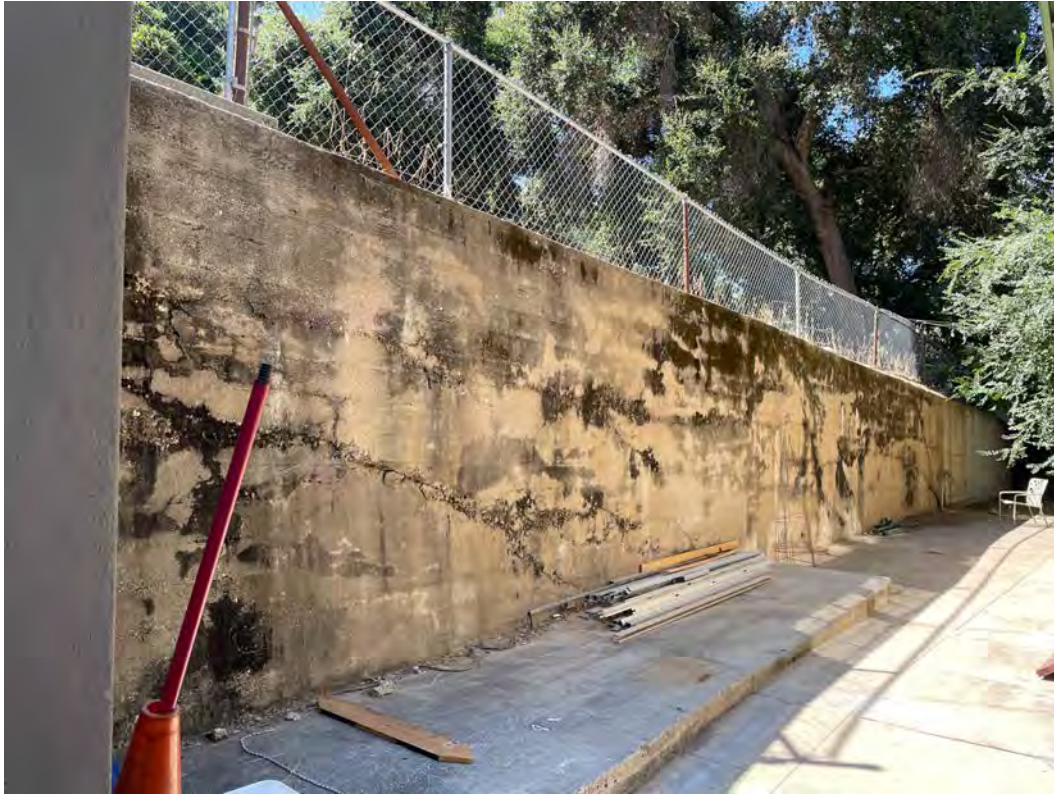
Figure 8 Detail of cracks and water penetration in retaining wall, south perspective
