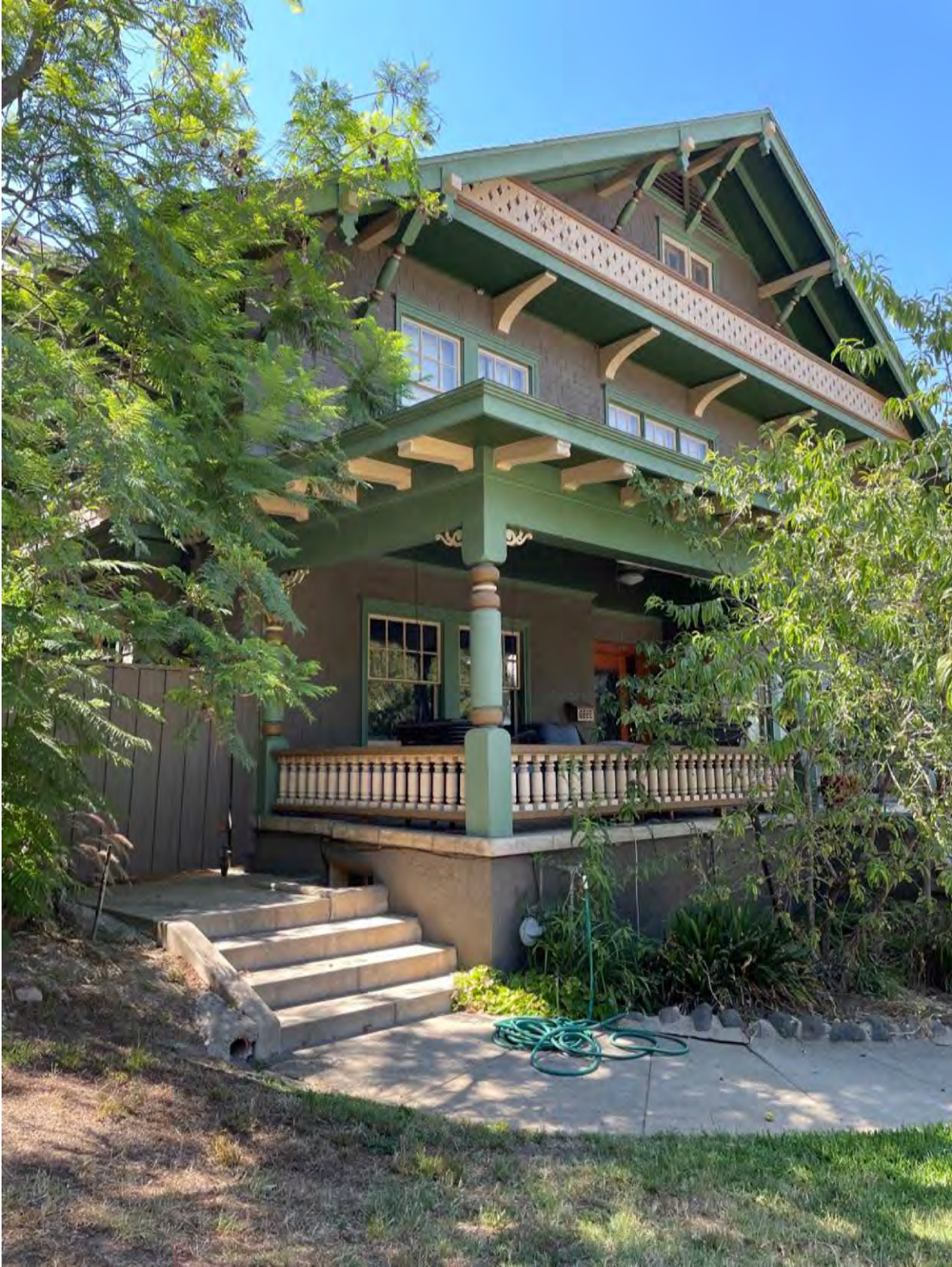
Figure 8 Swiss Chalet/Craftsman character-defining features on the façade, with decorative wood accents throughout the patio, second-story porch railing with geometric cut-outs, and wide wood roof eaves with decorative detailing, southeast perspective
