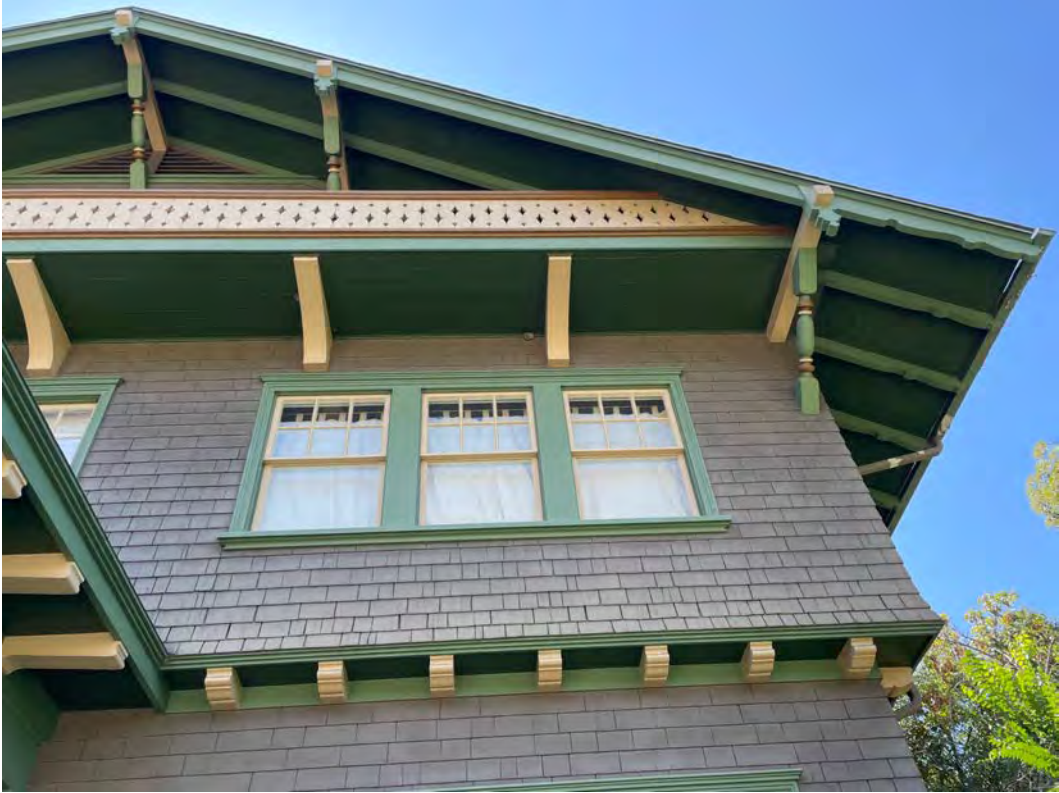
Figure 12 Tripartite wood windows and flared second-story base marked with faux, carved purlins, façade, east perspective
