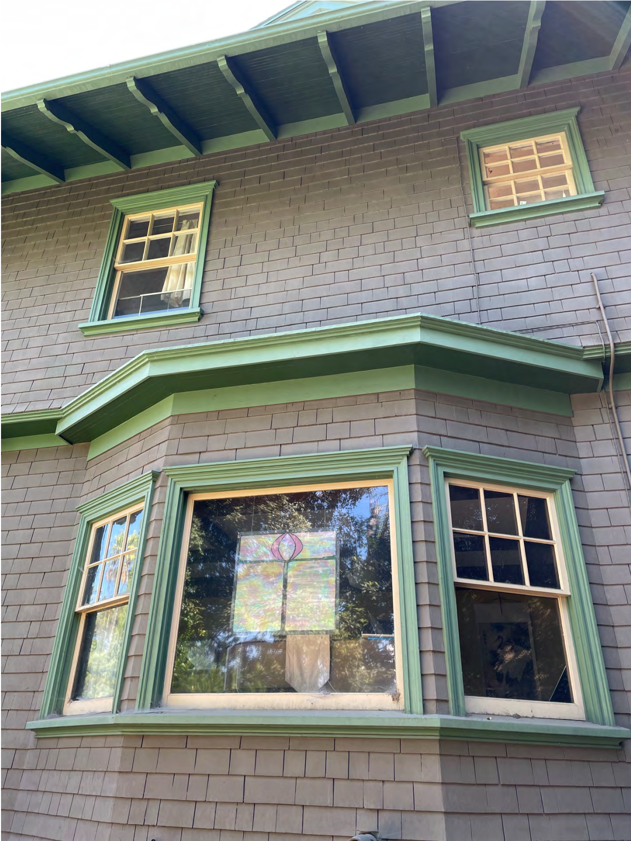
Figure 14 North elevation bay window, wood shingles, and window detailing, north perspective
