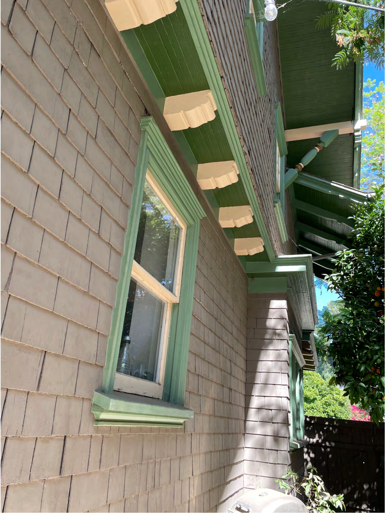
Figure 16 Detail of south elevation windows, triangular knee braces, and decorative carved brackets marking division between first and second stories, southwest perspective
