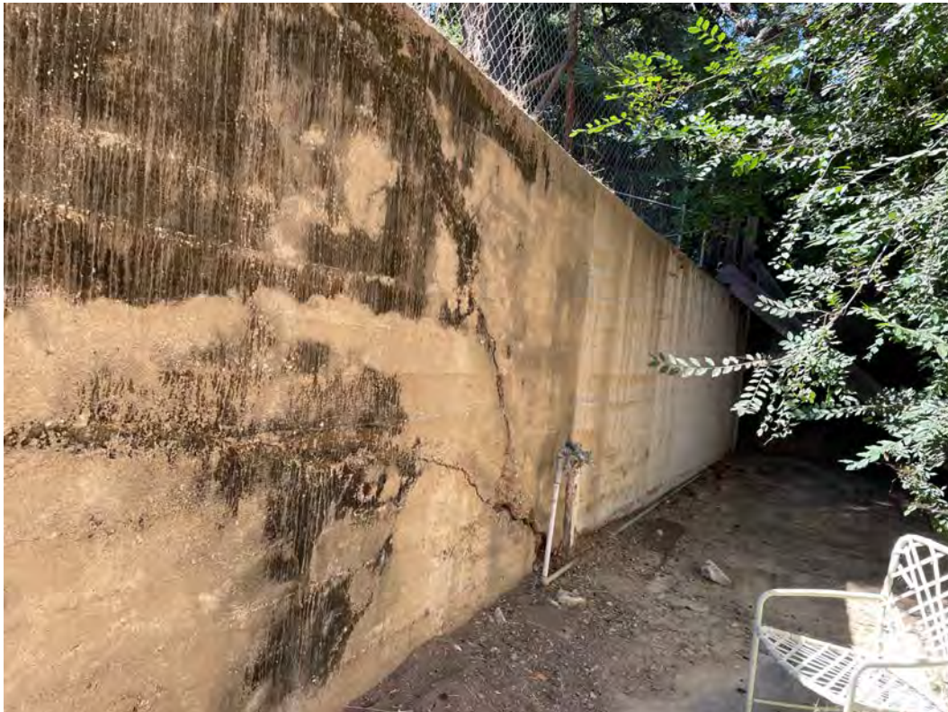
Figure 8 Detail of cracks and water penetration in retaining wall, south perspective
