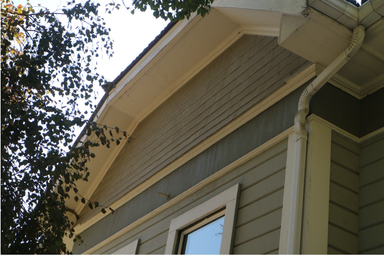
Figure 13 Detail of coursed wood shingles accenting gable apex and vertical plank band
