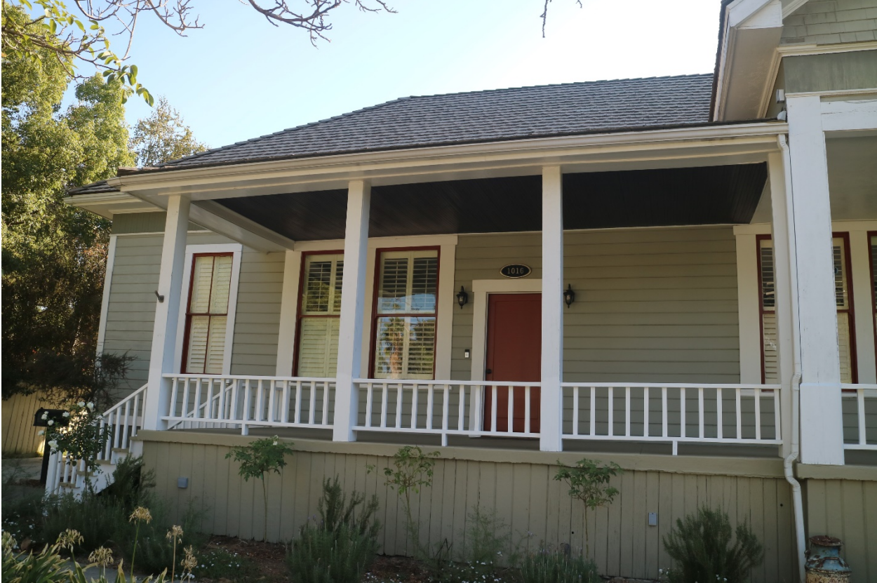
Figure 9 Detail of vertical-plank sheathing on foundation
