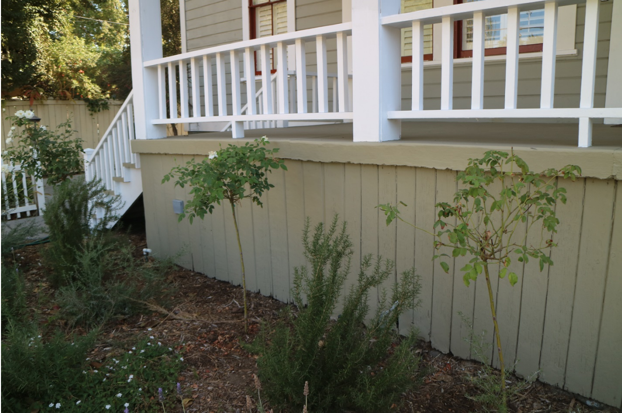
Figure 9 Detail of vertical-plank sheathing on foundation
