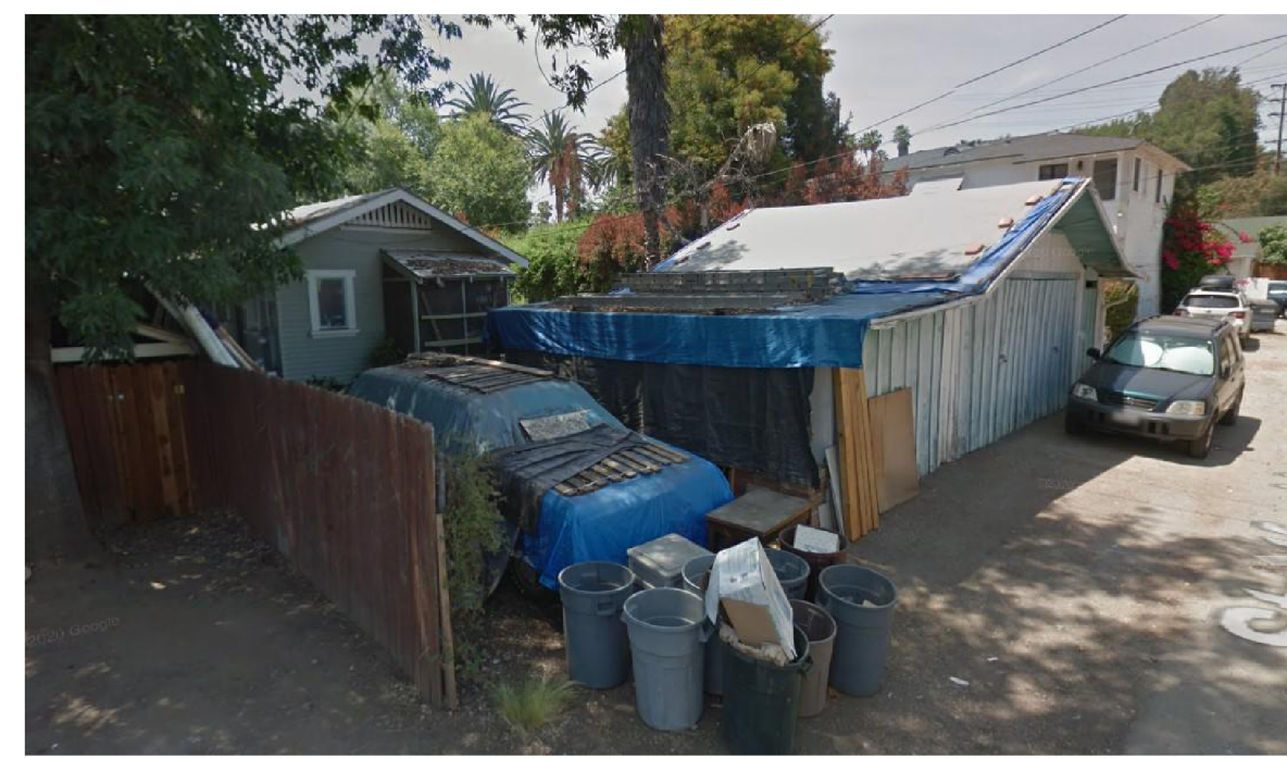
LOOKING NORTHWEST (EXISTING)
