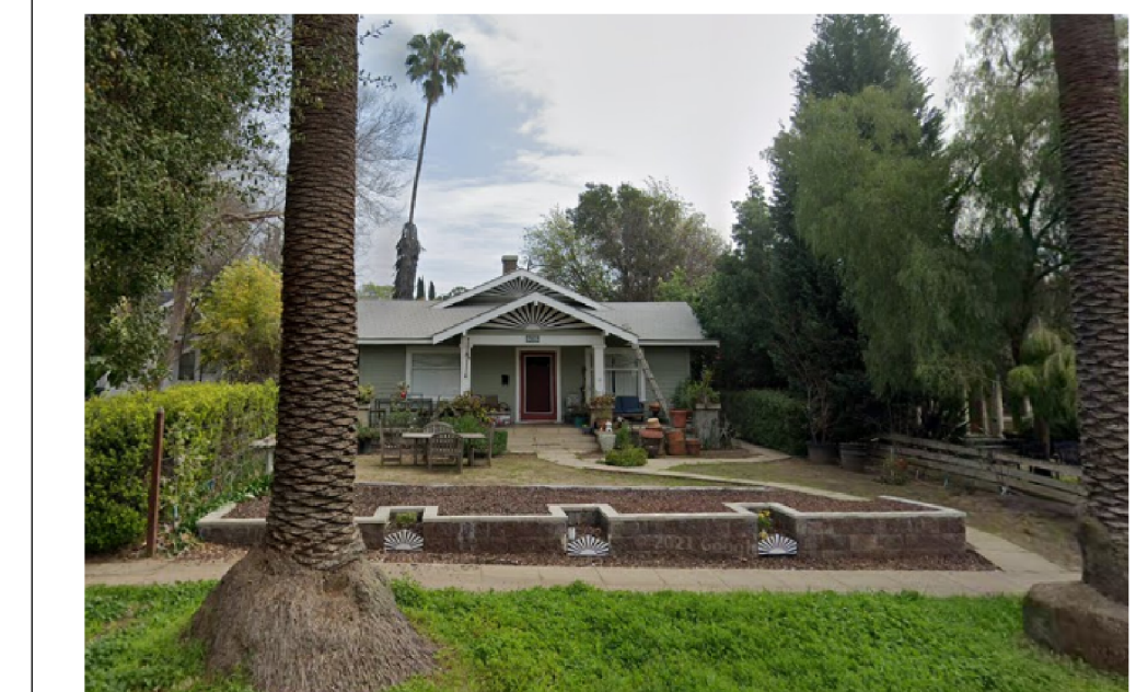
626 STRATFORD AVE. - WEST ELEVATION
