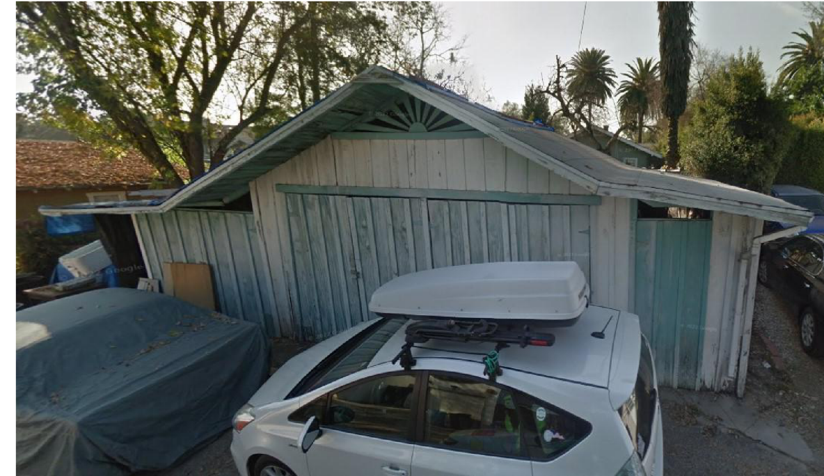
LOOKING WEST (EXISTING)
