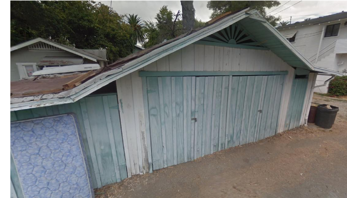
LOOKING NORTHWEST (EXISTING)
