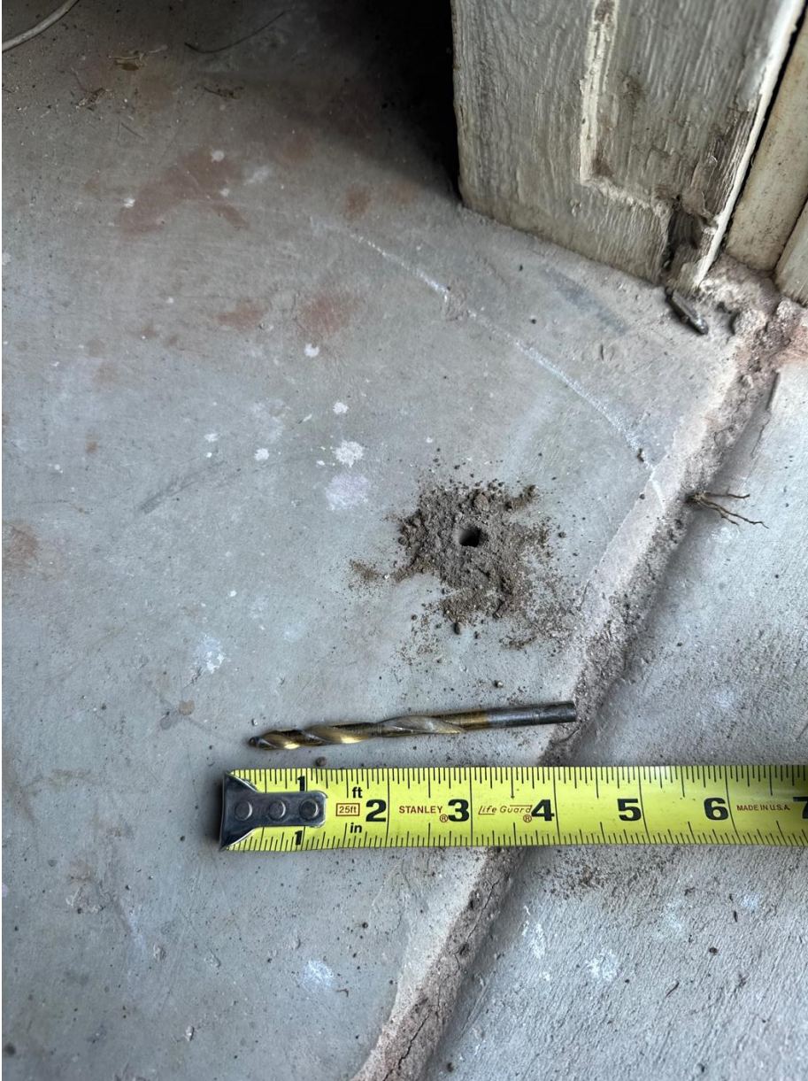
Showing thickness of concrete pad
