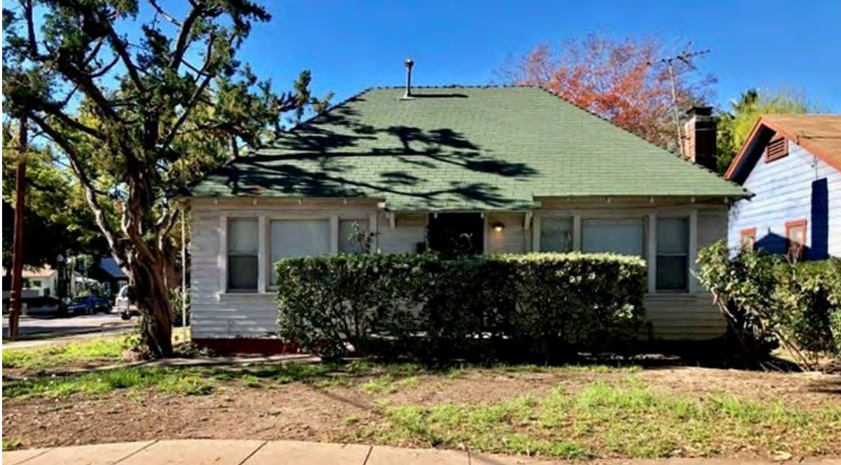
Figure 6 Façade, east perspective (prior to demolition)
