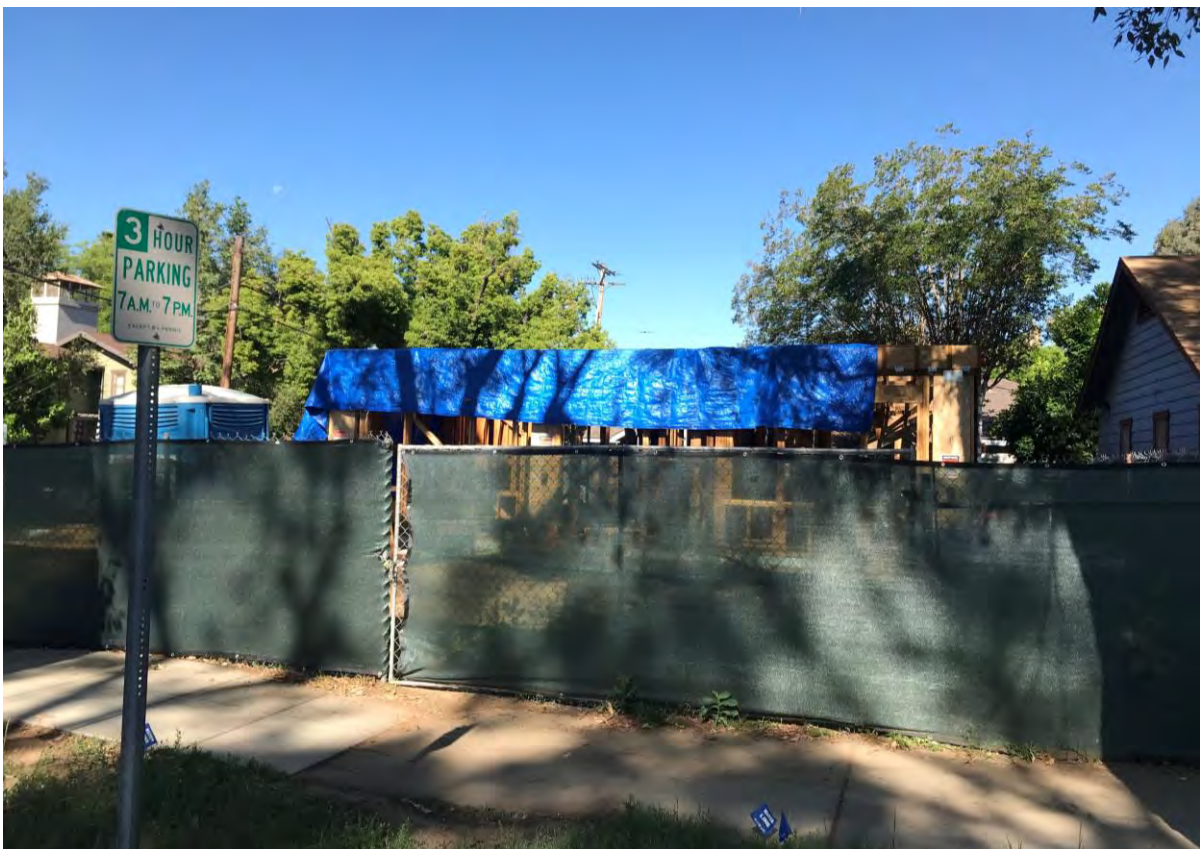
Figure 7 Façade, current condition, east perspective
