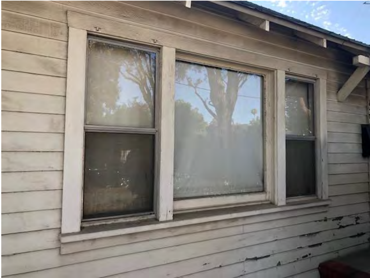
Figure 11 Detail, tripartite, wood-framed windows on façade
