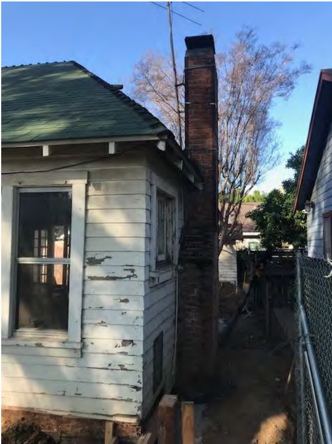
Figure 10 North elevation and brick chimney
