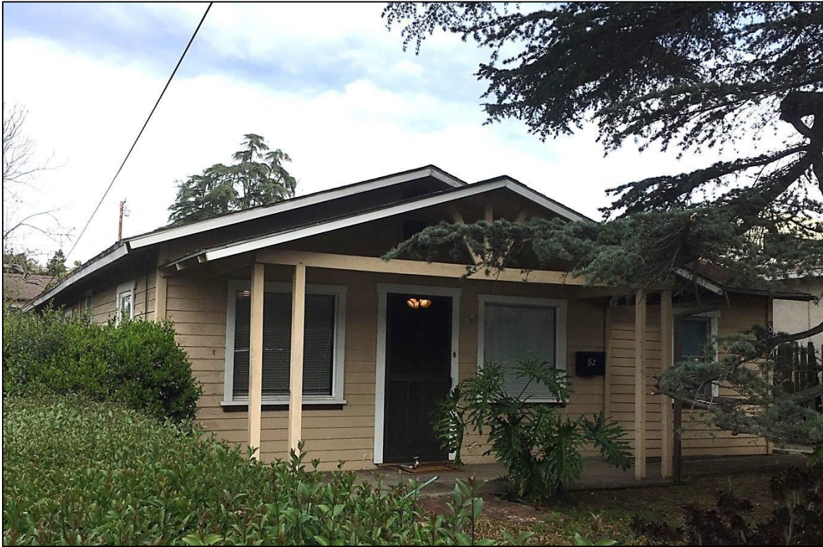
Figure 2 South (façade) elevation, from the southwest (top) and southeast (bottom) perspective, showing addition to property
