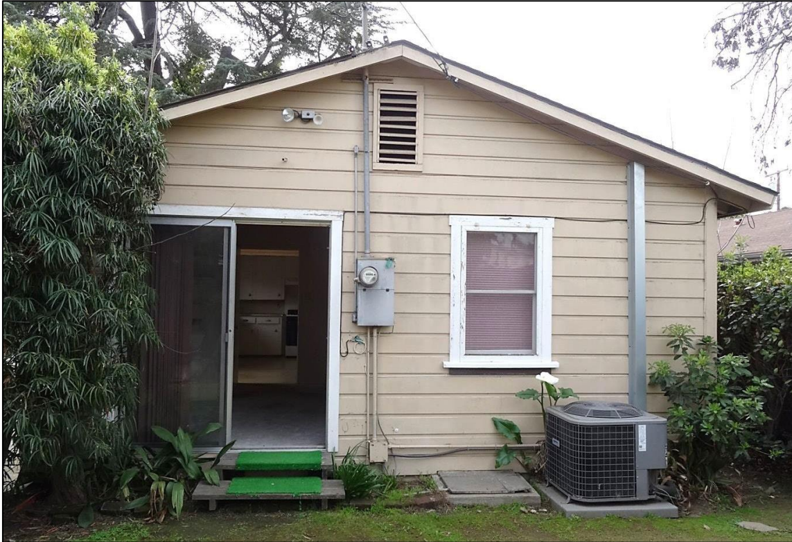
Figure 4 Overview of rear elevation (top) and garage, constructed in 1982 (bottom)
