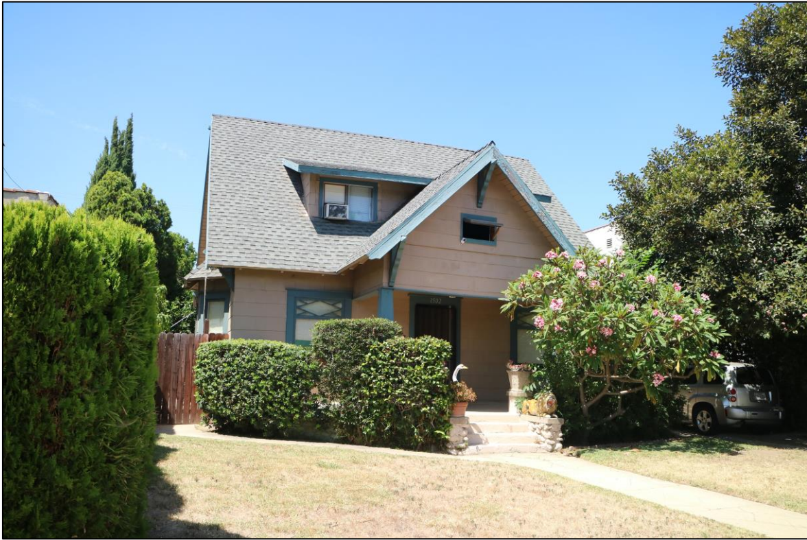
Figure 2 South (façade) elevation, from the southwest (top) and southeast (bottom) perspectives
