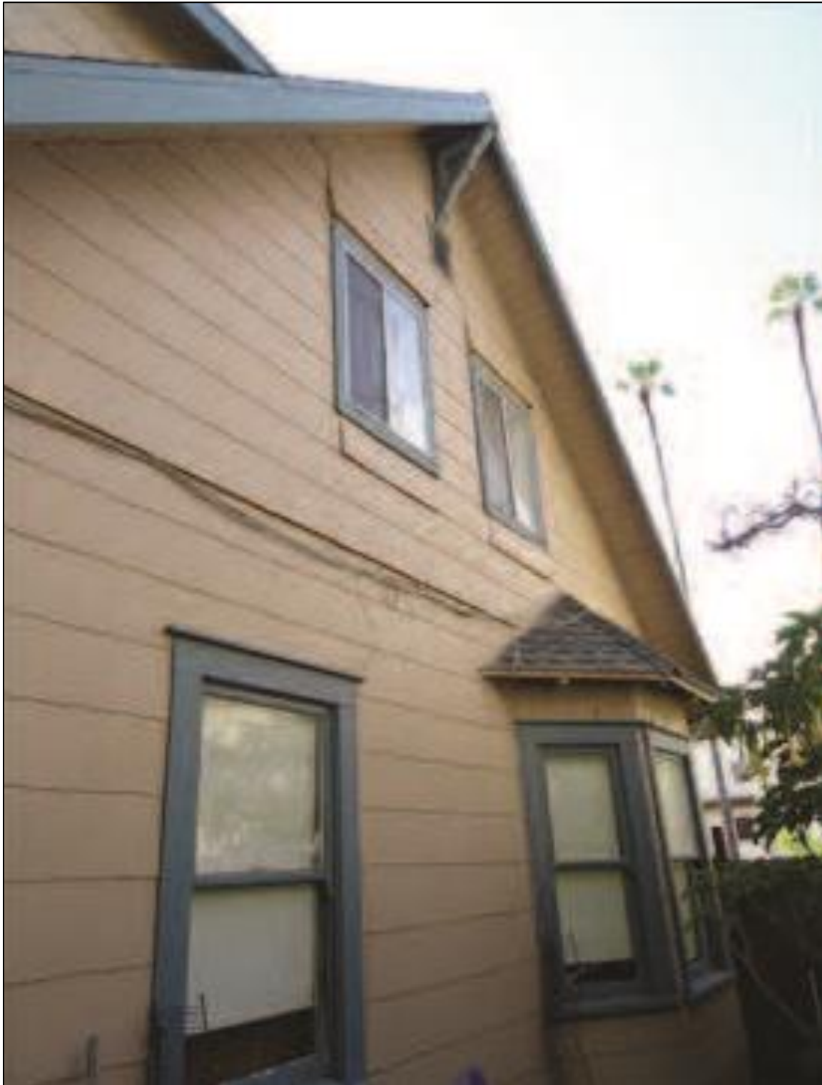
Figure 5 Detail of side (west) elevation and bay window, northwest perspective
