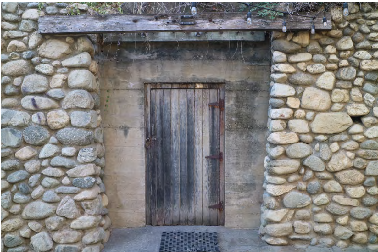
Figure 10 Wine cellar/root cellar in arroyo stone wall (north perspective)
