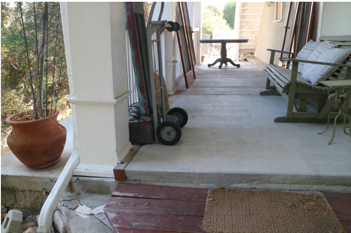
Figure 17 North elevation porch detail, 335 Monterey Road (west perspective)
