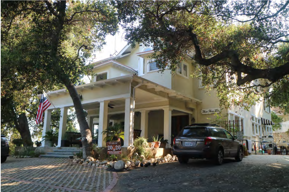
Figure 1 Primary elevation, 335 Monterey Road (southwest perspective)
