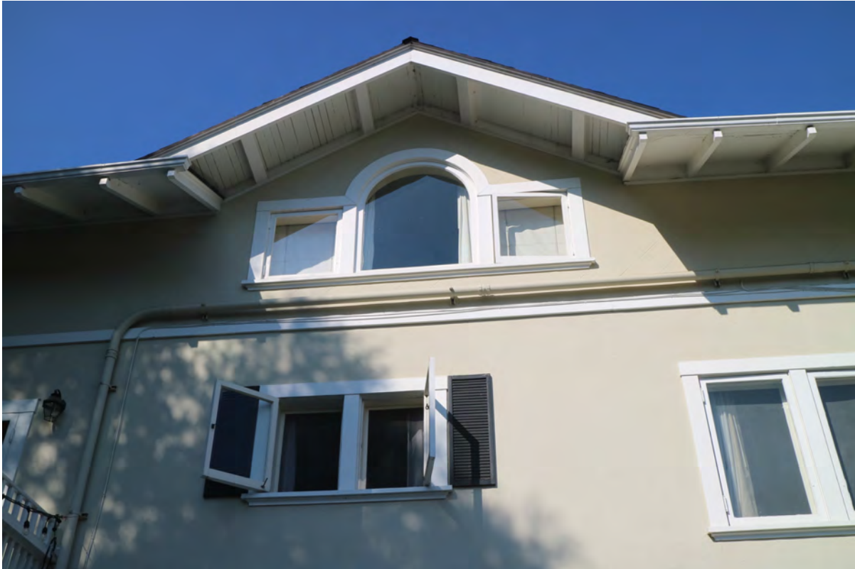
Figure 14 Roofline and window detail, rear elevation (east perspective)
