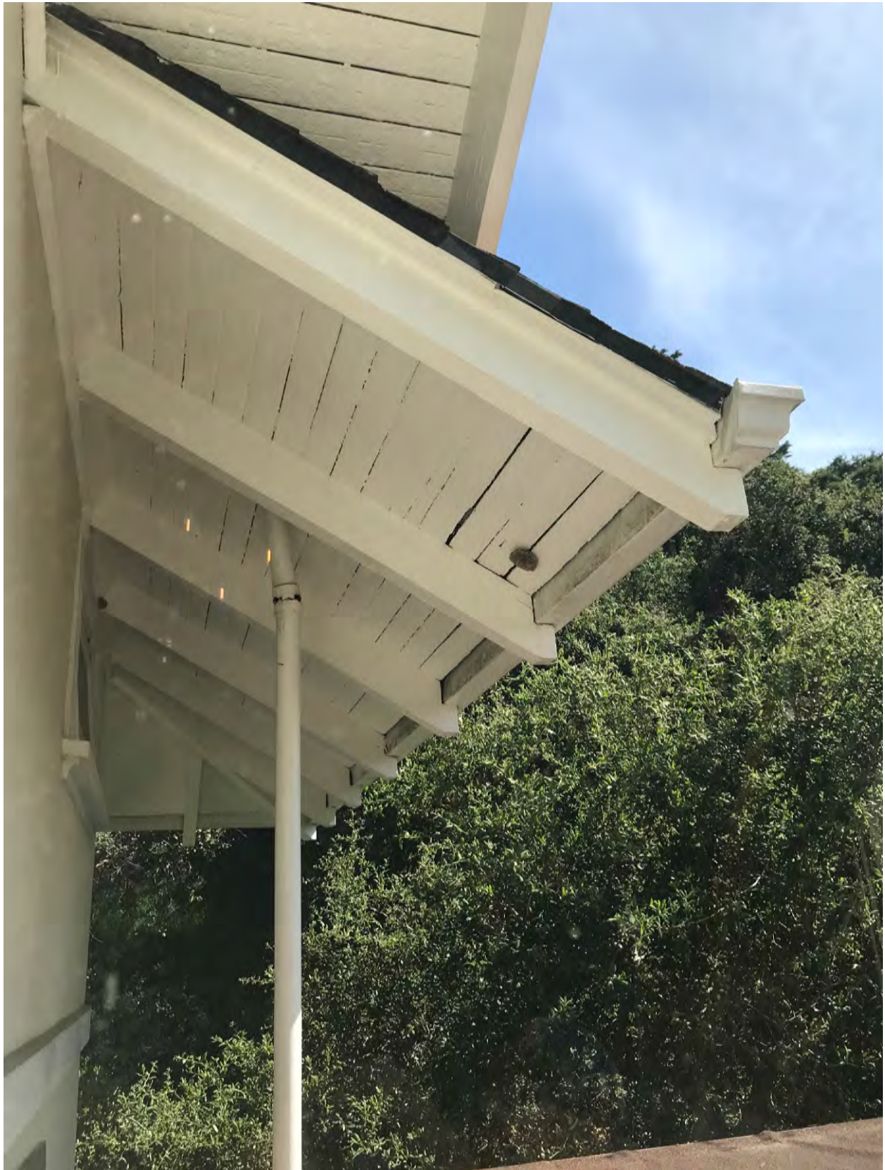
Figure 13 Detail of roof eaves, rafters, and wood-plank ceilings
