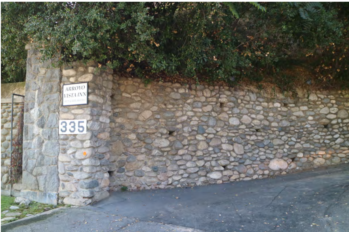
Figure 21 Arroyo stone wall, entrance to 335 Monterey Road (north perspective)
