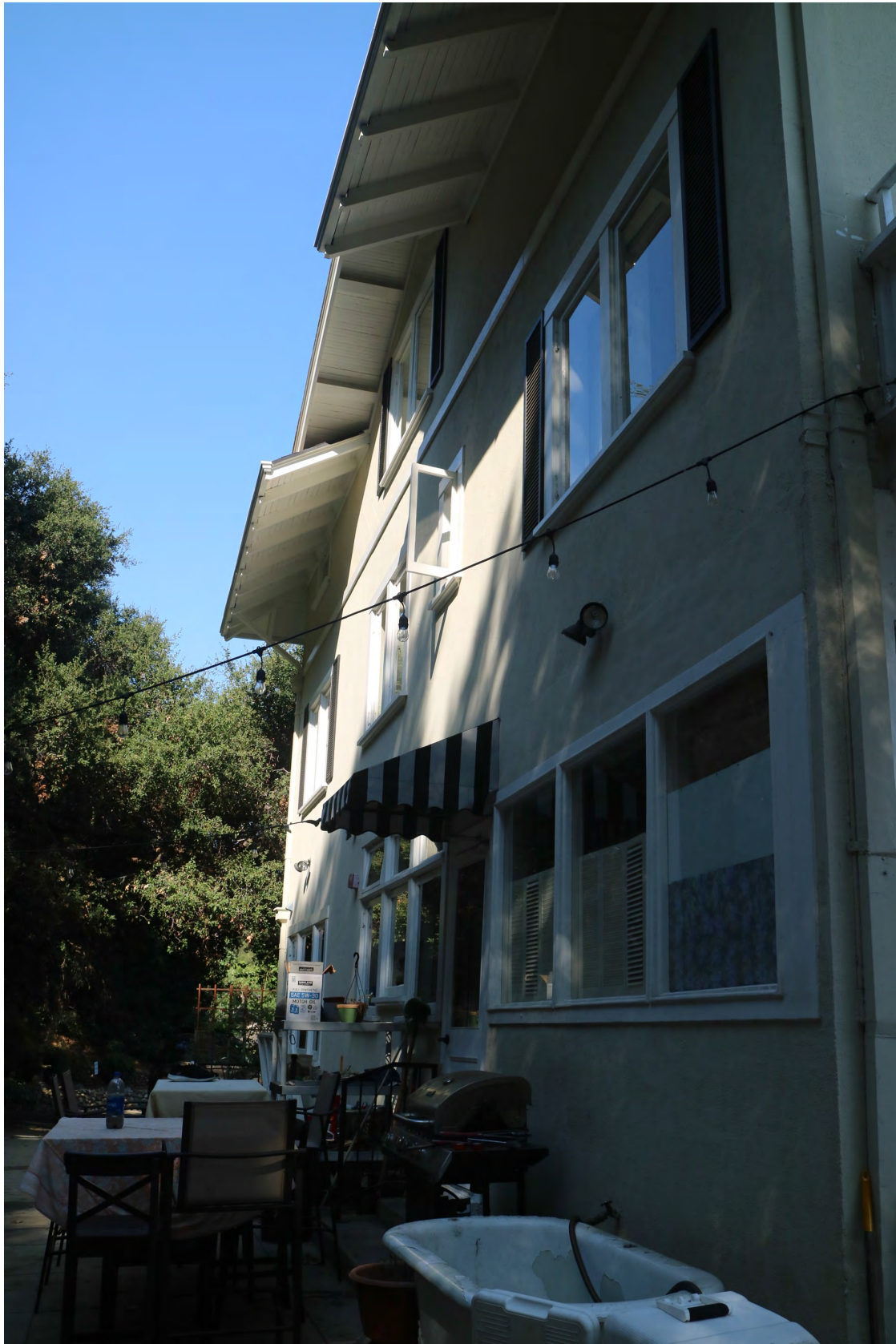
Figure 8 South elevation, overview, 335 Monterey Road (southeast perspective)
