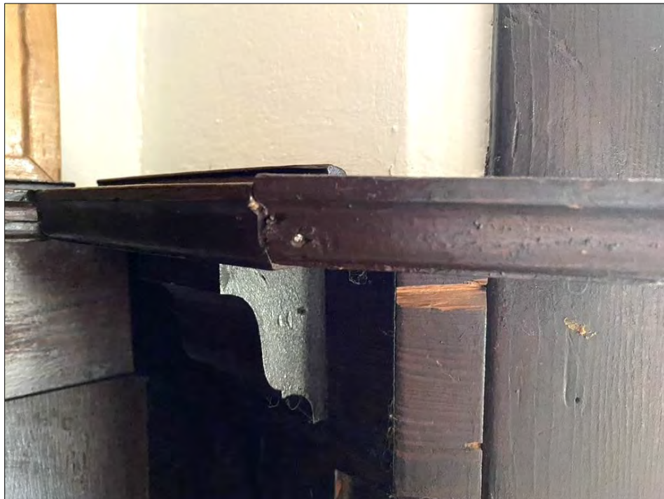
Broken pieces of wall galley shelves in the dining room to be restored.
