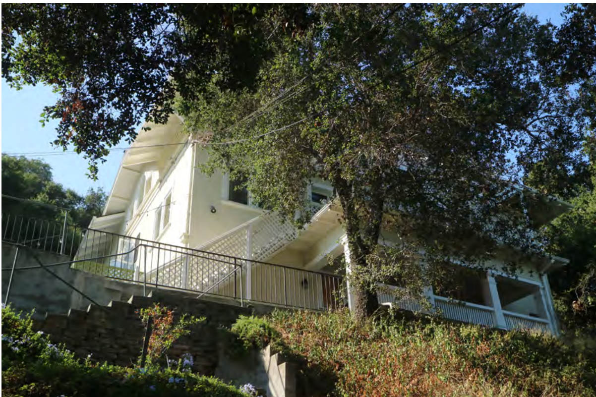
Figure 15 North elevation overview, 335 Monterey Road (northeast perspective)
