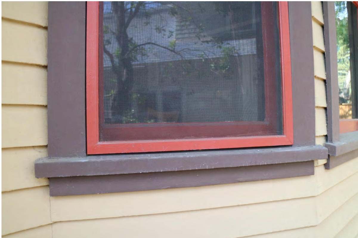
Figure 12 Detail of wood-framed screen
