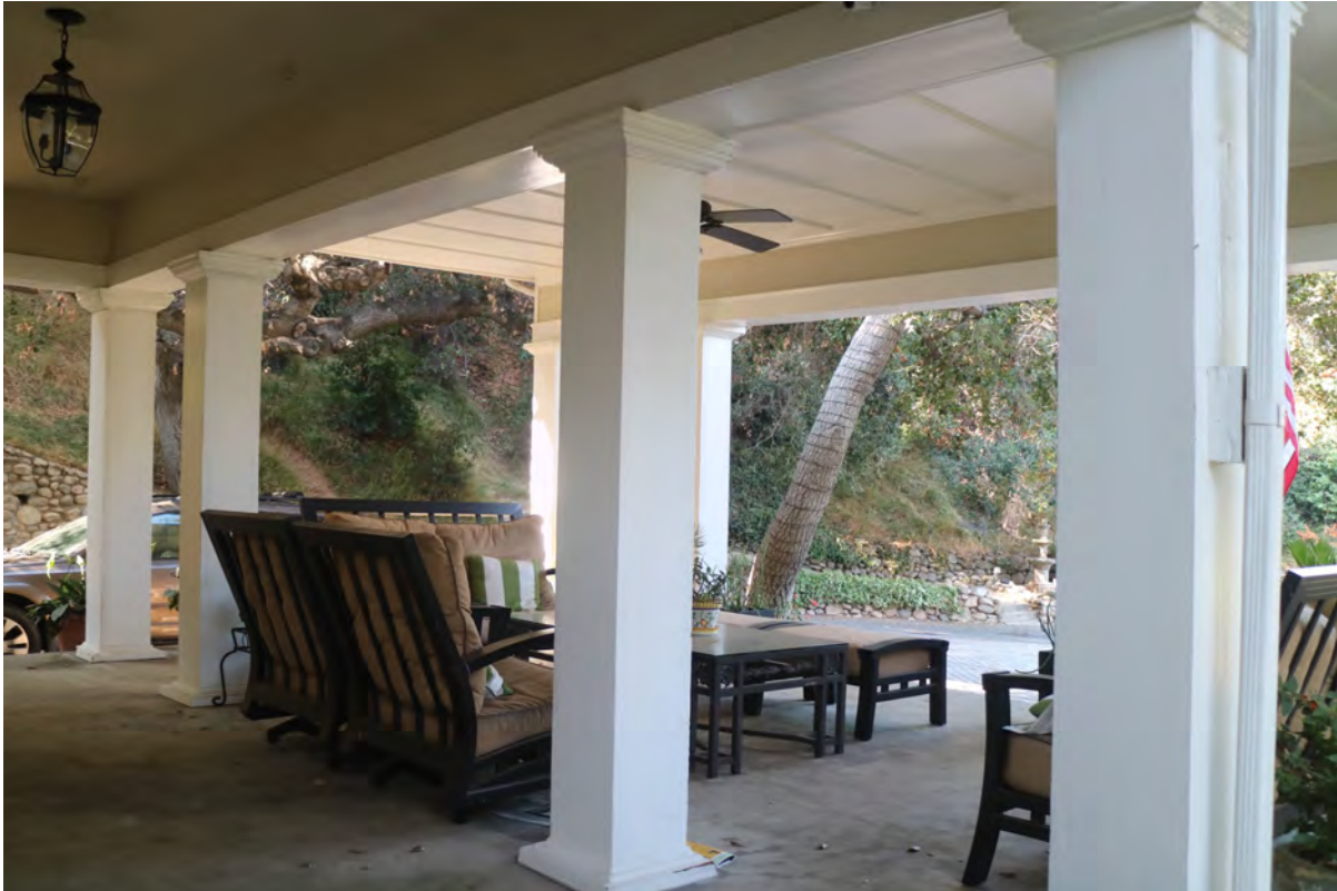
Figure 3 Detail of entrance porch (northeast perspective)
