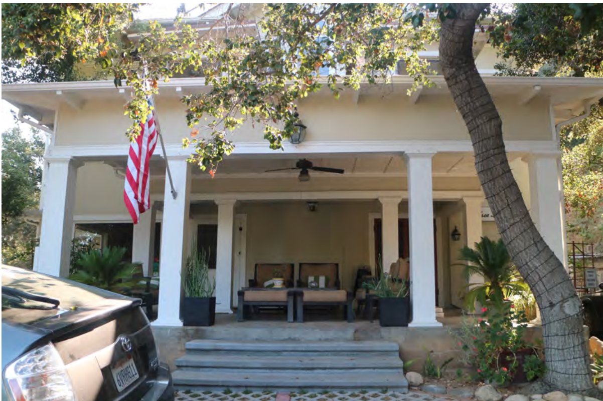
Figure 2 Primary elevation, detail, 335 Monterey Road (west perspective)
