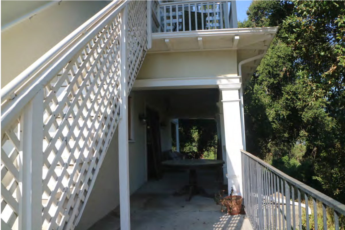
Figure 16 North elevation detail, 335 Monterey Road (east perspective)
