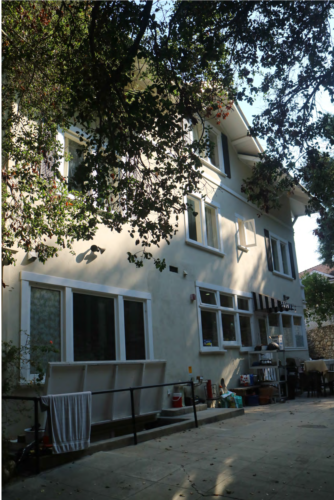
Figure 7 South elevation, overview, 335 Monterey Road (southwest perspective)
