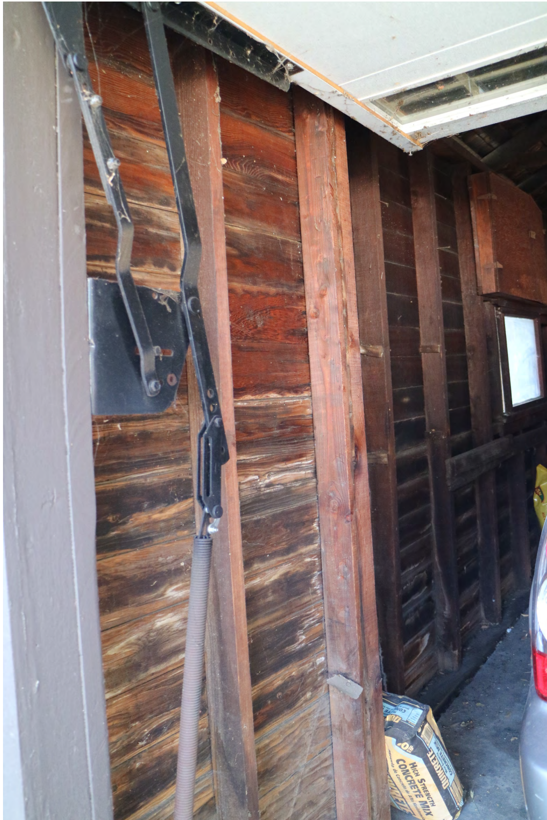
Figure 7 Garage interior, detail, 704 Meridian Avenue
