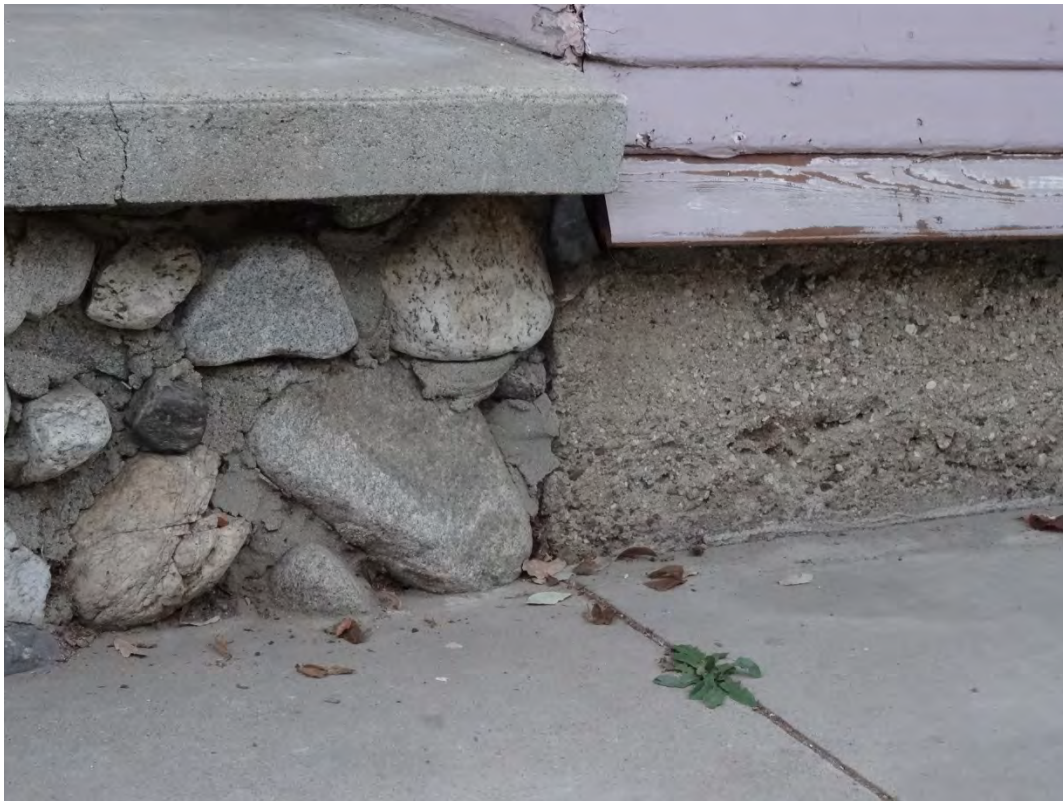
Stone and concrete foundation
