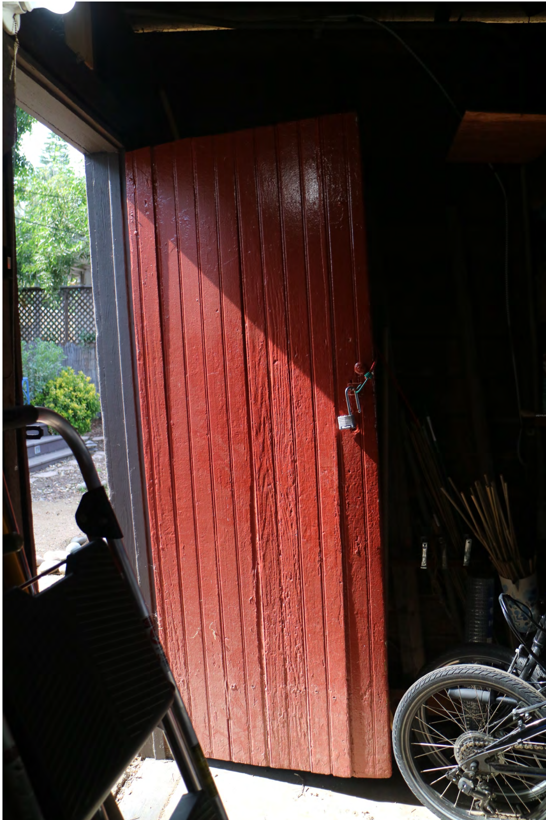
Figure 8 Garage interior, detail, 704 Meridian Avenue
