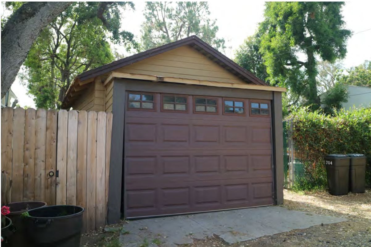
Figure 6 Rear elevation, garage, 704 Meridian Avenue (southeast perspective)
