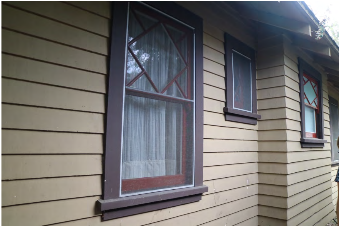
Figure 13 Detail of aluminum-framed screen, north elevation
