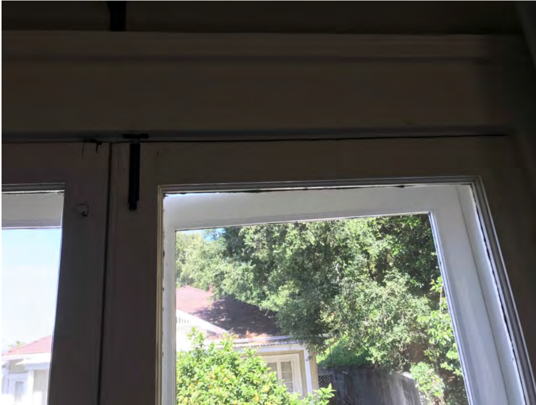
Figure 25 Interior, detail of wood-frame window and hardware
