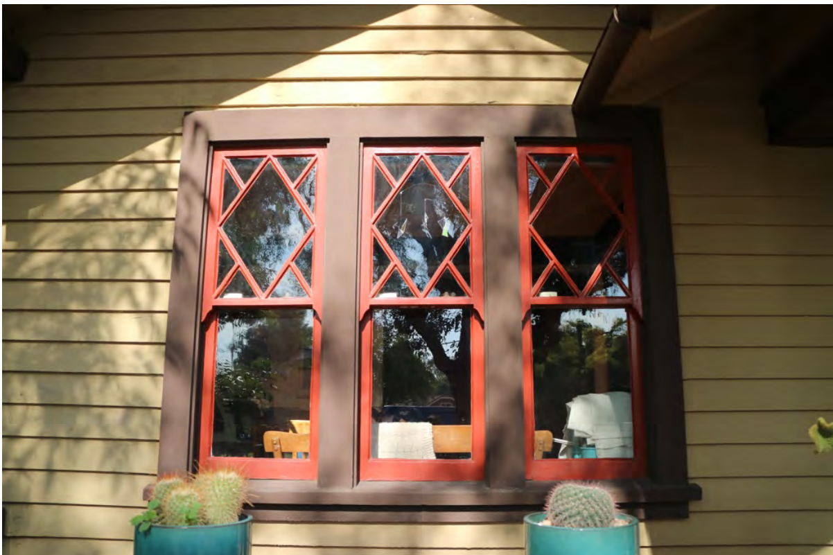
Figure 10 Overview of original, wood-frame windows
