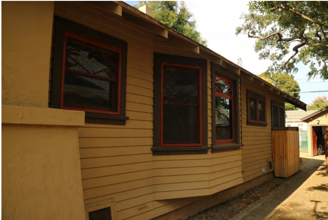
Figure 11 Overview of original, wood-frame windows
