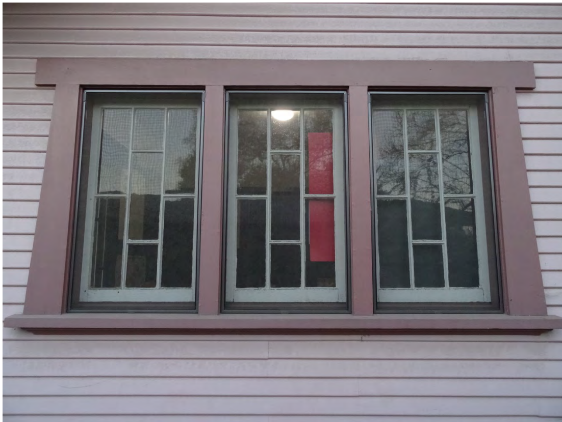
Original wood windows (to be repaired as needed)
