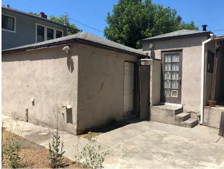
Figure 8. Southern Façade, 23 Short Way SOURCE: Sapphos Environmental, Inc., 2020
