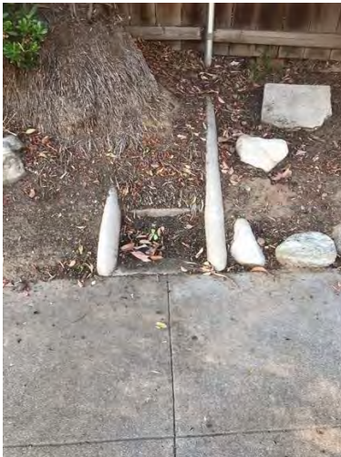
Original rear entry steps
