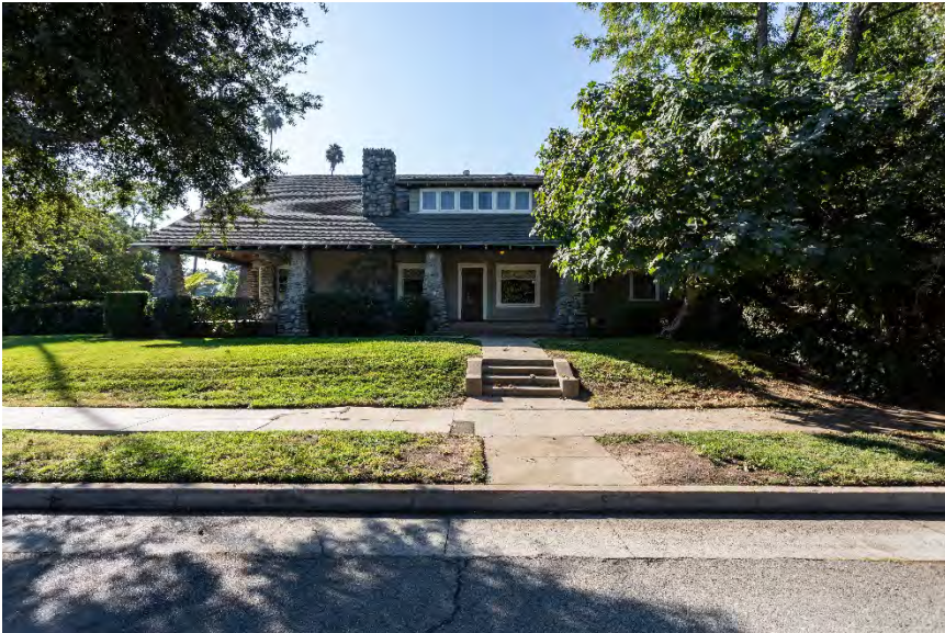
North façade, view facing south.
