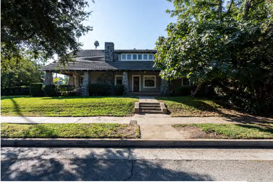
North façade, view facing south.
