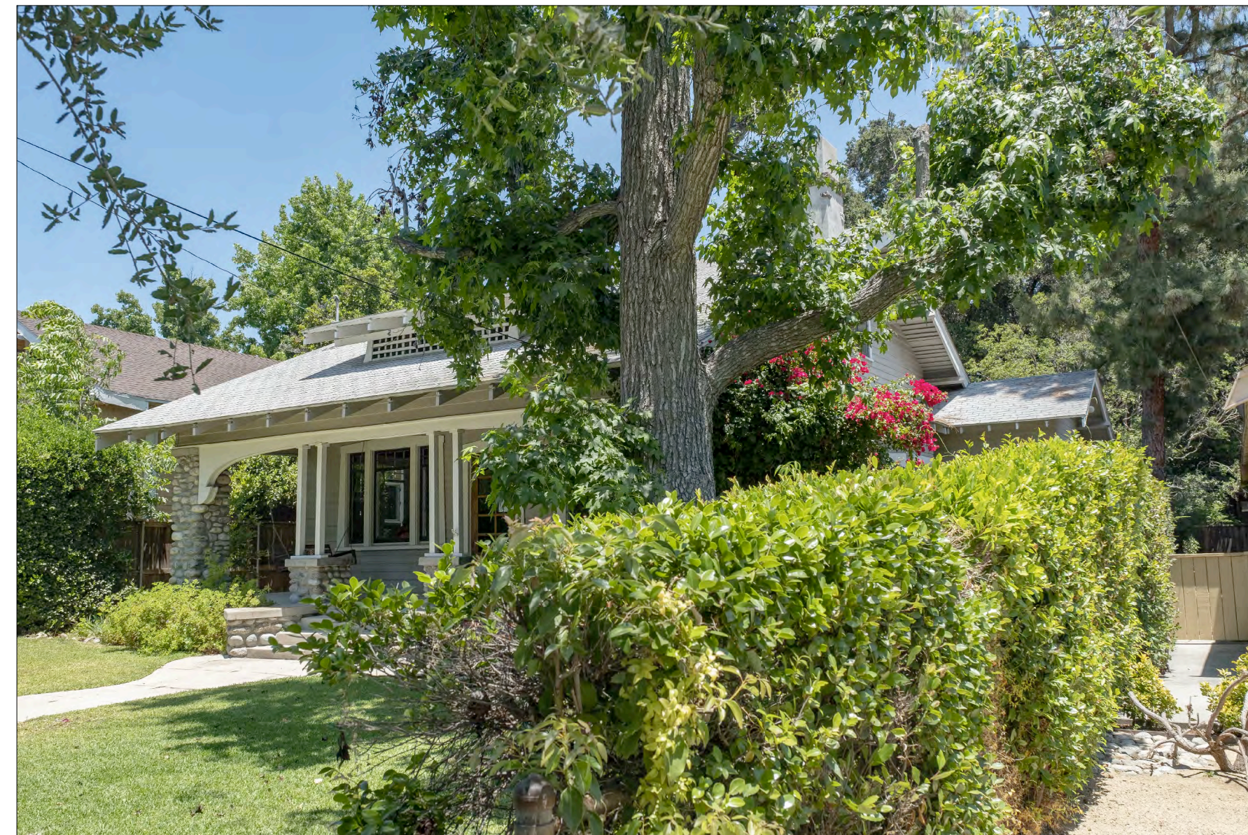
EXISTING FRONT / WEST ELEVATION - FROM SOUTH
