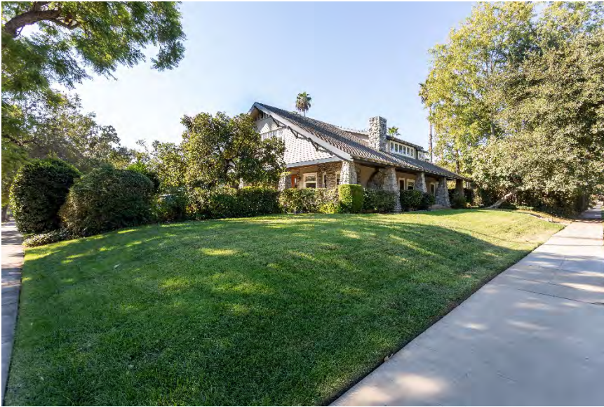
North and east façades, view facing southwest.
