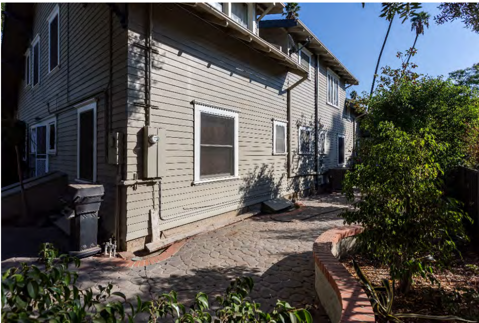
South and west façades, view facing northeast.
