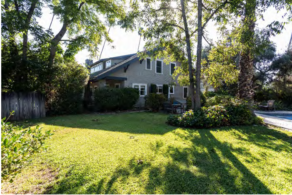
West and north façades, view facing southeast.
