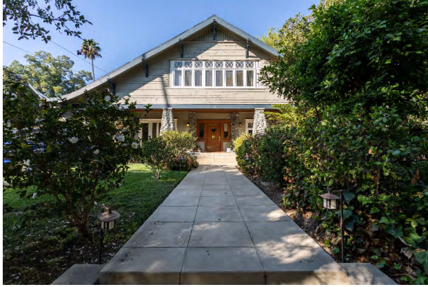
East façade, view facing west.
