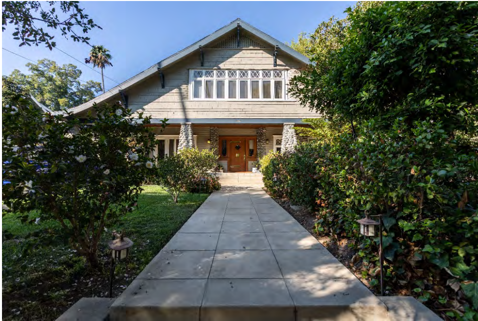
East façade, view facing west.
