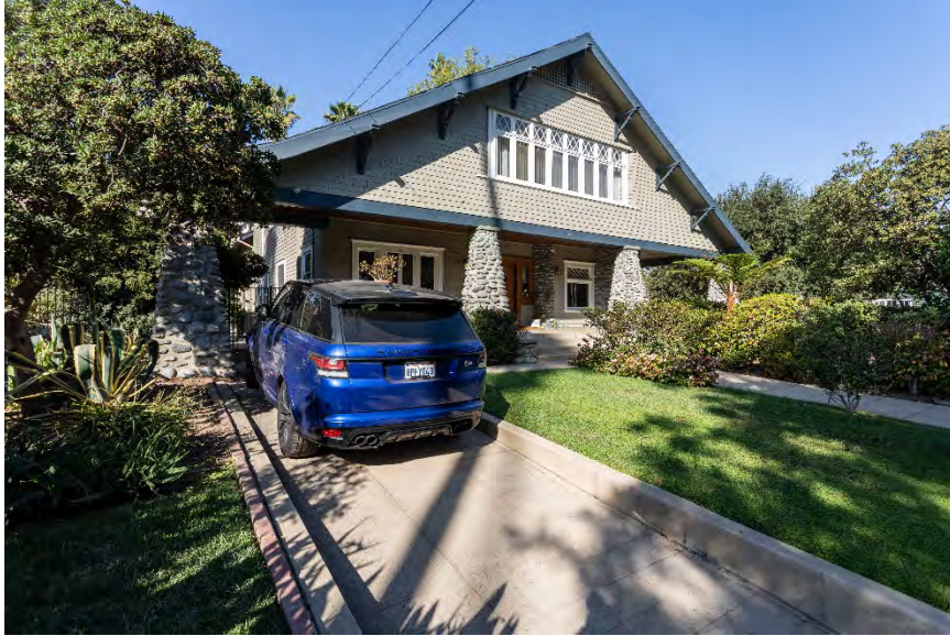
East and south façades, view facing northwest.
