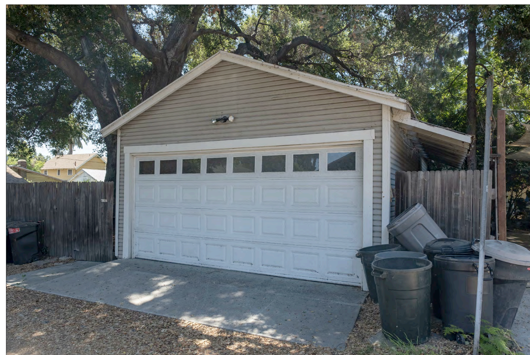
EXISTING GARAGE EAST ELEVATION
