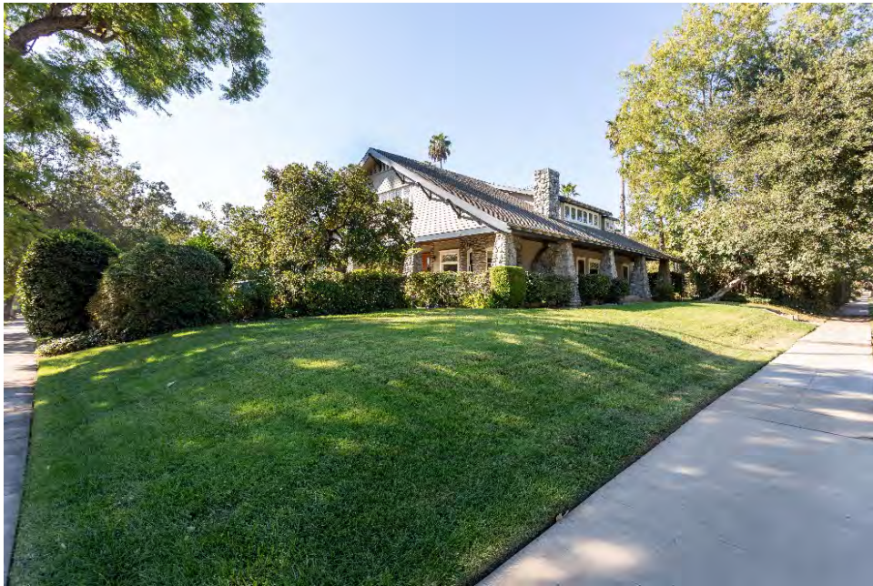
North and east façades, view facing southwest.
