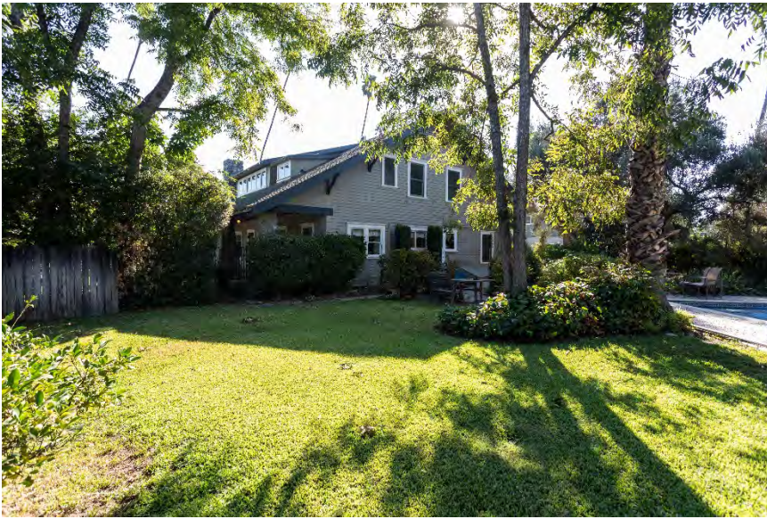
West and north façades, view facing southeast.
