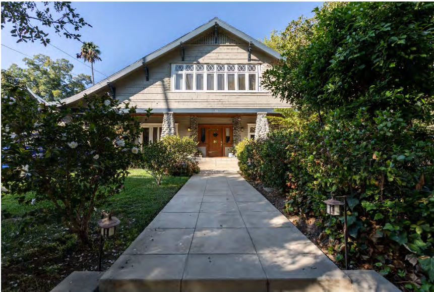
East façade, view facing west.
