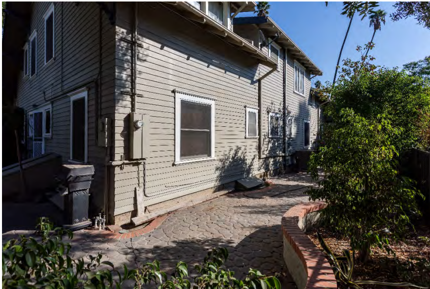
South and west façades, view facing northeast.
