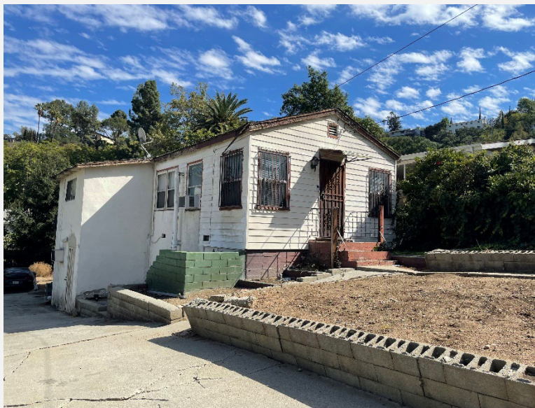
Exhibit 1. Primary (west) and north elevations, view looking east.
