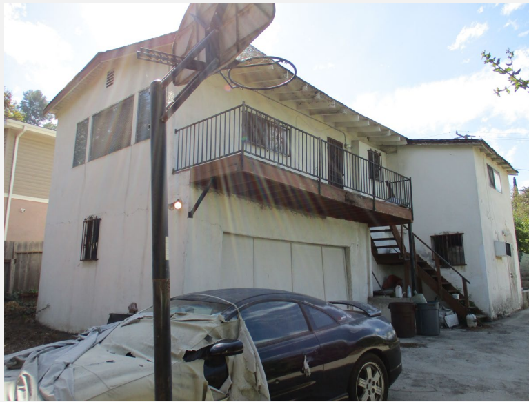
Exhibit 2. North and rear (east) elevations, view looking southwest.
