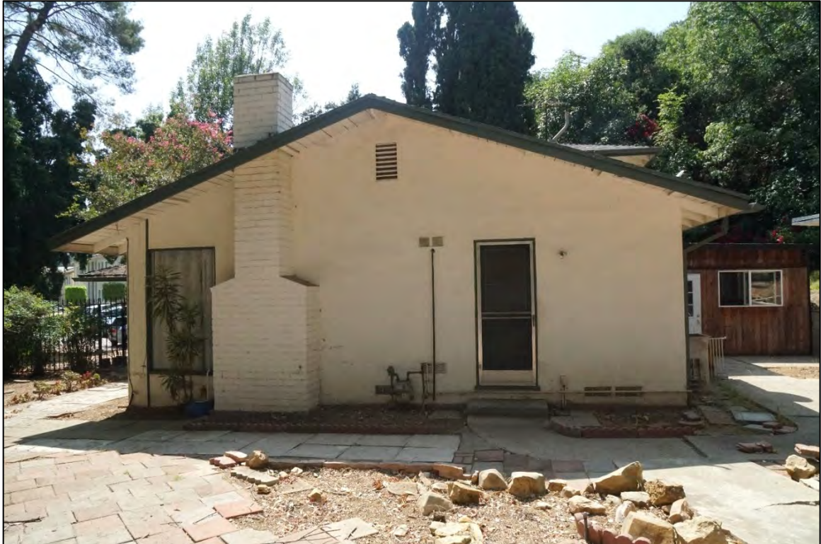
Figure 7. East elevation of home, view facing west.
