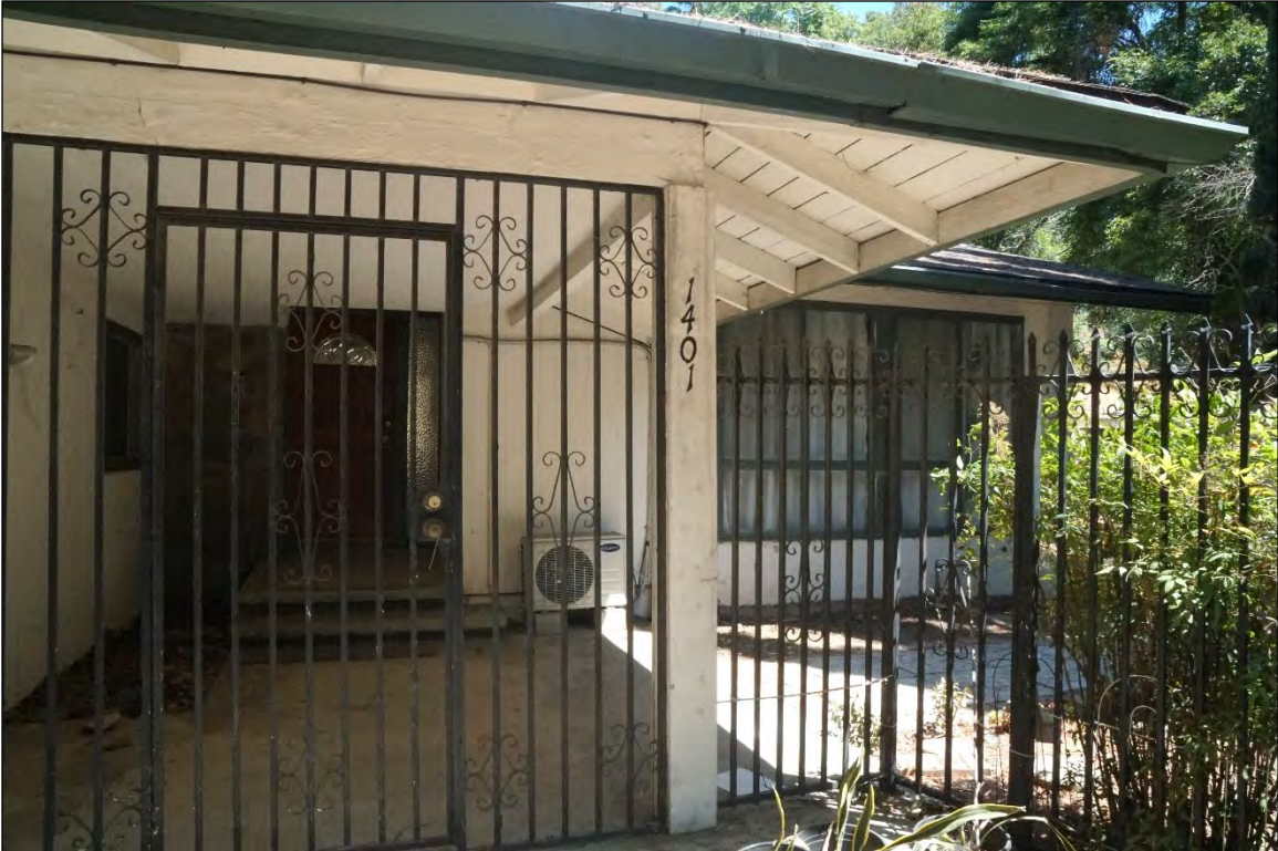
Figure 6. Closeup of primary entrance and east wing; view facing north.
