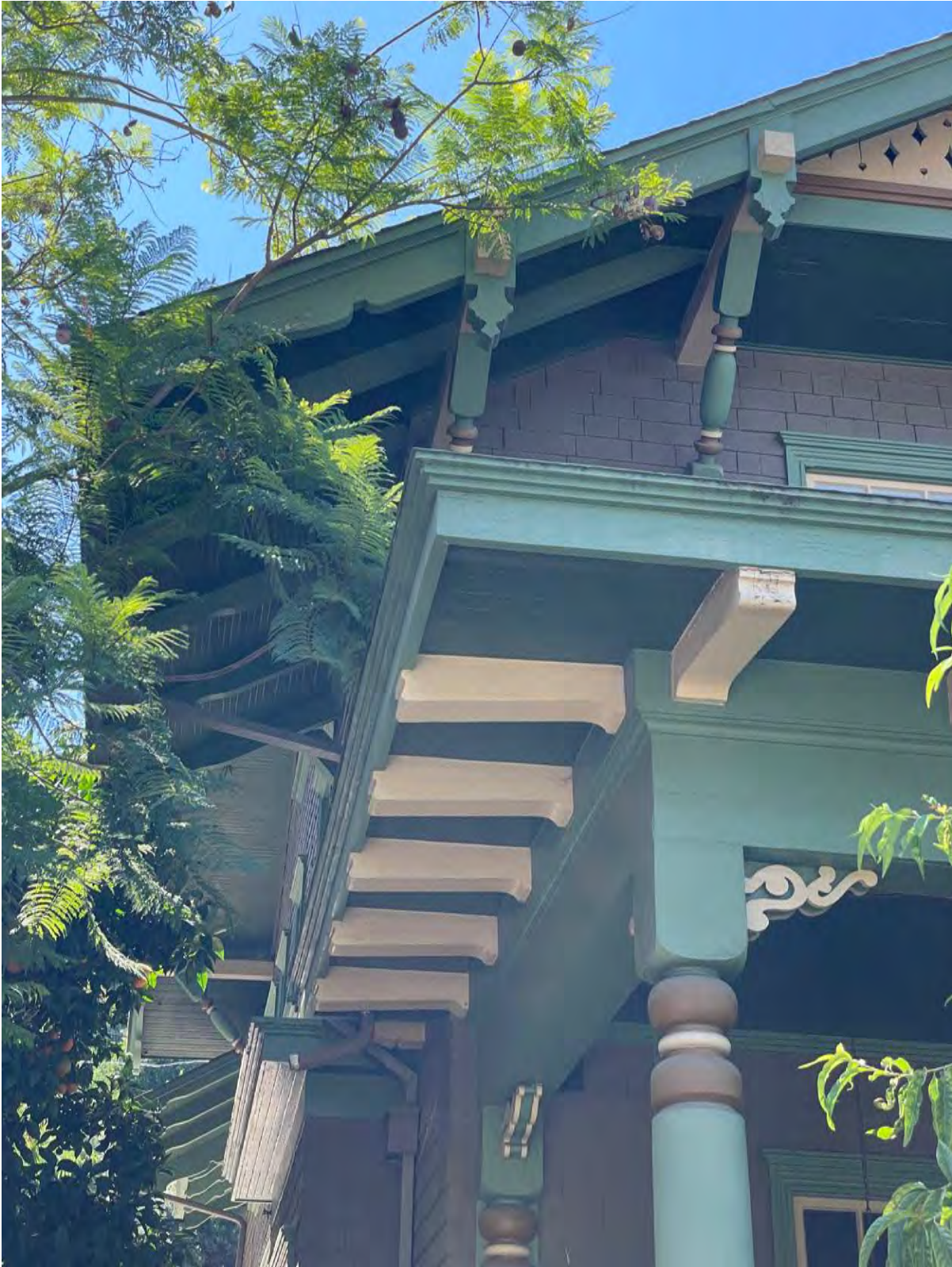
Figure 5 Roof eave treatment and details, façade and south elevation, east perspective
