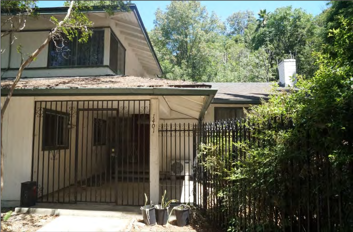
Figure 5. Closeup of the south façade at the juncture of the two-story and one-story wings, view facing north (the east wing is partially obscured by foliage).
