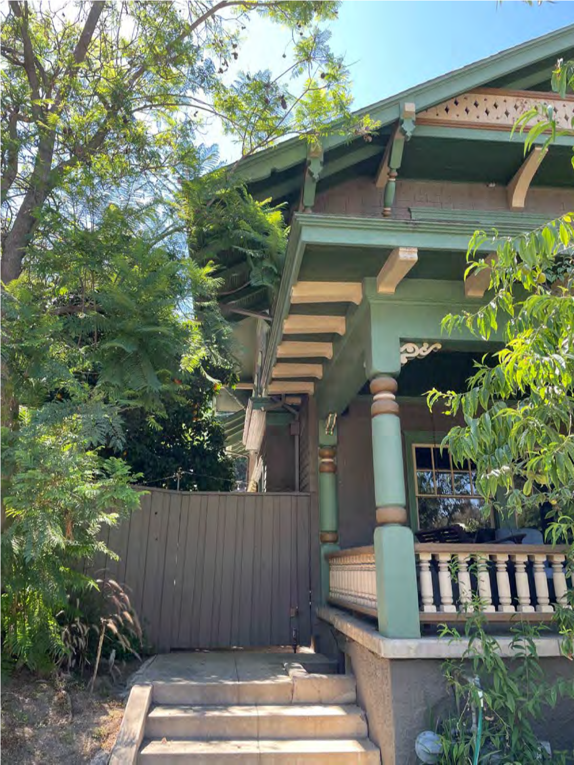
Figure 4 Detail, façade and south elevation, 1209 Indiana Avenue, east perspective
