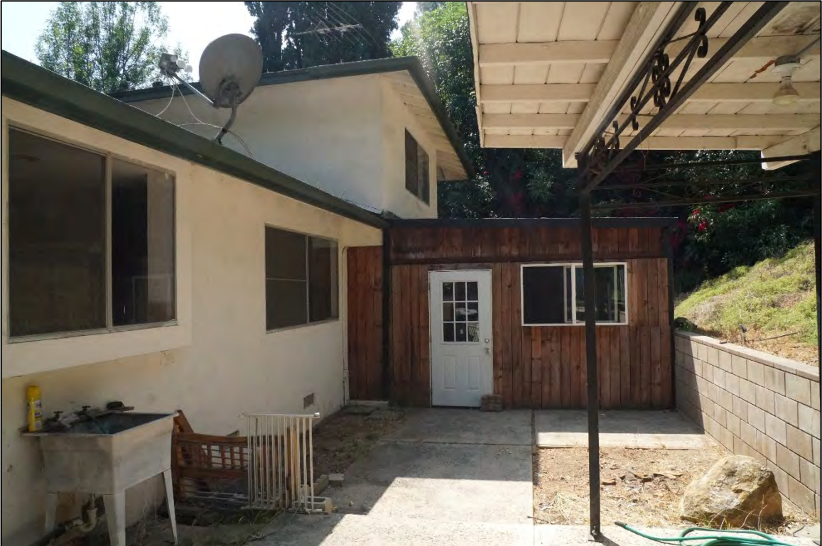
Figure 9. Closeup of the home’s rear elevation and addition, view facing southwest.
