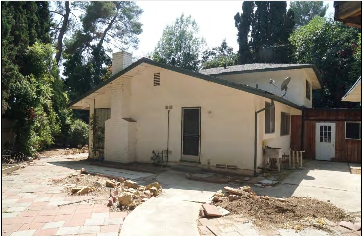
Figure 8. Overview of rear of home showing addition, view facing southwest.
