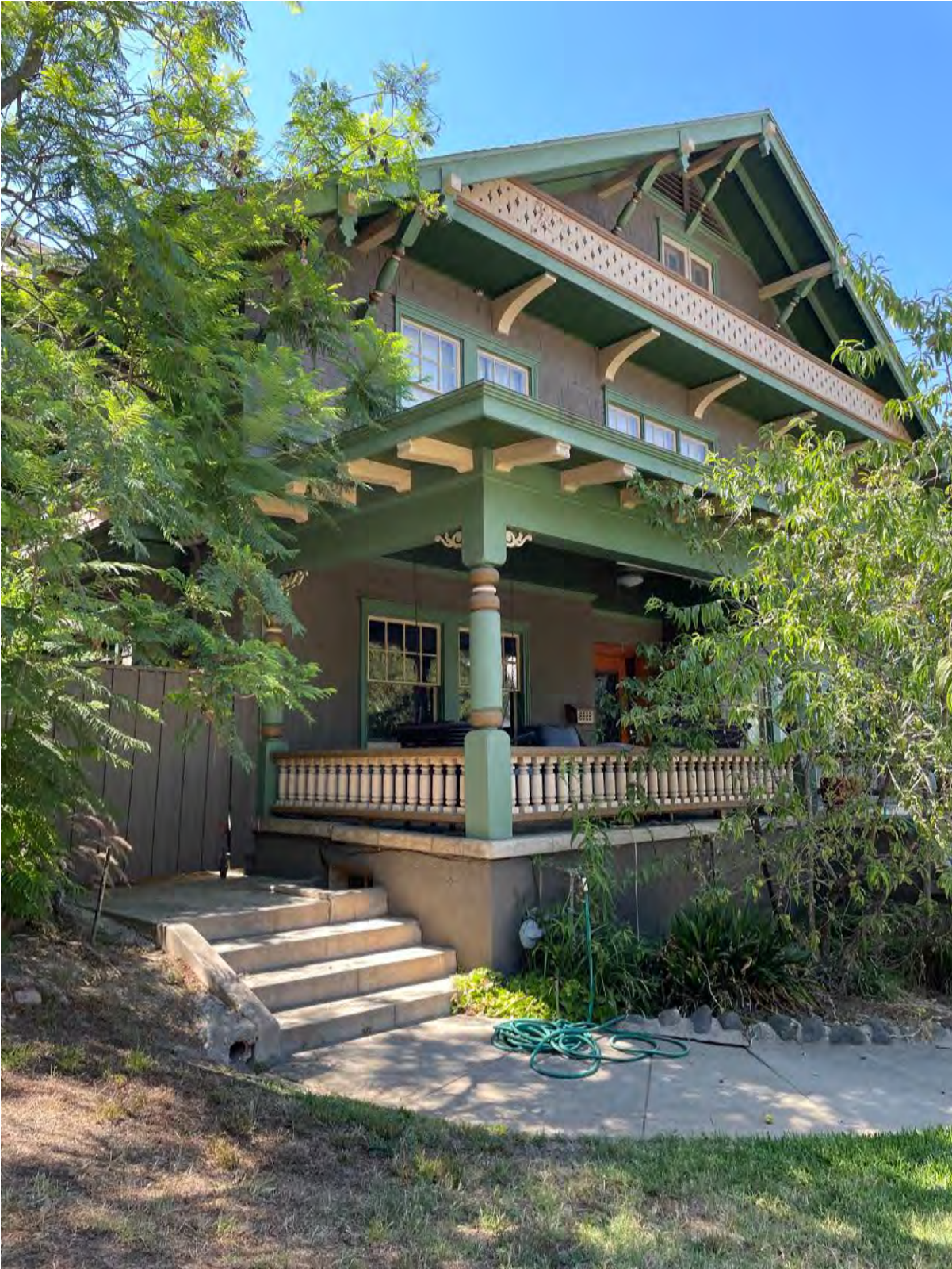
Figure 3 Detail, façade, 1209 Indiana Avenue, southeast perspective
