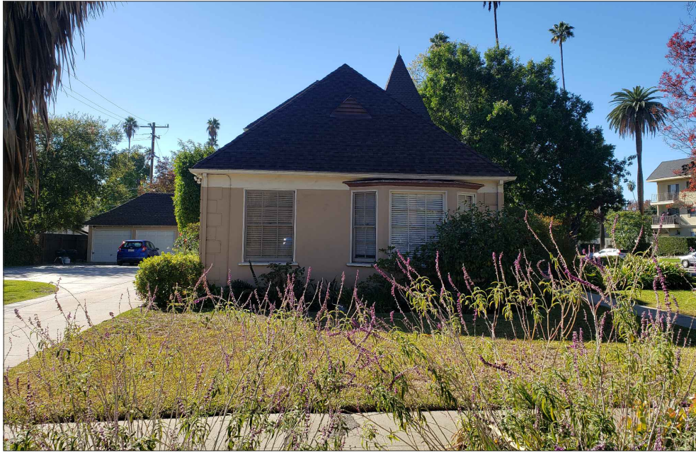
05 - 1600 FREMONT AVE, SOUTH PASADENA, CA 91030
