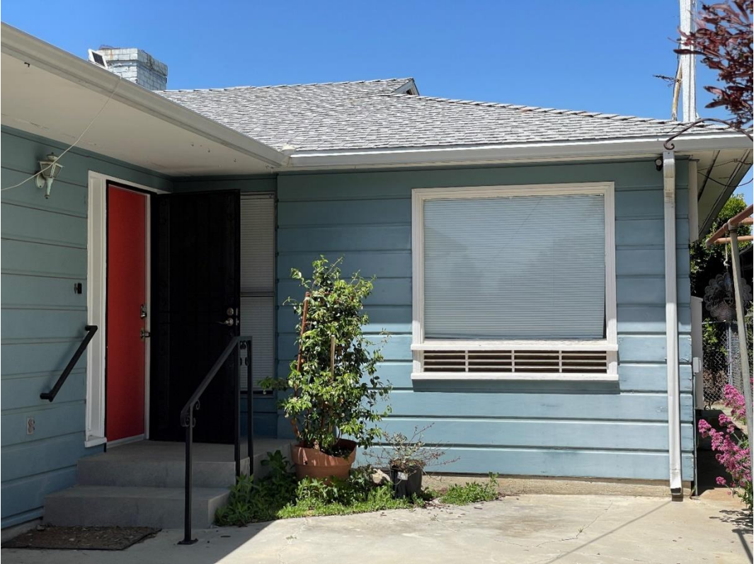
Figure 4. Detail of entry patio, door, fenestration, and roof-line treatment, east/southeast elevation
