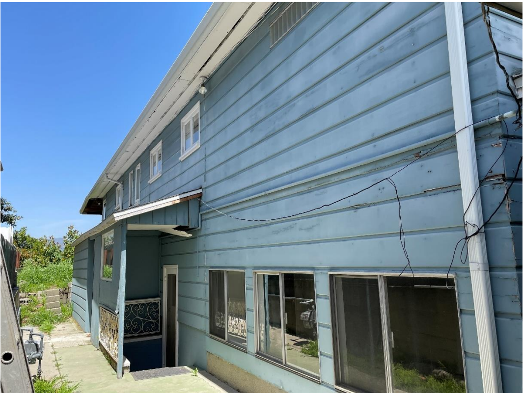
Figure 5. West elevation, showing two-story mass and partial basement-level ground story in the northern portion of the house
