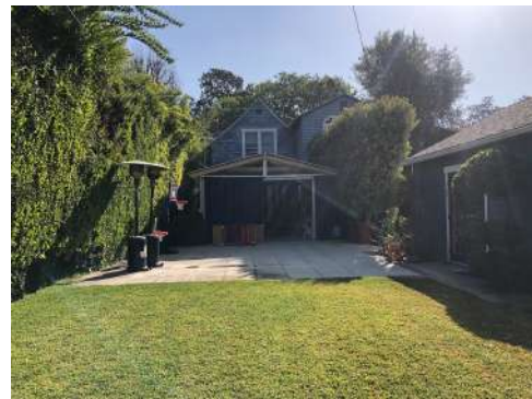
G - (E) REAR ELEVATION & YARD
