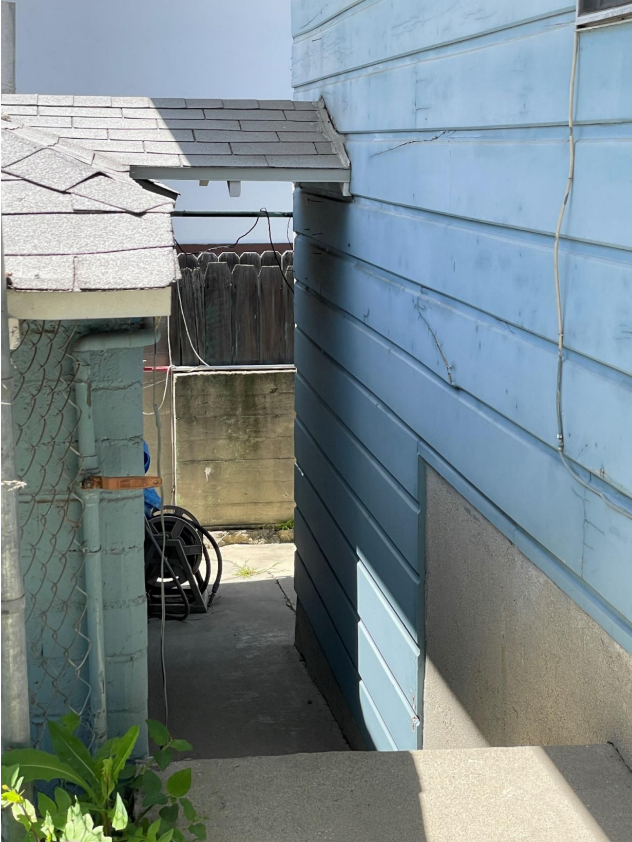
Figure 8. Connection point, small roof extension between garage and house, west elevation
