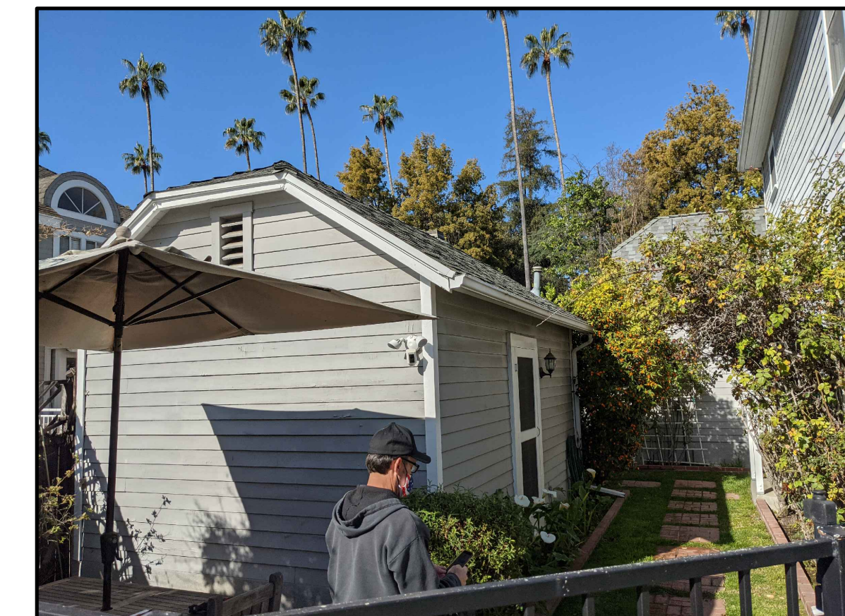
1806 WAYNE AVENUE GARAGE LOOKING WEST
