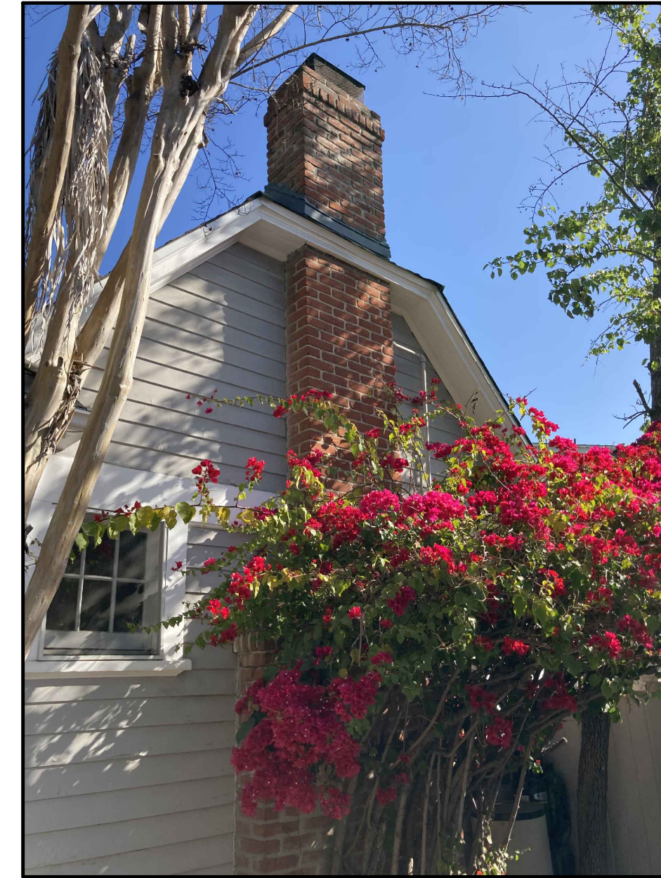
1806 WAYNE AVENUE WHERE ADDITION OCCURS LOOKING NORTH EAST
