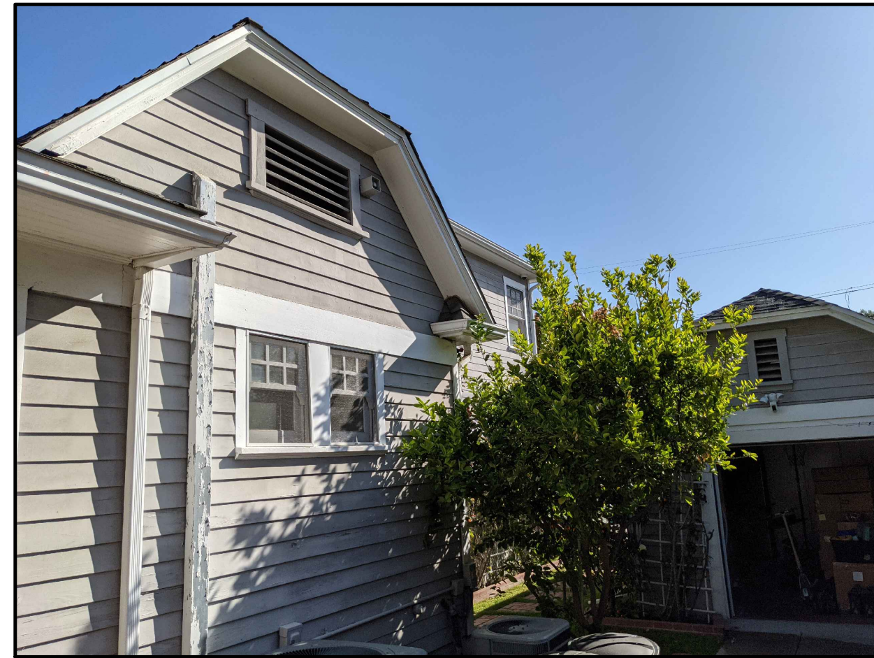
1806 WAYNE AVENUE WHERE ADDITION OCCURS LOOKING NORTH EAST
