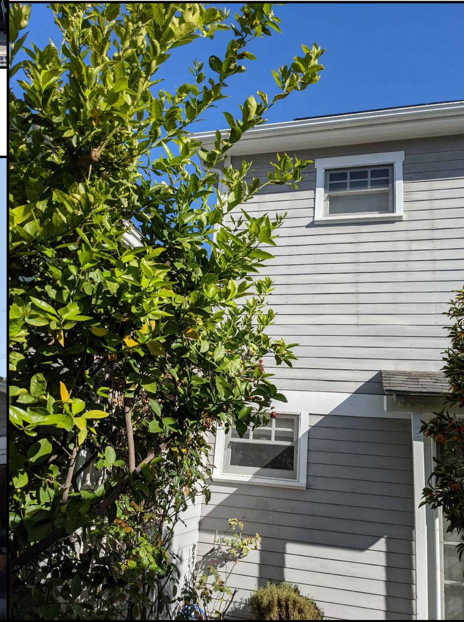
1806 WAYNE AVENUE WHERE ADDITION OCCURS LOOKING NORTH WEST
