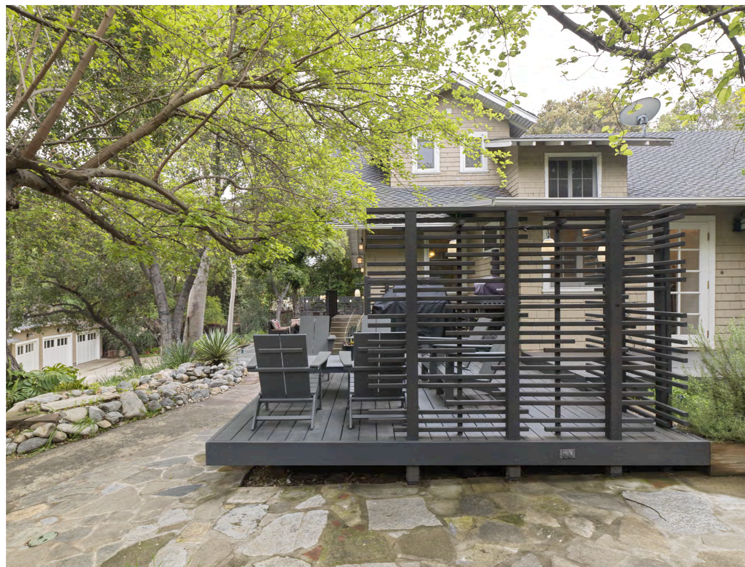
NORTH DETAIL VIEW
