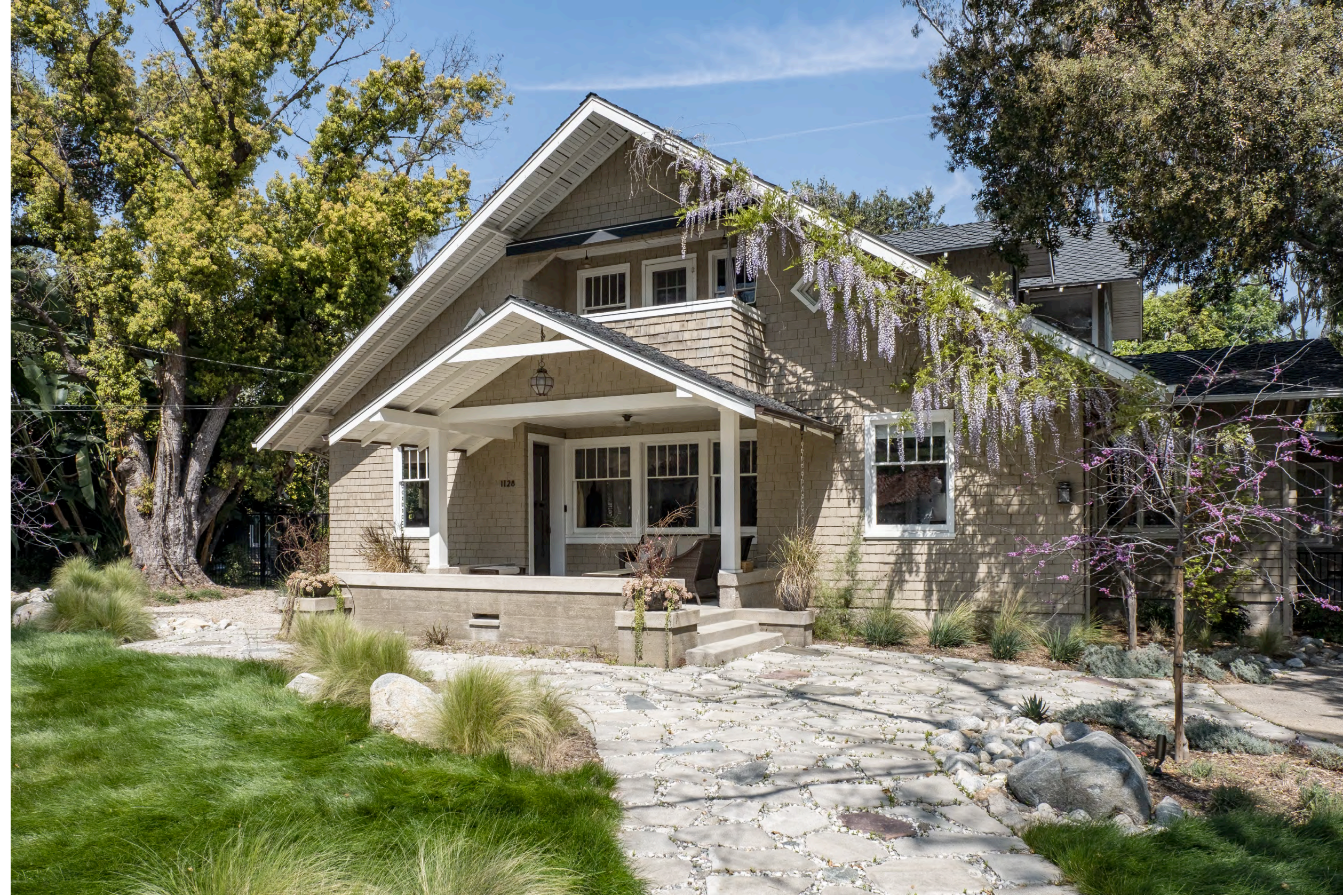
SOUTHWEST DETAIL VIEW
