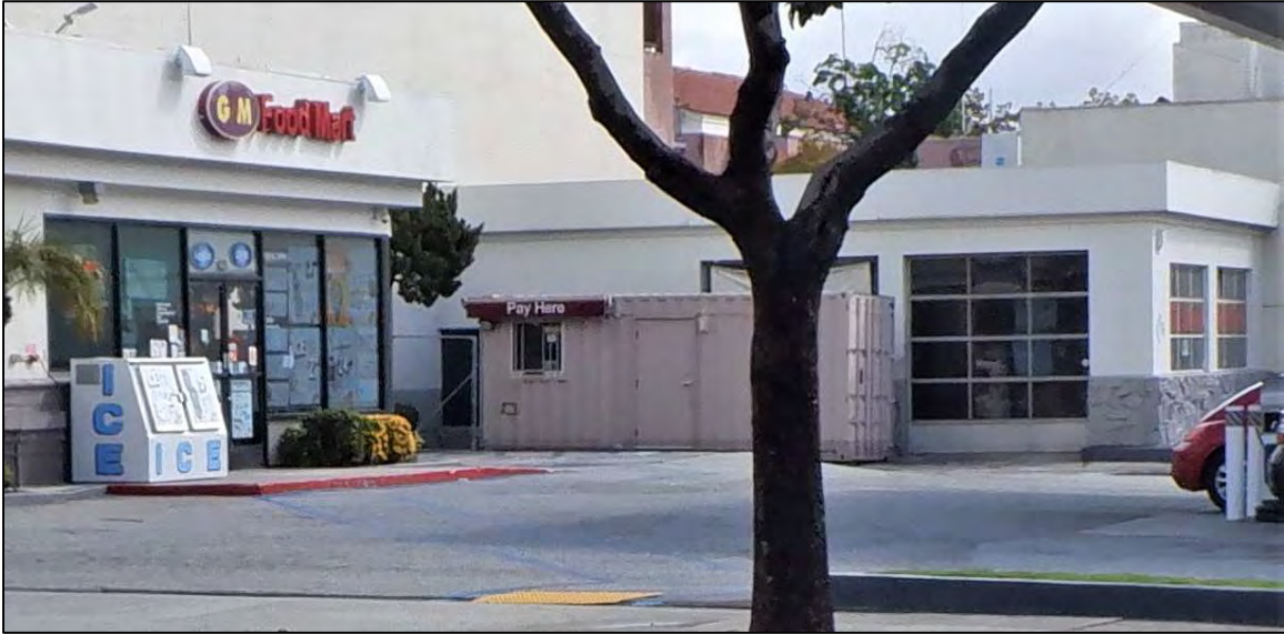
Photograph 3: Portable shipping container retrofitted for cashier services. Camera facing northeast, March 23, 2023.
