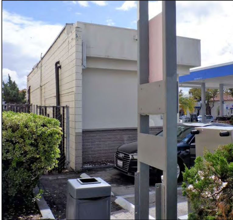
Photograph 7: Rear, north side and west end of the convenience store at 1400 Mission Street. Camera facing southeast, March 23, 2023.
