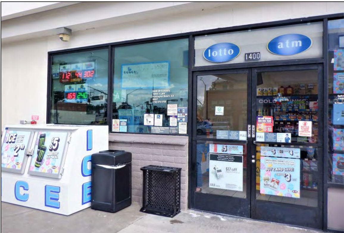
Photograph 6: Detail view of the entrance on the south façade of the convenience store at 1400 Mission Street. Camera facing northwest, March 23, 2023.
