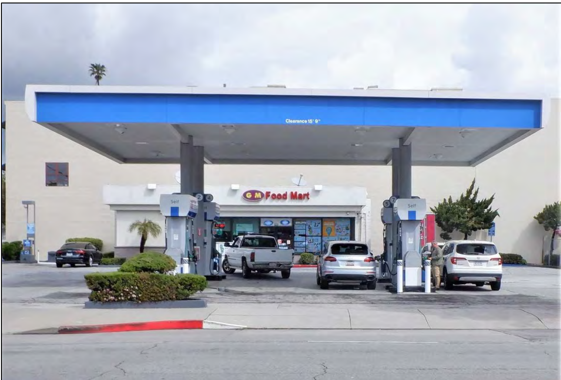
Photograph 2: Modern canopy mounted over the fuel pump stations at 1400 Mission Street. Camera facing north, March 23, 2023.
