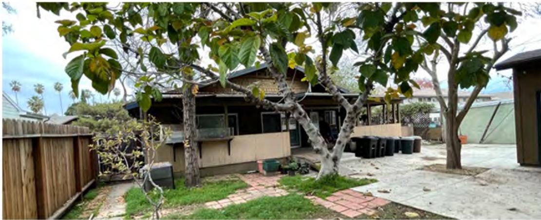
Rear elevation looking from rear of the property
