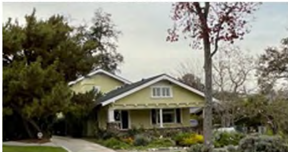
1510 Rollin st. neighboring property
