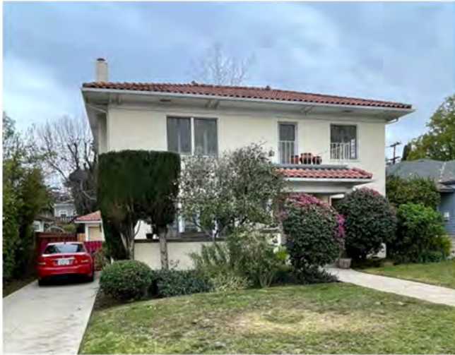
1429 Rollin st. neighboring property
