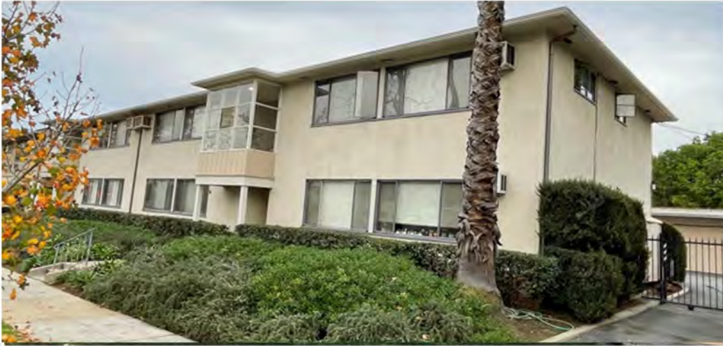
apartment complex Rollin st. & Fair oaks neighboring property (to the left)
