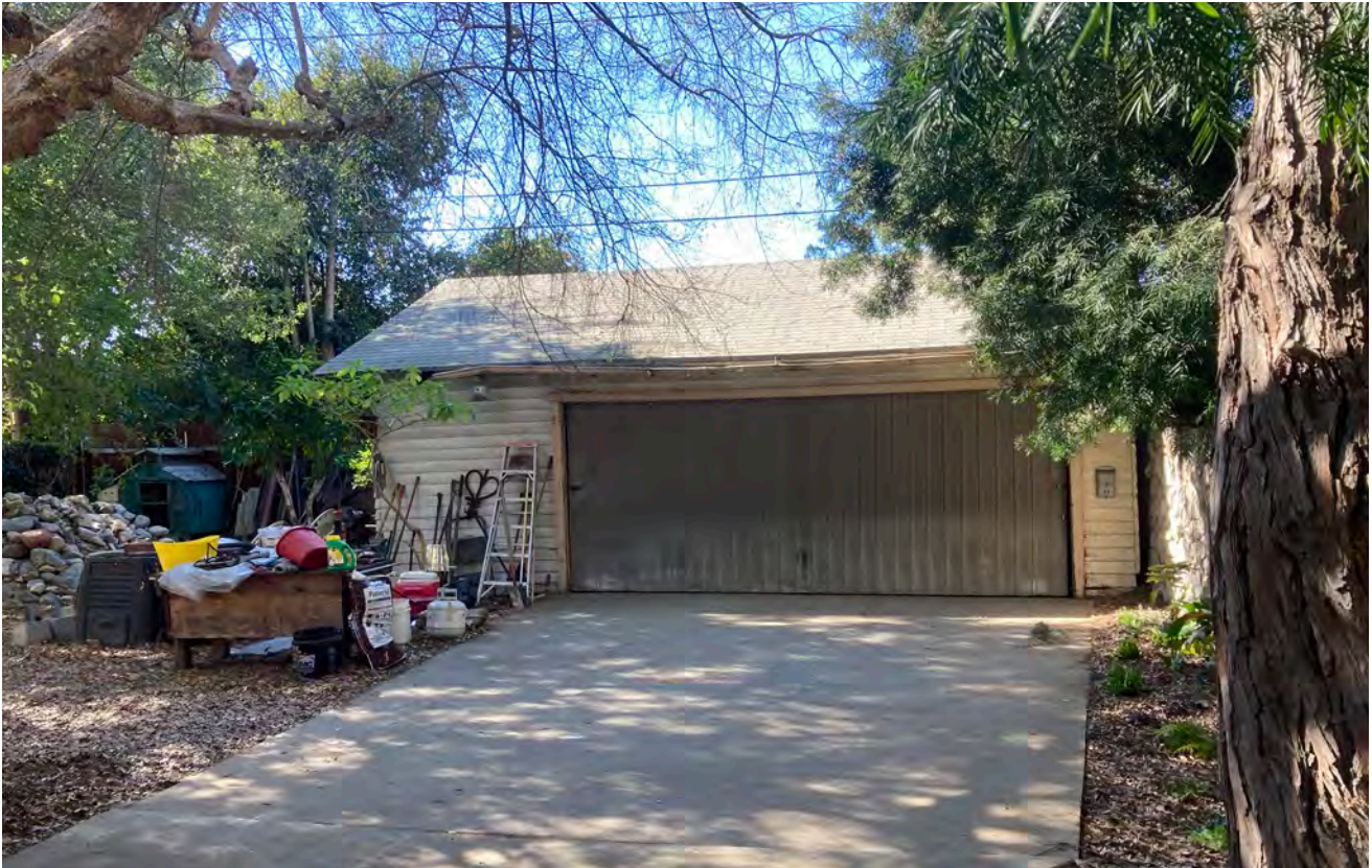
View of Front of (E) garage
