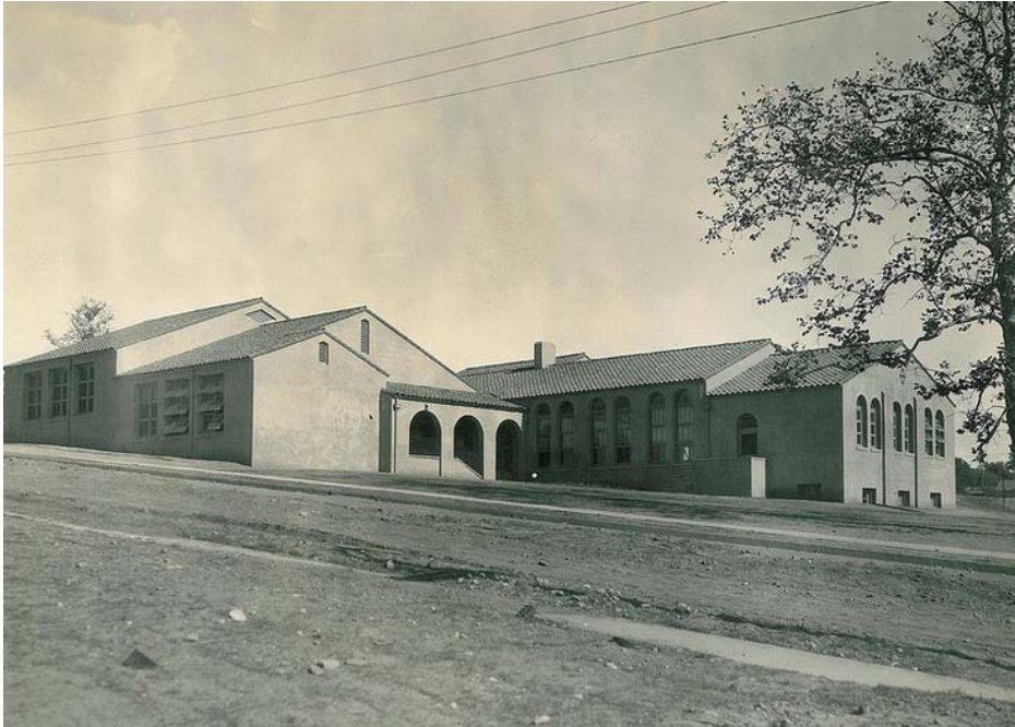
Figure 71. Las Flores Elementary School, 1924 (demolished). Source: South Pasadena Public Library.
