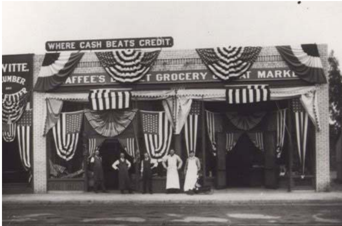
Figure 63. Chaffee's Basket Grocery, 1910 (demolished). Source: South Pasadena Public Library.
