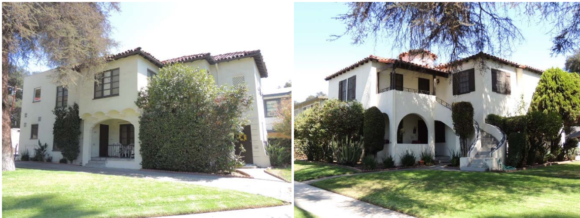
Figure 75. Spanish Colonial Revival multi-family residences. R: 315 Pasadena Avenue. R: 317 Pasadena Avenue. Photographs 2014; source: Historic Resources Group.
