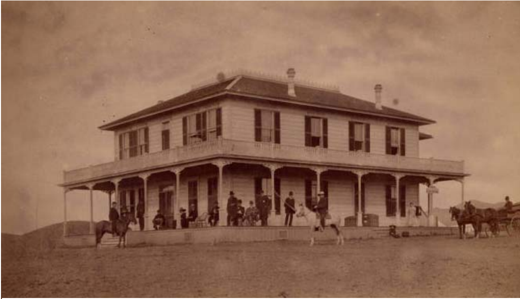
Figure 15. Hermosa Vista Hotel, Columbia and Orange Grove, 1883 (demolished). Source: Pasadena Digital History Collaboration.
