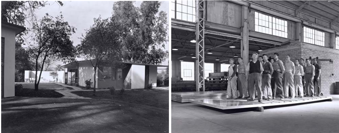
Figure 103. L: Exterior of Vultee prefabricated house at 325 Monterey Road, South Pasadena Landmark #51. R: Consolidated Vultee Aircraft factory workers standing on a panel for the prefabricated “Vultee” or “Fleet” House marketed through Southern California Homes Inc. in 1949. Source: Julius Shulman, Getty Research Institute, Digital Collection.
