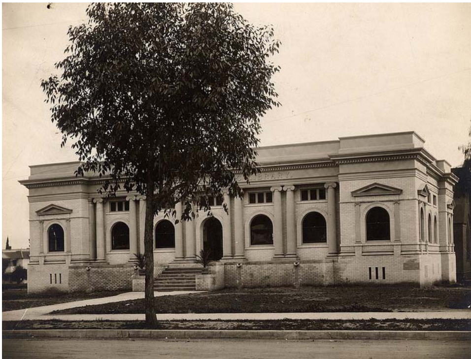
Figure 68. Carnegie Library, as originally designed in 1908. Photograph 1910; source: South Pasadena Public Library.
