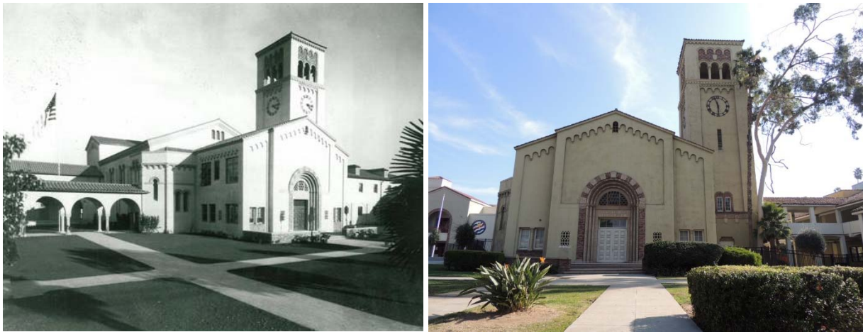
Figure 86. L: South Pasadena Middle School Auditorium, designed by Marsh, Smith & Powell, 1928. Photograph c. 1960; source: South Pasadena Public Library. R: The building in 2014. Source: Historic Resources Group.
