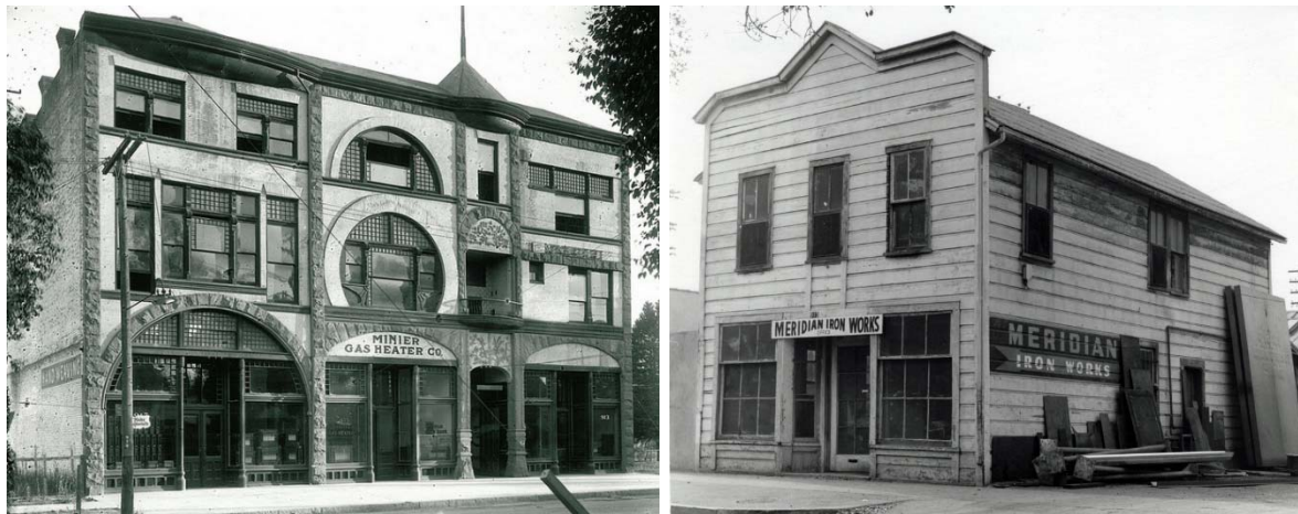
Figure 28. L: Mohr-Graham Building, originally constructed in 1888 (demolished). Photograph 1910; source: South Pasadena Public Library. R: Meridian Iron Works, originally constructed in 1887. Photograph c. 1950; source: South Pasadena Public Library. The Meridian Iron Works has been relocated to 913 Meridian Avenue; it is South Pasadena Landmark #5.
