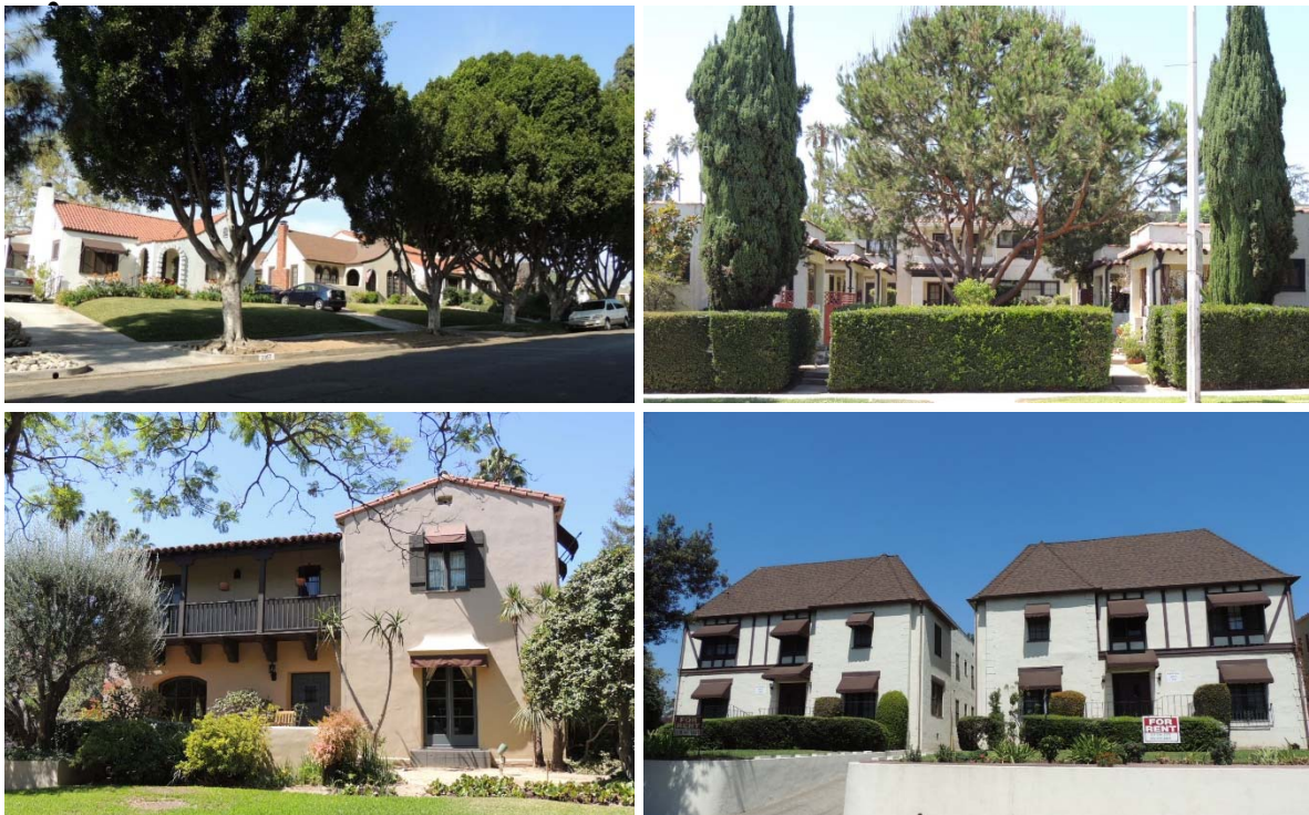
Figure 80. TL: Collection of 1920s residences along Primrose Avenue. TR: Bungalow court at 1825 Fremont Avenue. BL: 1719 Marengo Avenue. BR: “Marengo Apartments,” 1612-1616 Huntington Drive. Photographs 2014; source: Historic Resources Group.
