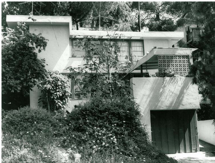
816 Bonita Drive, Grokowsky House. Photograph c. 1980; source: South Pasadena Public Library. (South Pasadena Landmark #28)
