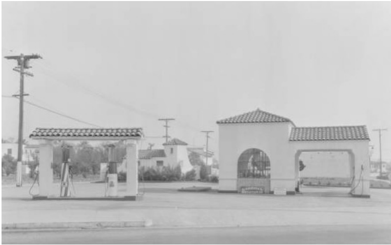
Figure 83. Gas Station at Mission and Los Robles, 1930. Source: Huntington Digital Library.
