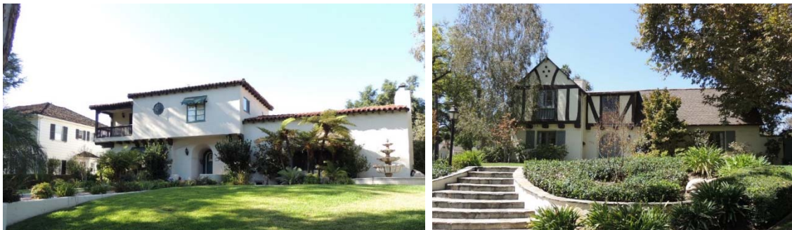
Figure 76. L: Spanish Colonial Revival single-family residence at 928 Buena Vista, 1927. Tudor Revival single-family residence at 1623 Marengo, 1927. Located in the Oneonta Park tract. Photographs 2014; source: Historic Resources Group.
