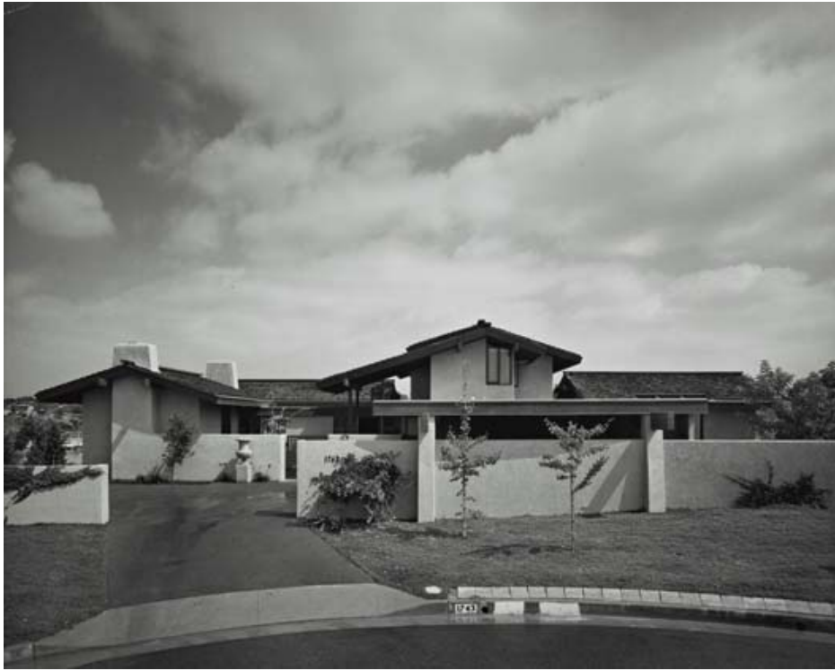
Figure 124. Melbye Residence, Tyron and Driskel, 1967, 1743 Camino Lindo. Source: Julius Shulman, Getty Research Institute, Digital Collection.
