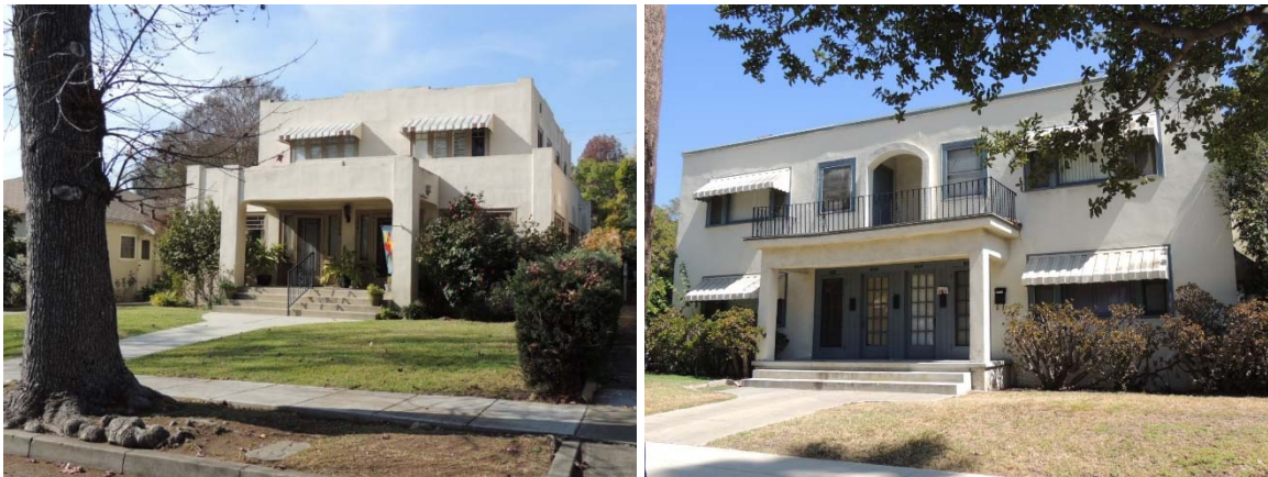
Figure 79. L: 1741 La Senda Place, one of a small grouping of duplexes from this period. R: 331 Pasadena Avenue, part of a group of multi-family residential properties along Pasadena Avenue. Photographs 2014; source: Historic Resources Group.
