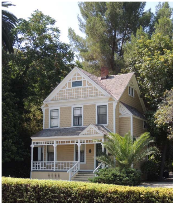
309 Monterey Road, Vivekananda House (South Pasadena Landmark #29)
