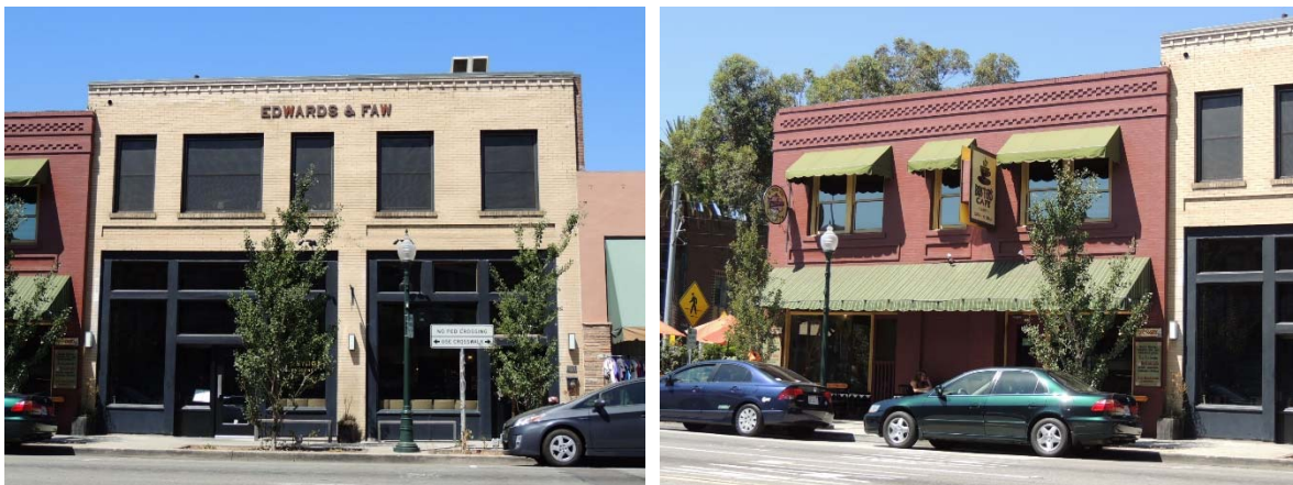
Figure 61. L: Edwards Faw Building, 1912, 1008 Mission. R: Shapiro Building, 1915, 1002 Mission. Photographs 2014; source: Historic Resources Group.
