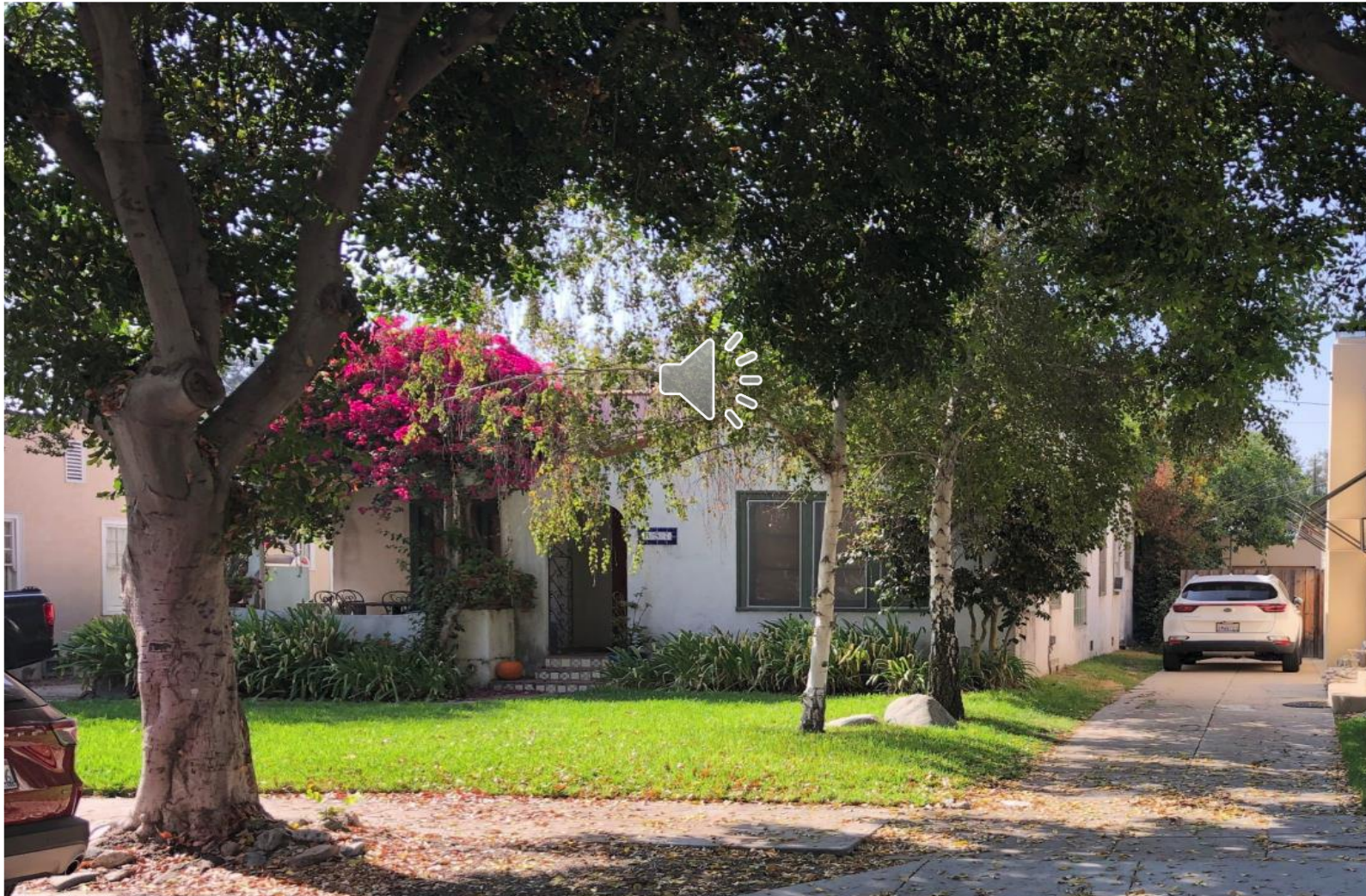
Figure 2: Street Elevation, 657 Forest Avenue
