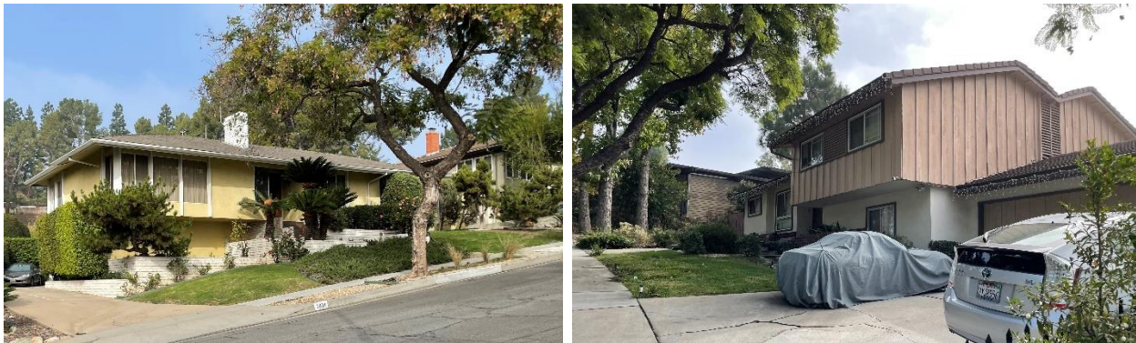
Figure 8: Residences with Overhangs on Nearby La Fremontia Street
