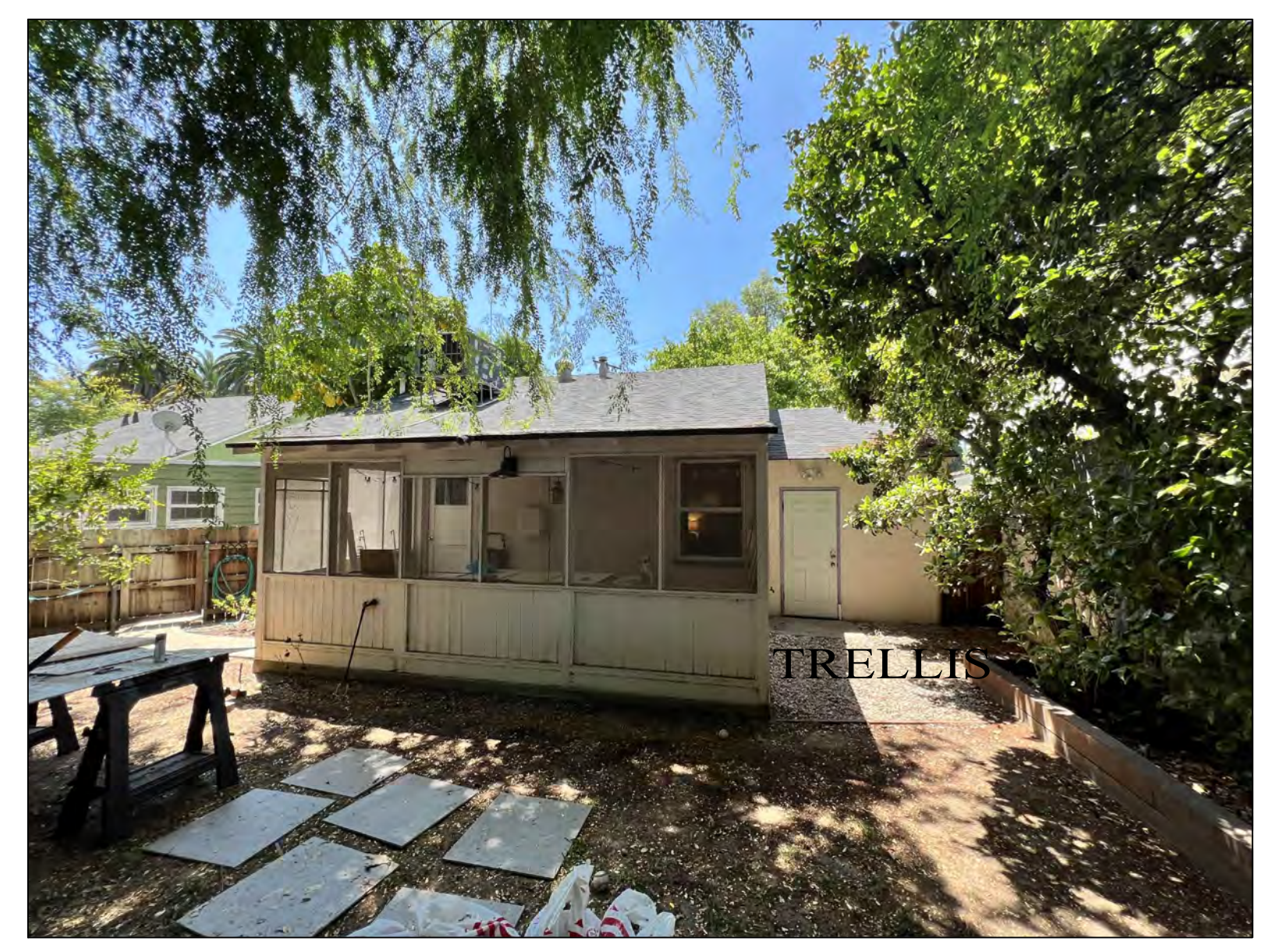
EXISTING HOUSE REAR VIEW
