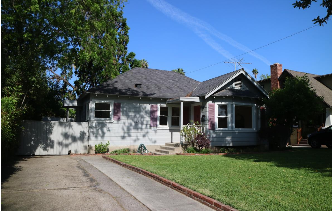
Figure 5 Façade, from southeast (top), north elevation, from northeast (bottom)
