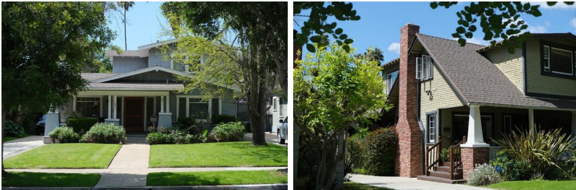
Figure 14 Potential noncontributors to Marengo School Craftsman District, due to alterations; 1311 Stratford (left) and 1315 Stratford (right, adjacent to subject property)
