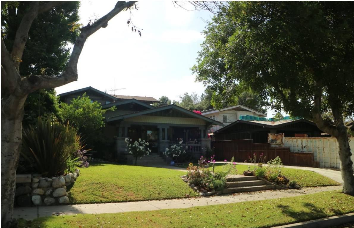
Figure 17 2nd-story additions in 1300 block of Stratford Avenue; 1312 Stratford (1913, on left), 1314 Stratford (1914, on right, addition under construction), northwest perspective
