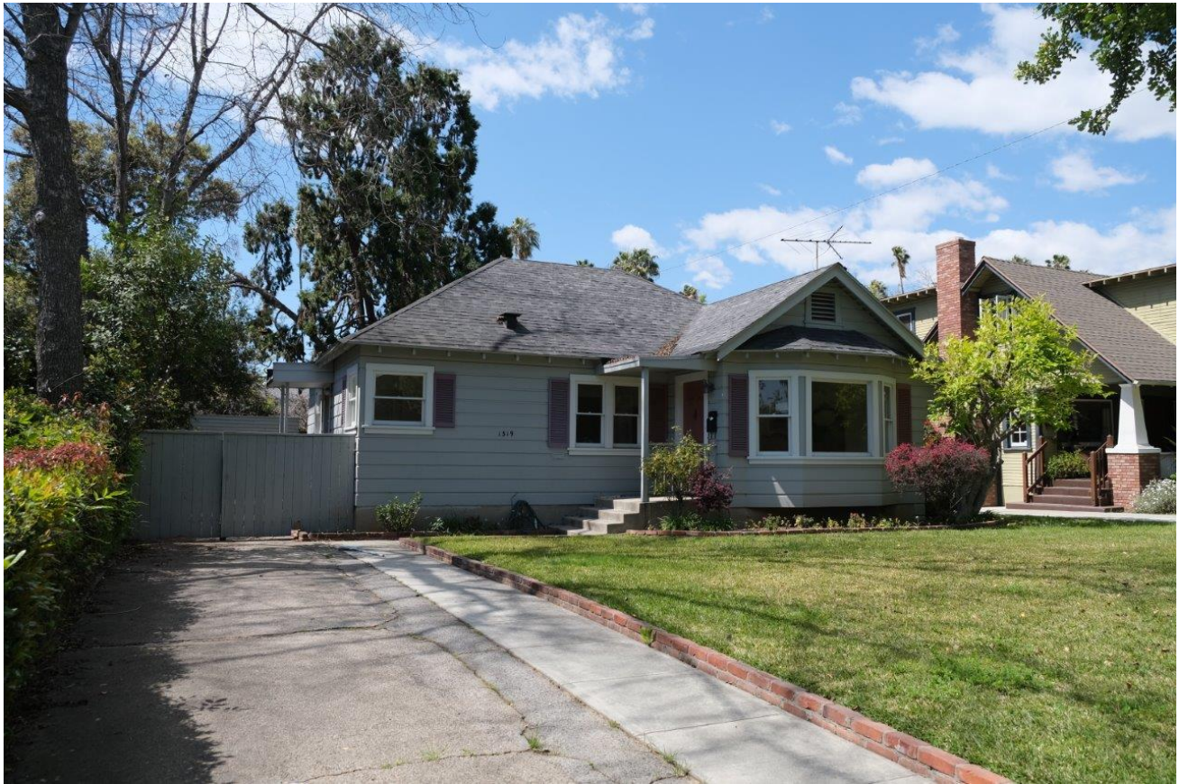
Figure 2: Street View of Existing House
