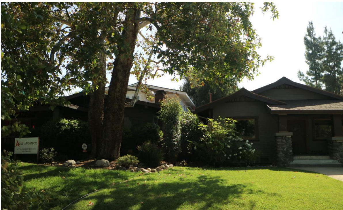
Figure 18 View from west perspective of 1318 Stratford and 2nd-story addition to 1314 Stratford Avenue
