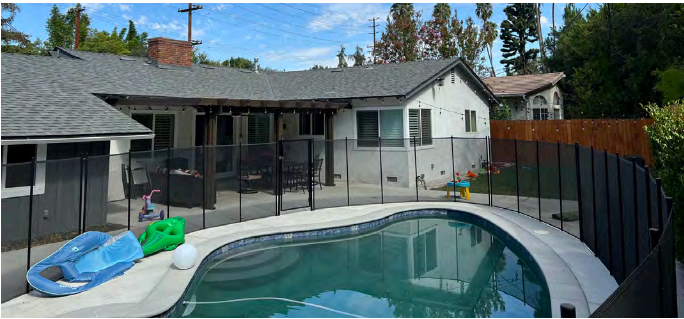
EAST ELEVATION LOOKING NORTH
