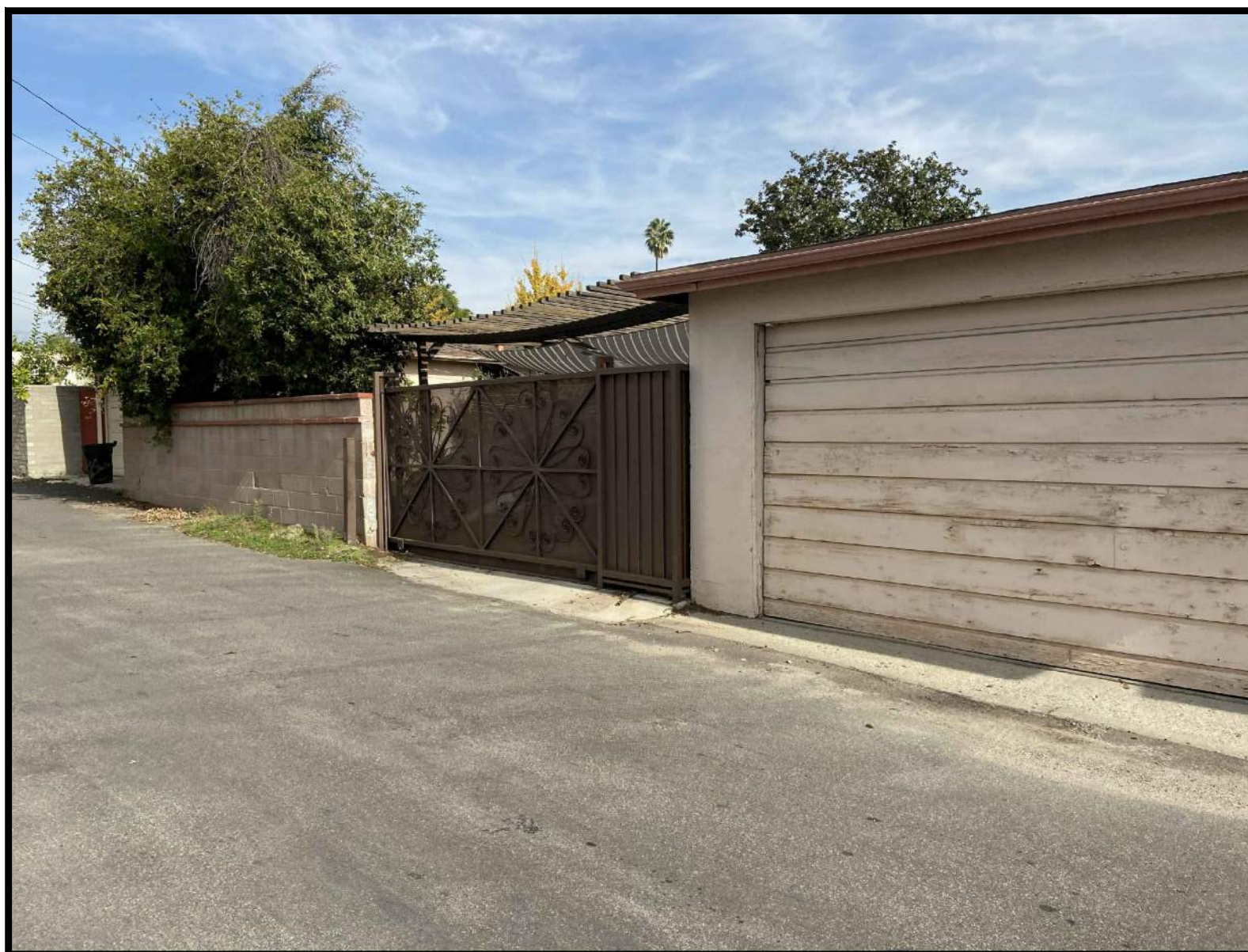
CARPORT ENTRANCE GATE FROM ALLEY C4
