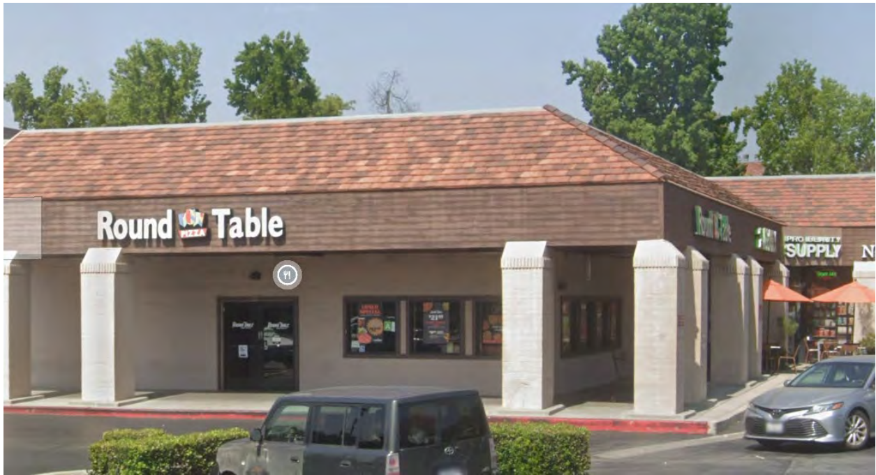
Figure 2: Existing Building with Clay-tiled Roof, Wood Fascia, and Brick Columns
