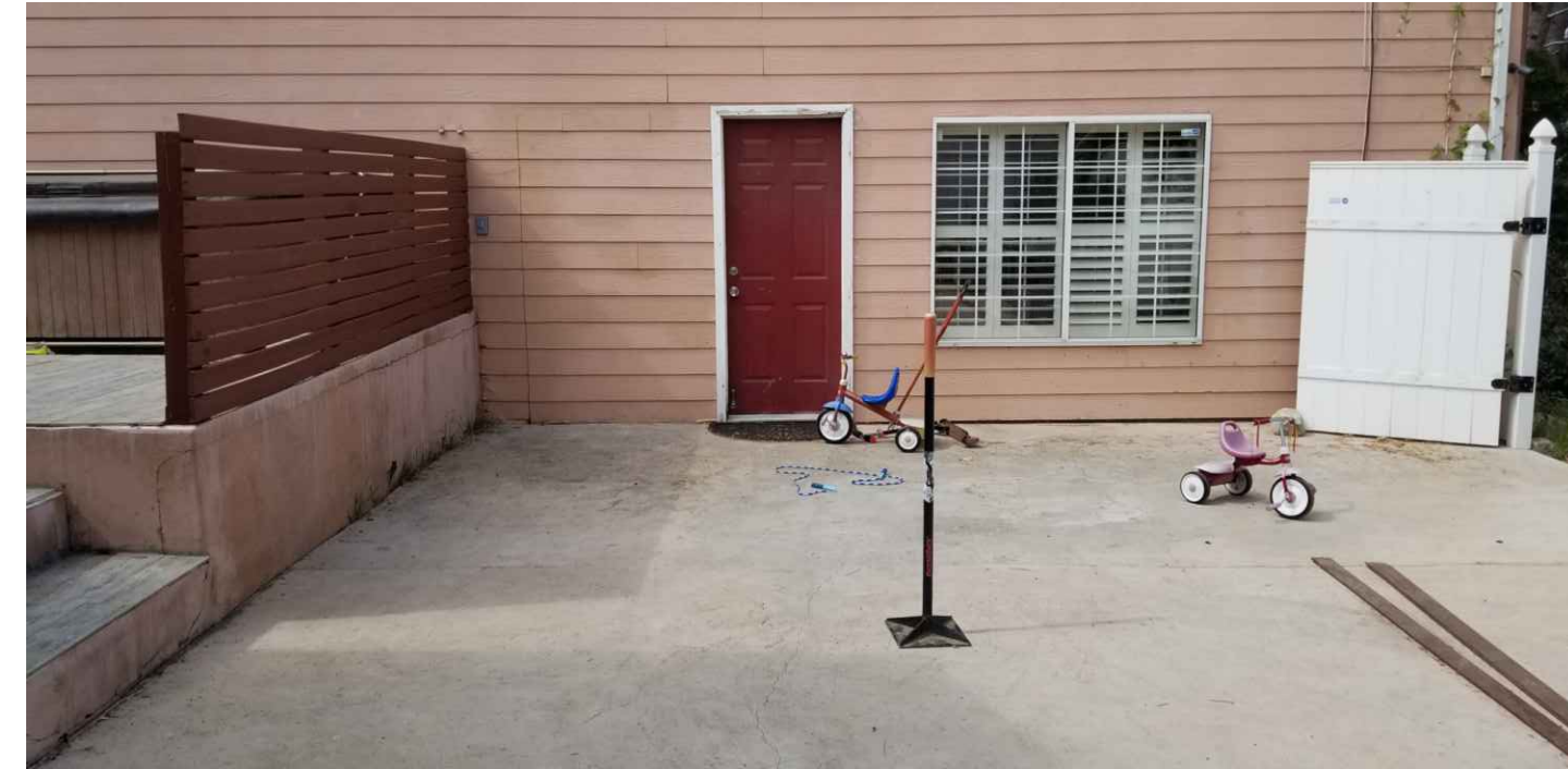
7. EXISTING NORTH FACADE
