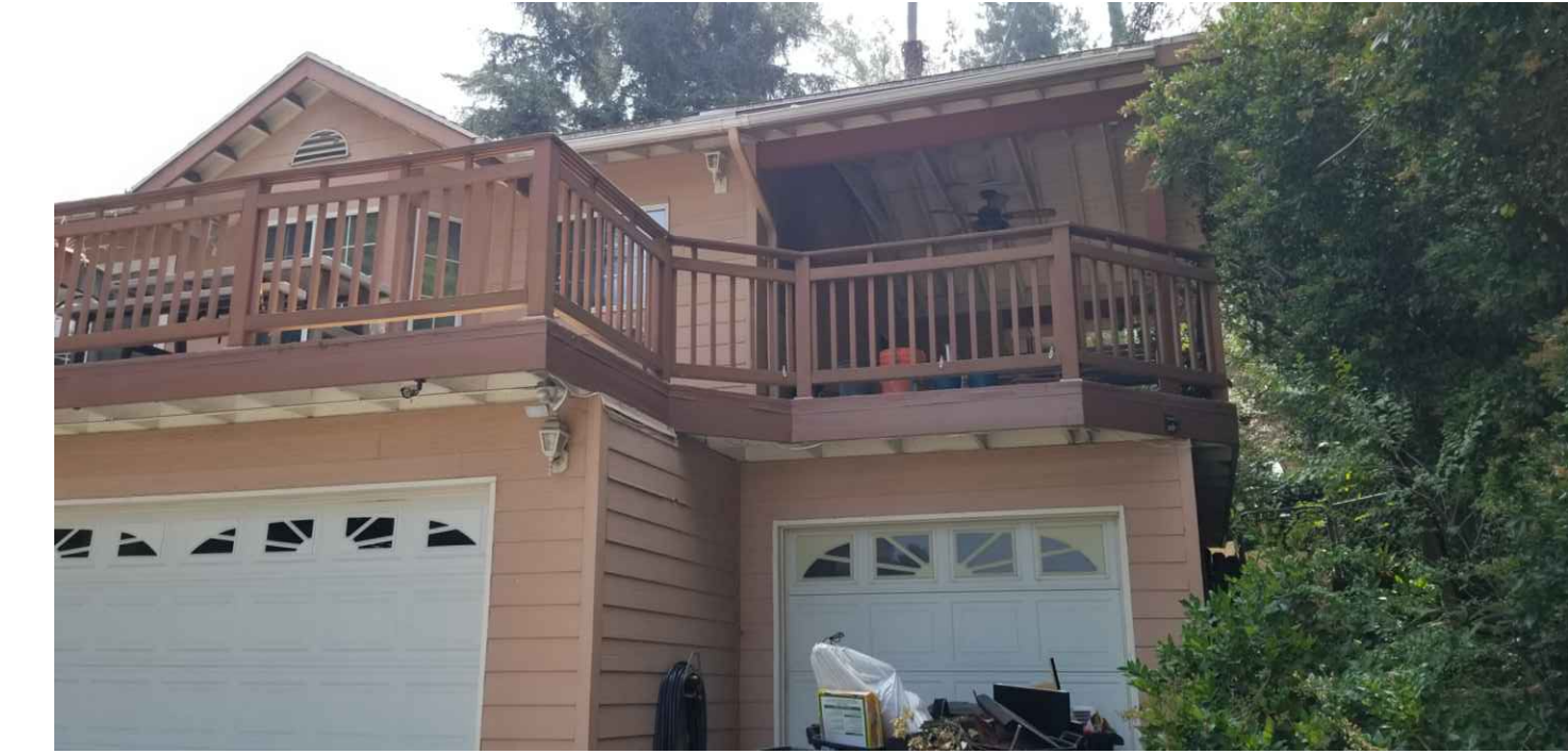
1. EXISTING WEST FACADE
