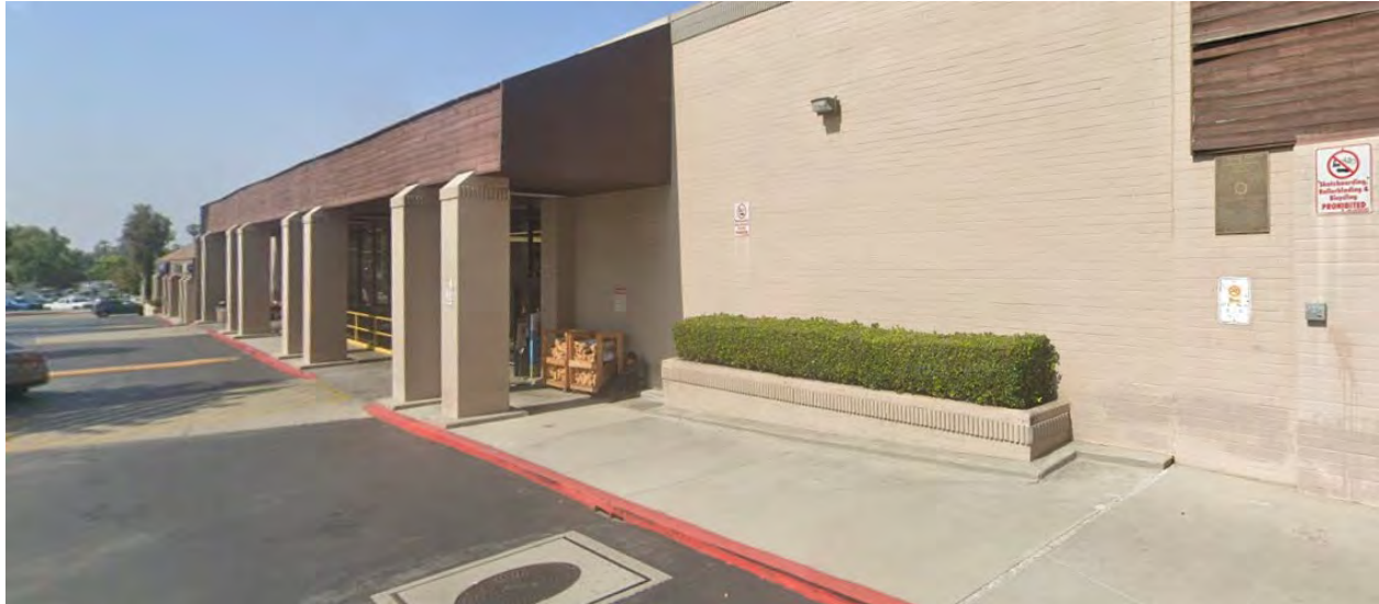
Figure 4: Image of Existing “Shoulder” Columns
