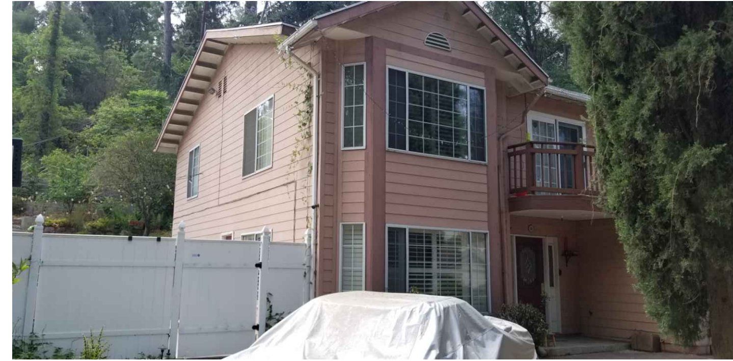
6. EXISTING WEST FACADE
