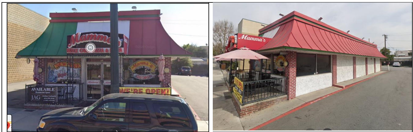
Figure 2: View of Existing – West (Front) and Southwest Elevations
