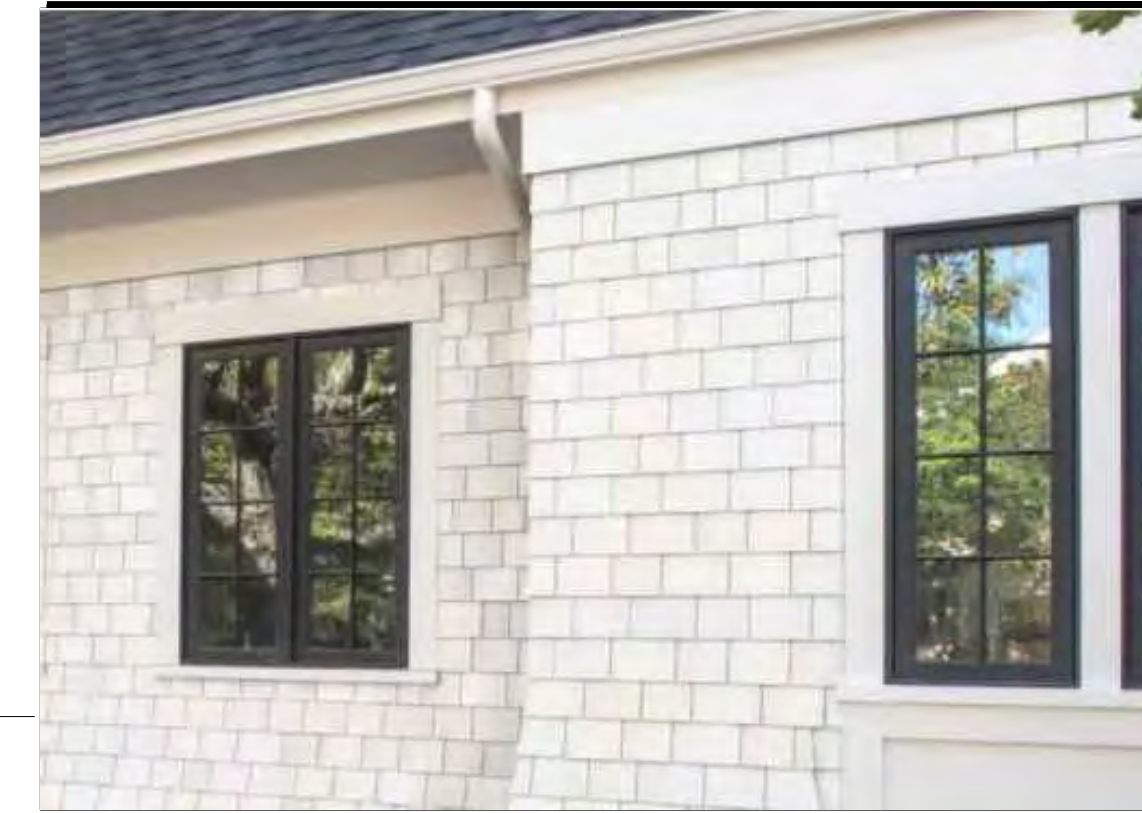
(N) HARDI-SHINGLE SIDING -WHOLE HOUSE
