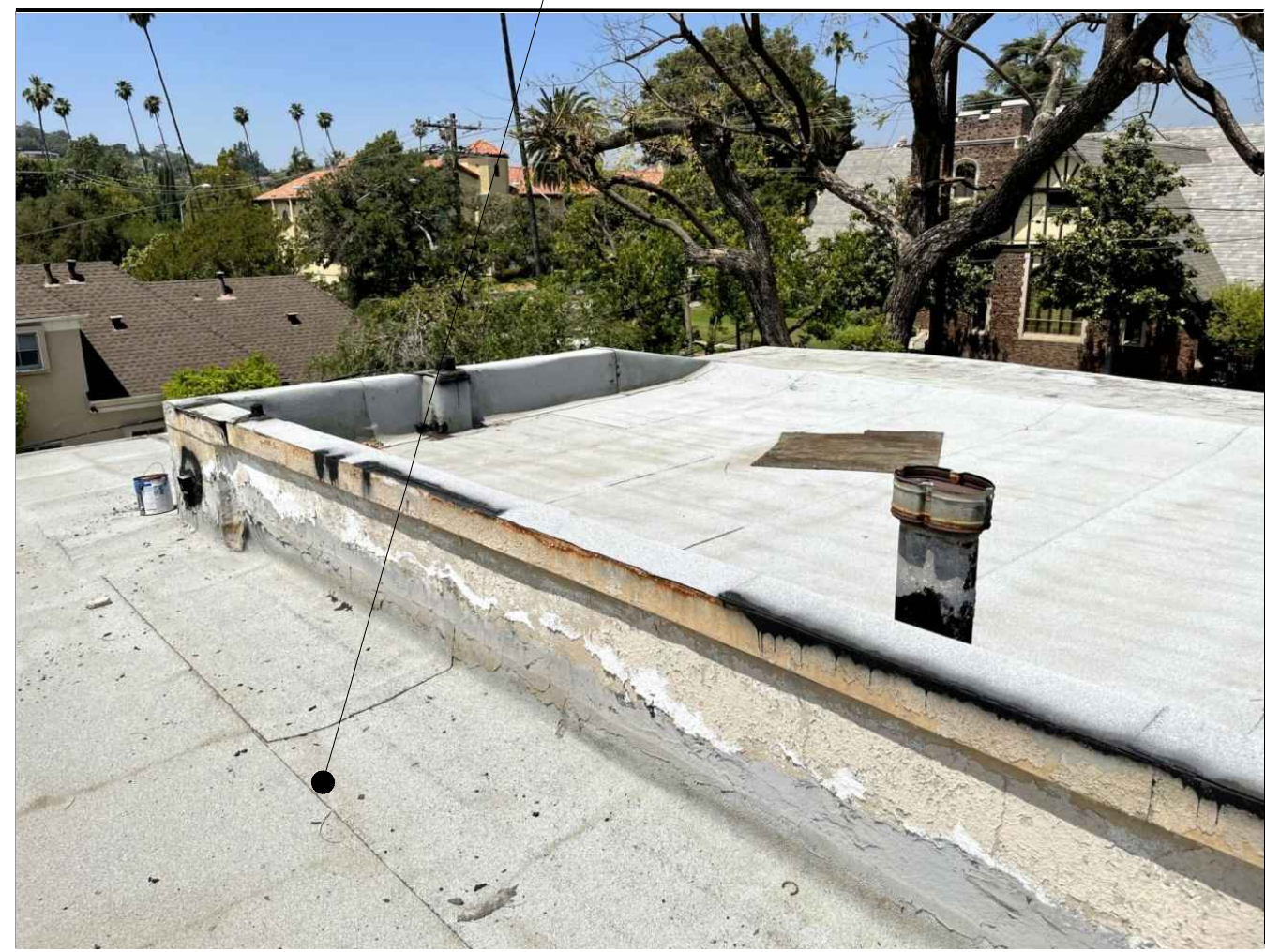
ROOF RAFTER CONDITION
