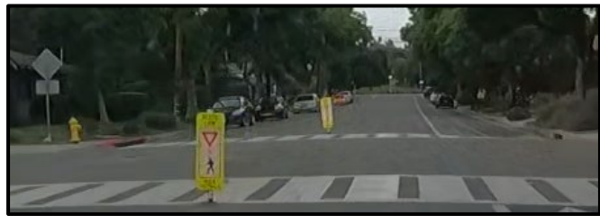
Typical In-Pedestrian Crossing Signs on Crosswalks
