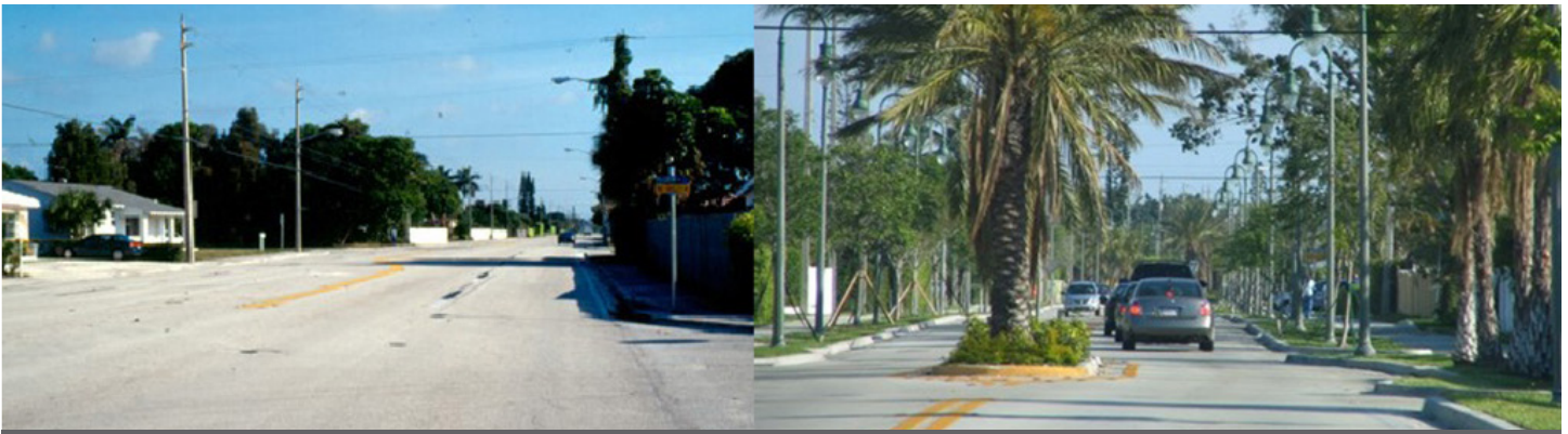
Figure 11: Before and After a Road Diet of a Five-Lane Arterial in West Palm Beach
