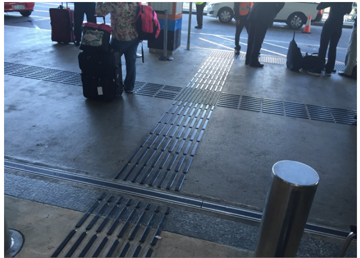
Figure 66: Example of Guide Strips
