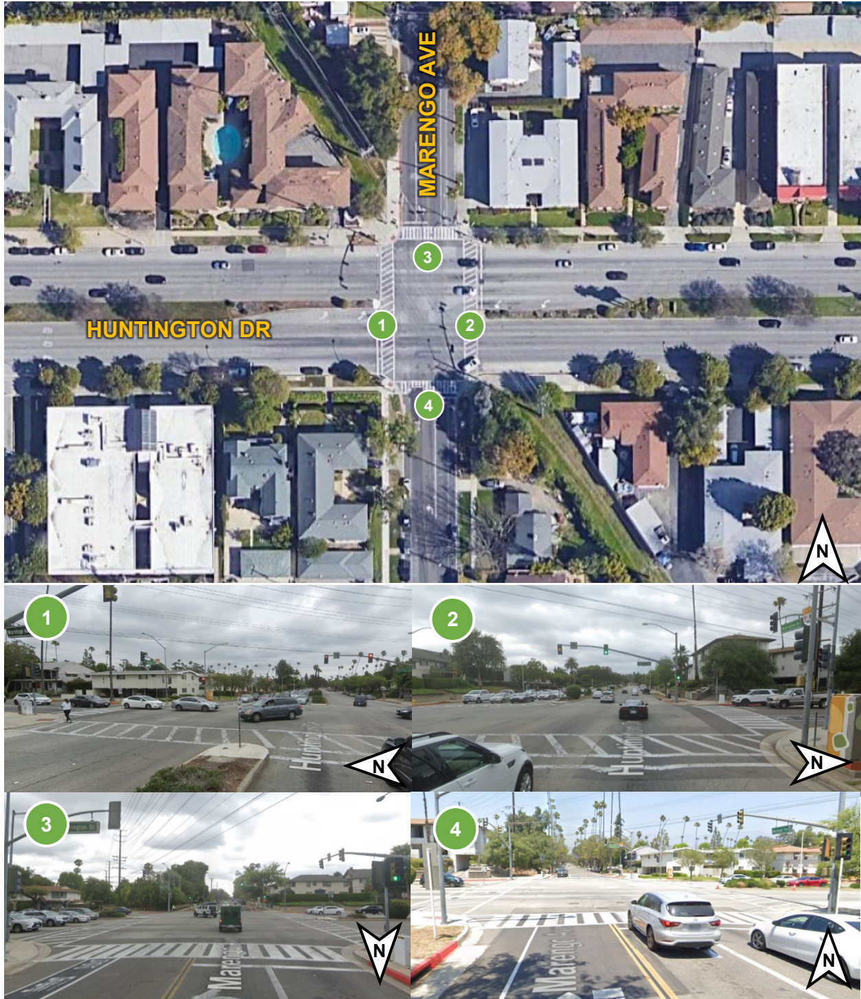
Figure 2: Driver Visibility of Huntington Dr & Marengo Ave Crosswalks
