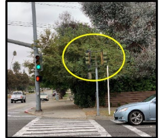
Southwest Corner – Eight Inch Vehicle Heads for North/South
