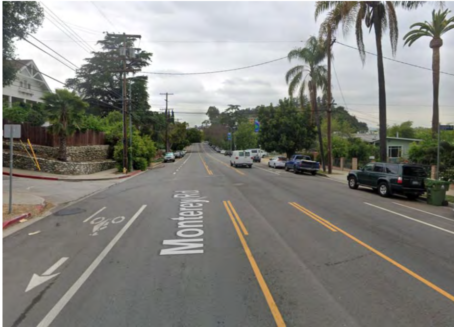
Existing Condition: Class II Bike Lane on Monterey Road in City of Los Angeles
