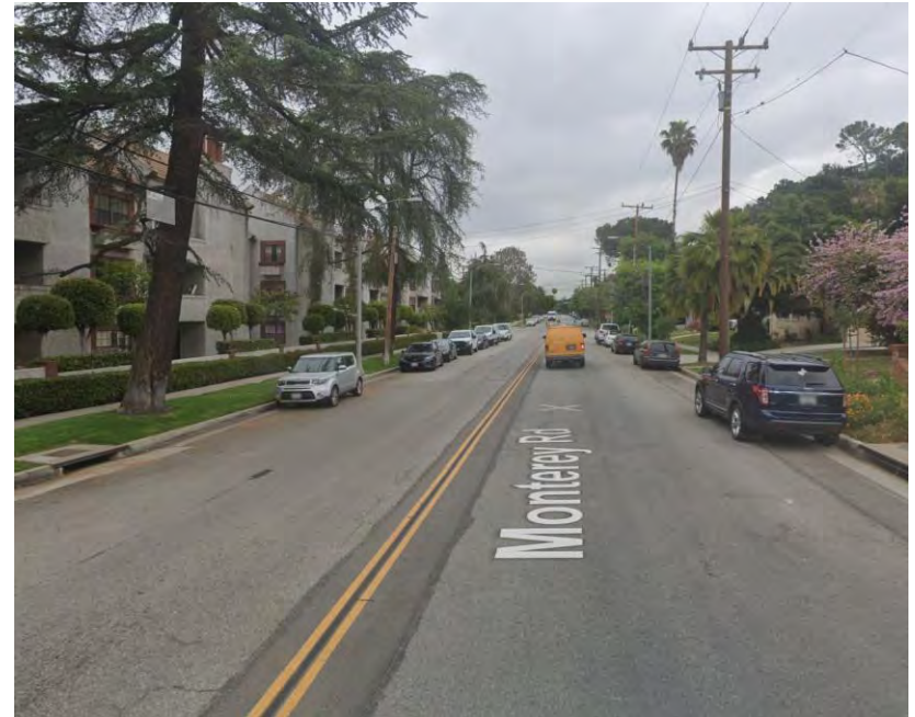
Existing Condition: Monterey Road in City of South Pasadena
