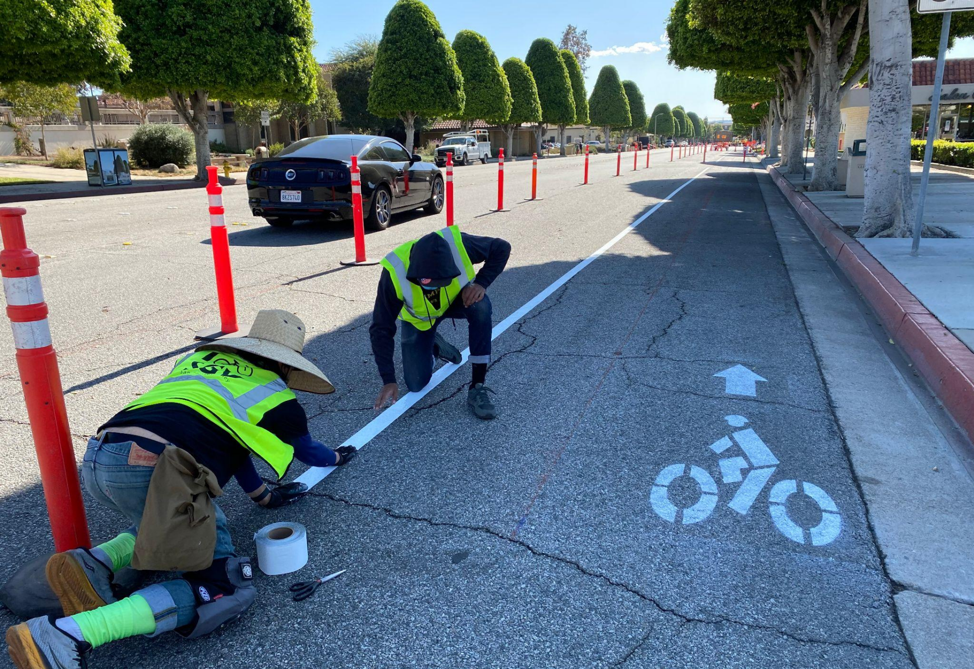
Demo utilizes temporary, reflective, white and yellow "lane tape" - Glendora, CA (2020)
