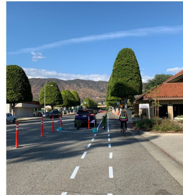
Temporary protected bicycle lane on Glendora Avenue from Ada to Foothill
