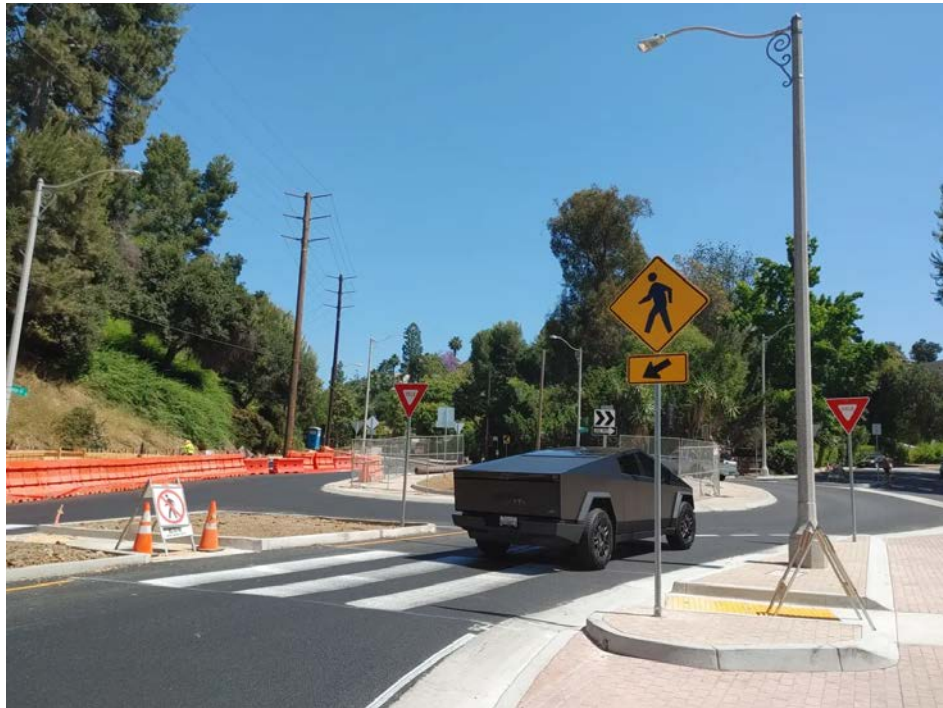
The roundabout at Avenue 64 and Burleigh Drive in Pasadena. Credit: Chris Greenspon/SBLA
