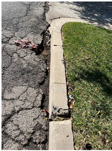
Gutter Erosion, curb damage
