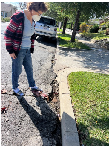
Gutter Erosion, curb damage
