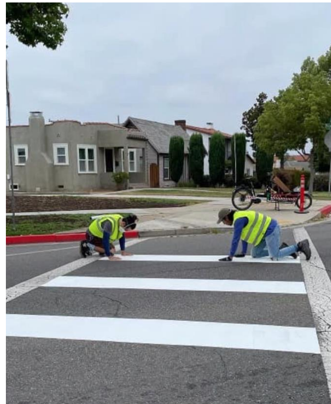
Glendora demonstration utilized temporary materials: reflective, white and yellow "lane tape"; heavy-duty, crash-resistant security planters; reflective delineators.
