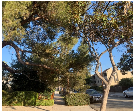
The large branch near the ground leans on utility lines but cannot be removed without destabilizing the tree. (View east)
