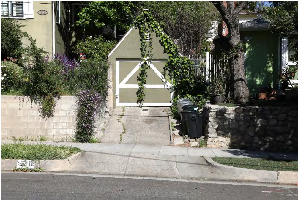
Garage, view facing east.
