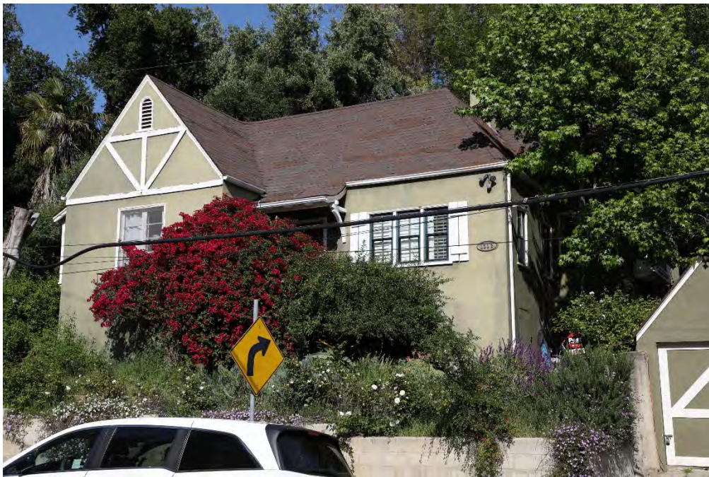
West and south facades, view facing northeast.
