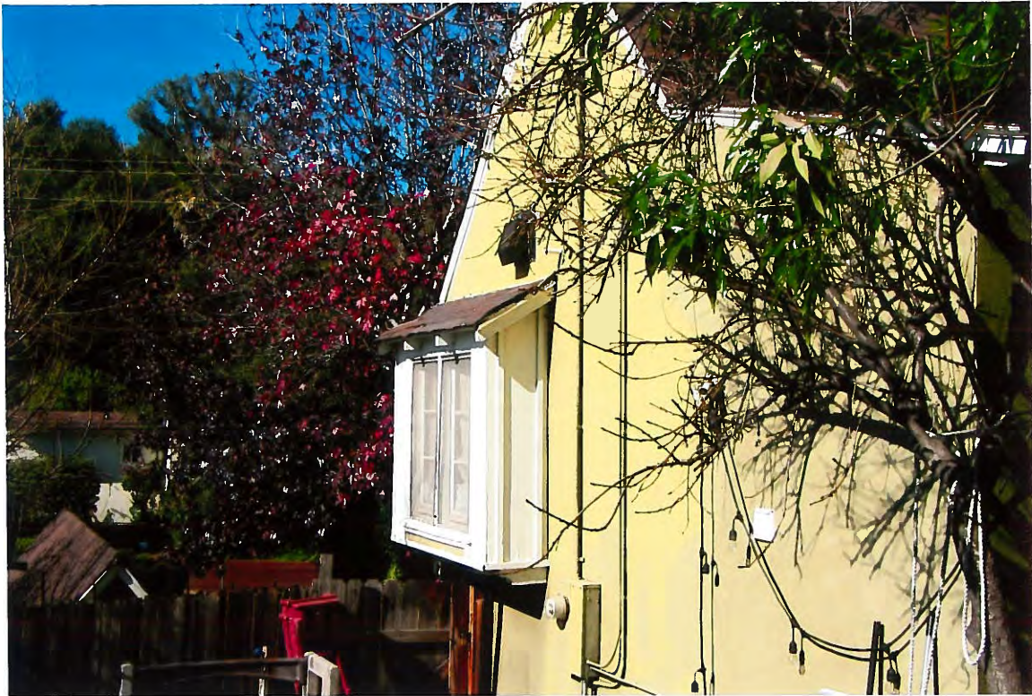
Side of house facing West Side gate
