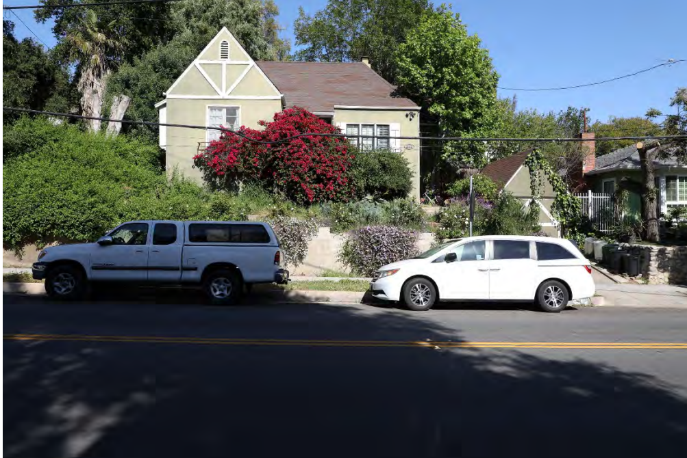
Primary (west) façade, view facing east.
