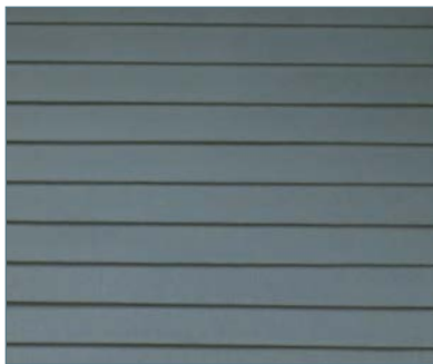
Wood clapboard siding
