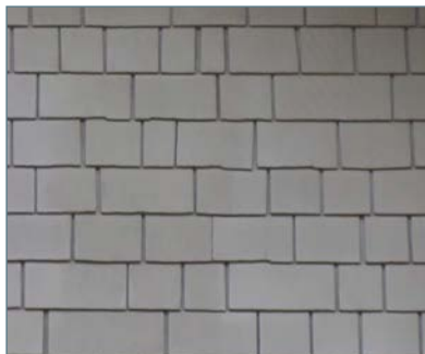
Wood shingle siding (coursed)
