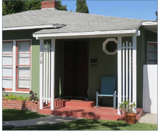
Partial-width projecting porch
