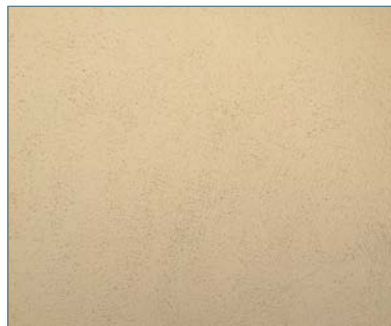
Stucco cladding (sand/float finish)
