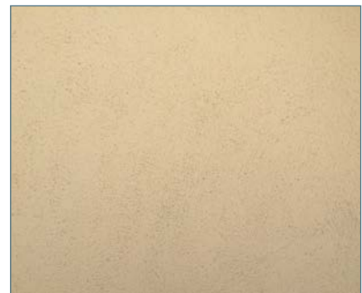
Stucco cladding (sand/float finish)
