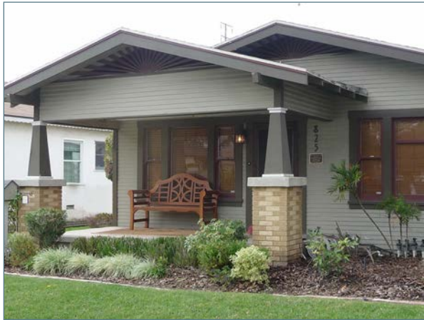
Partial-width projecting porch
