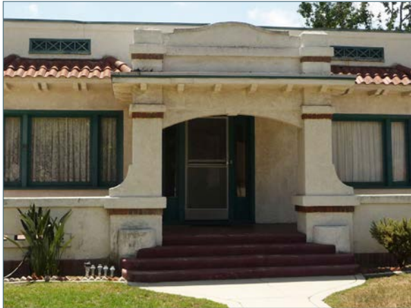
Partial-width projecting porch
