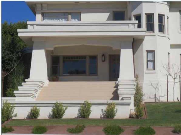
Partial-width projecting porch
