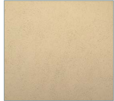
Stucco cladding (sand/float finish)
