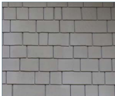
Wood shingle siding (coursed)
