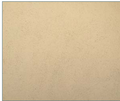
Stucco cladding (sand/float finish)
