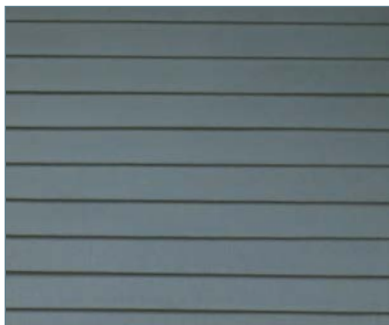
Wood clapboard siding
