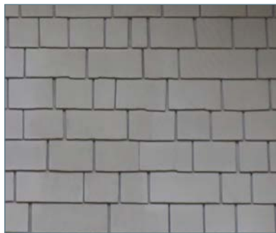
Wood shingle siding (coursed)
