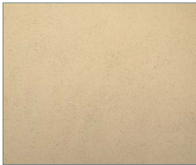
Stucco cladding (sand/float finish)
