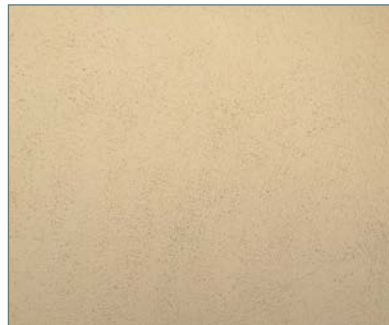
Stucco cladding (sand/float finish)
