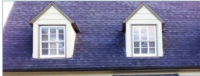
Multiple gable roof dormers
