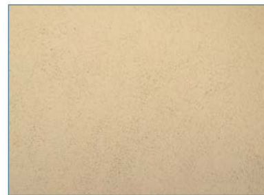
Stucco cladding (sand/float finish)
