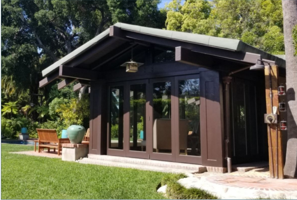
Example of new detached ADU located on a Craftsman residential property (courtesy of Louisa Van Leer Architecture)
