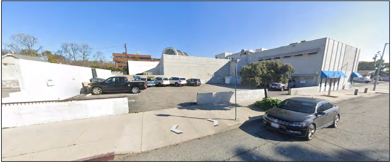
Figure 4. Looking northeast from Hope Street
