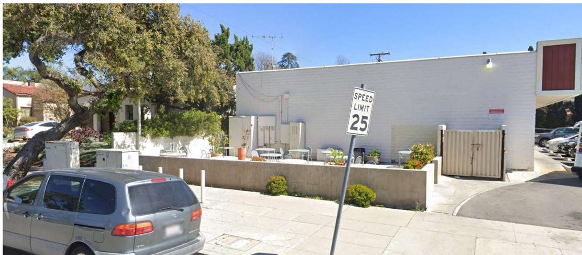
Figure 2. Senor Fish 12 outdoor patio tables directly adjacent to a single-family residential property.
