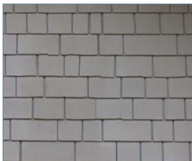
Wood shingle siding (coursed)
