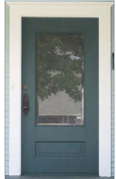
Paneled wood door with glazing
