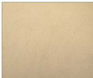
Stucco cladding (sand/float finish)
