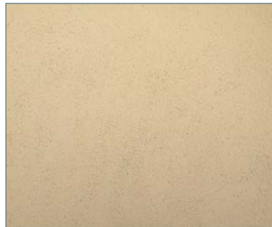
Stucco cladding (sand/float finish)
