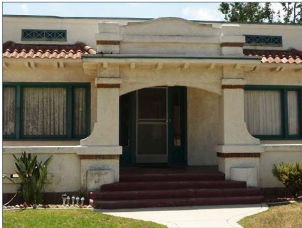
Partial-width projecting porch
