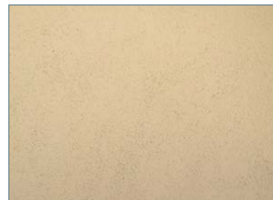
Stucco cladding (sand/float finish)
