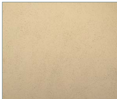
Stucco cladding (sand/float finish)
