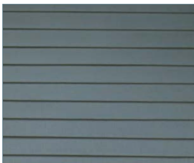
Wood clapboard siding
