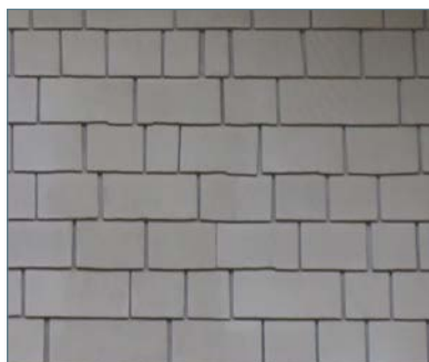
Wood shingle siding (coursed)
