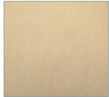
Stucco cladding (sand/float finish)
