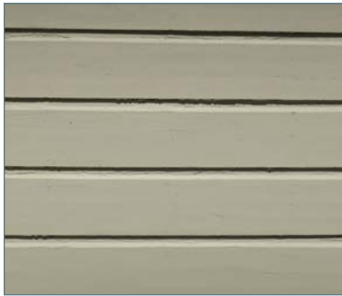
Horizontal wood channel siding
