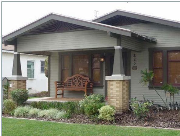
Partial-width projecting porch
