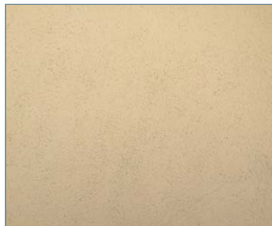
Stucco cladding (sand/float finish)
