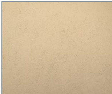
Stucco cladding (sand/float finish)
