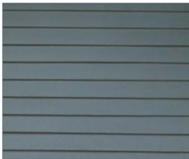
Wood clapboard siding
