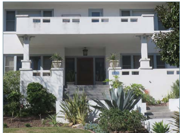
Partial-width projecting porch with low stucco wall
