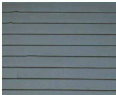
Wood clapboard siding
