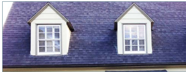
Multiple gable roof dormers
