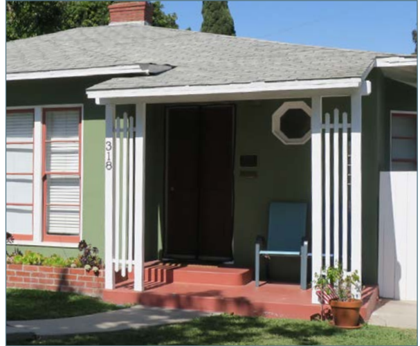
Partial-width projecting porch
