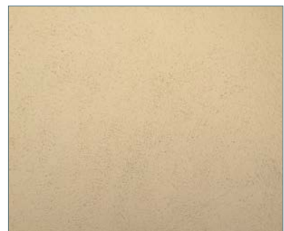
Stucco cladding (sand/float finish)
