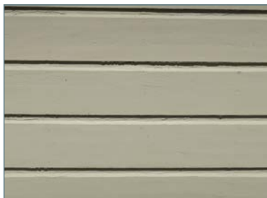
Horizontal wood channel siding
