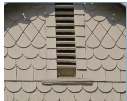
Wood shingle siding (variegated)
