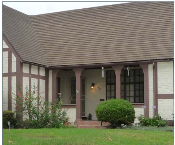
Recessed entrance porch
