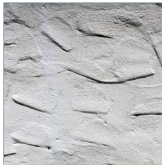
Stucco with different trowel patterns
