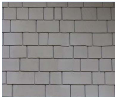
Wood shingle siding (coursed)
