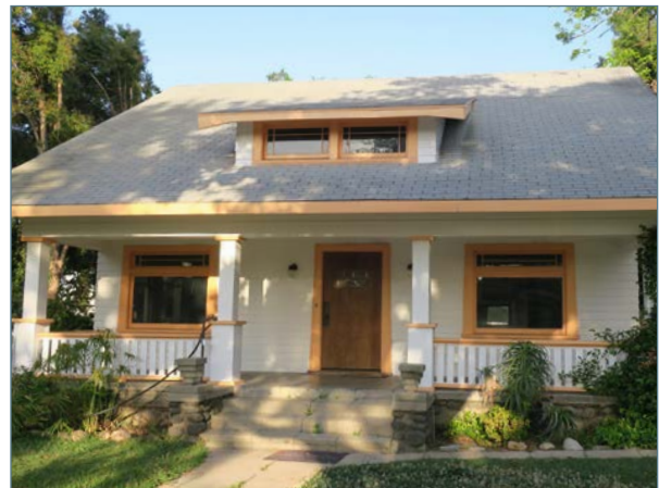
Full-width porch with wood railing
