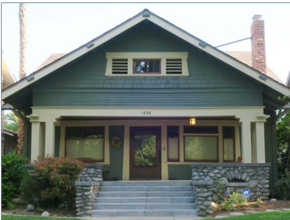
Full-width porch with low stone wall
