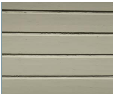
Horizontal wood channel siding
