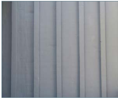
Vertical wood board-and-batten siding
