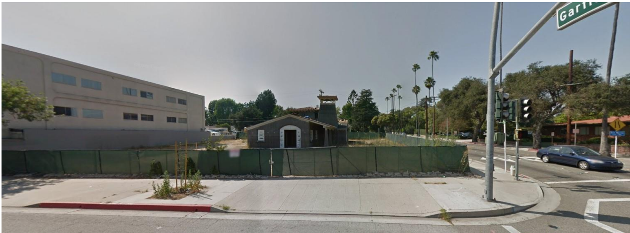
Photo 3: the abandoned and unfinished carwash structure as seen in 2012 (photo credit: Google Maps).
