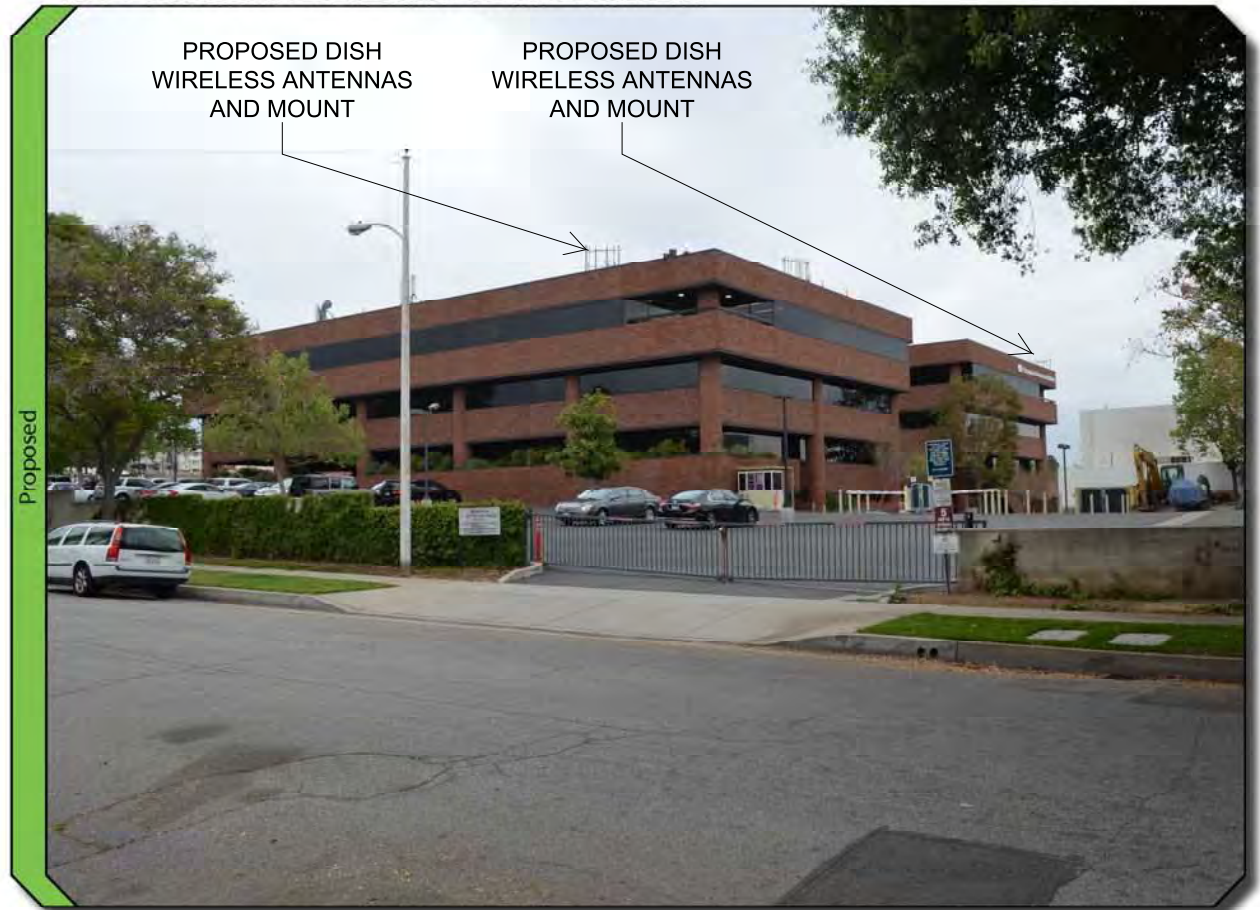
View 3 of 3: SOUTH WEST ELEVATION LOOKING NORTH EAST
