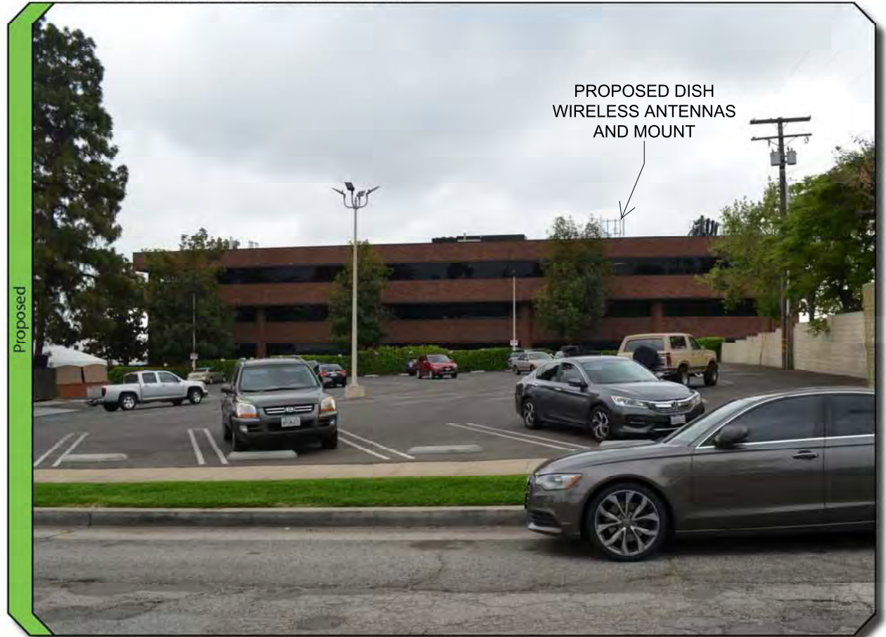
View 1 of 3: NORTH ELEVATION LOOKING SOUTH
