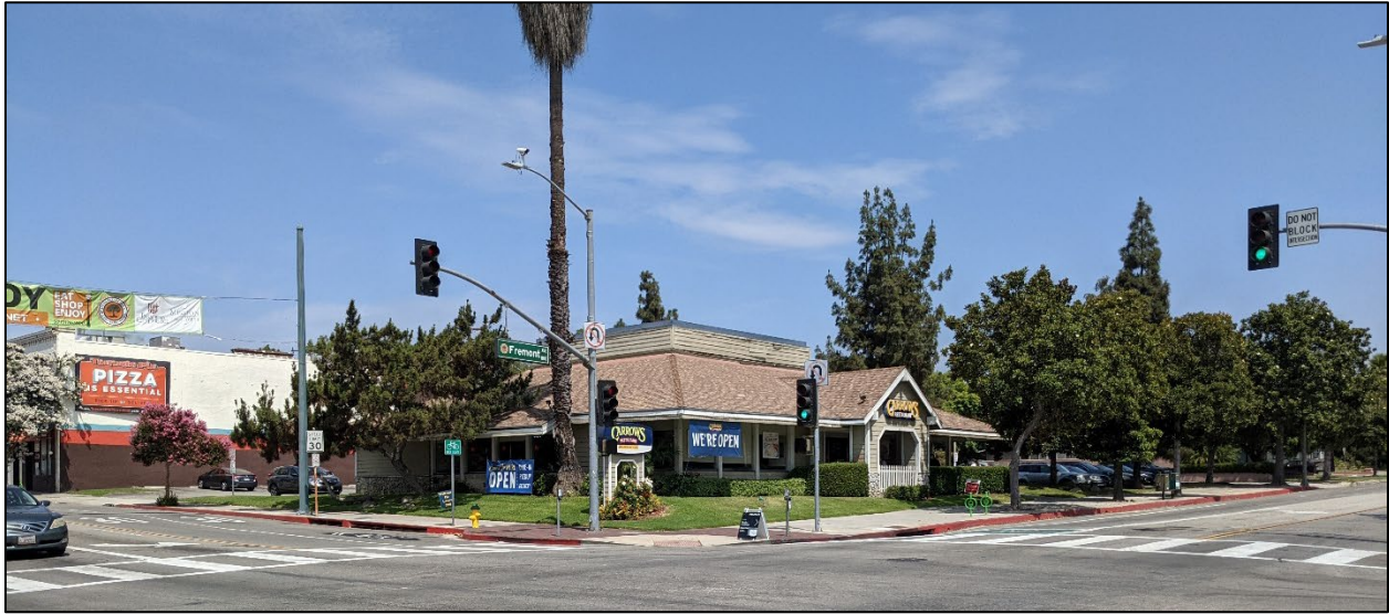
Project Site – northwest corner of Mission Street and Fremont Avenue. Figure 2
