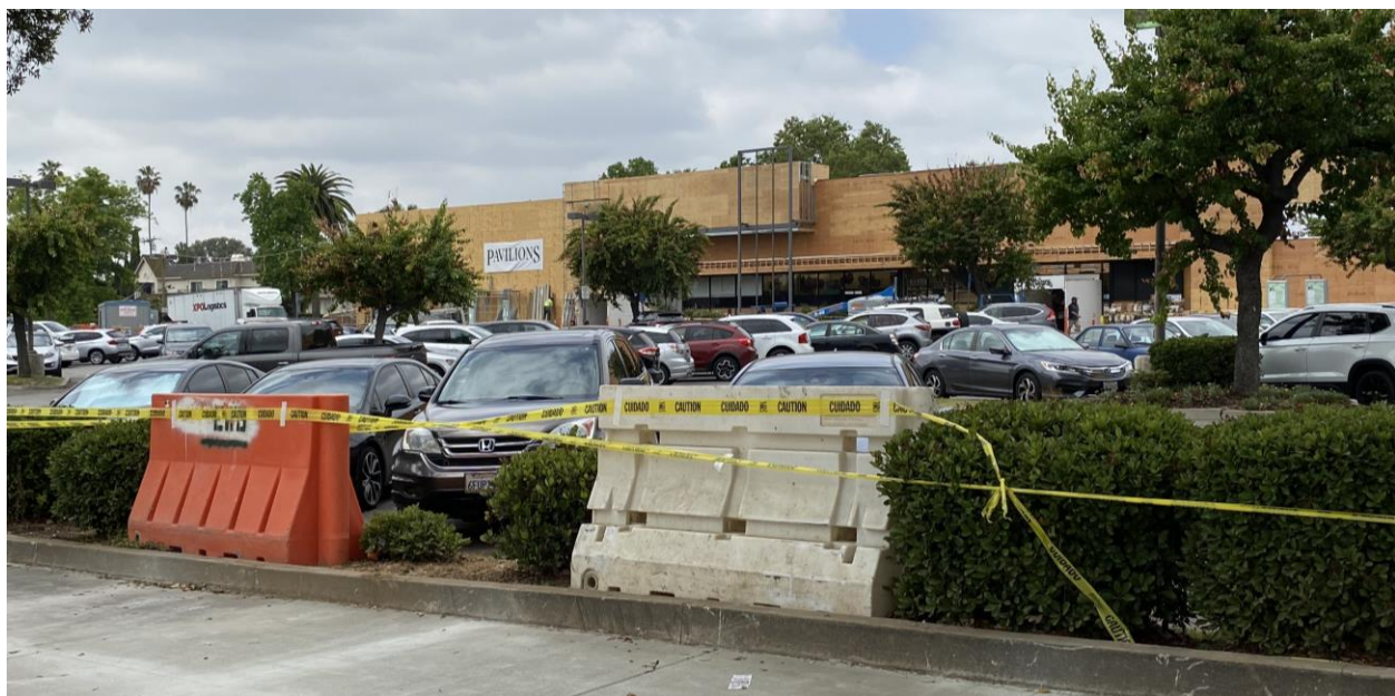
Figure 4: Street View of Project Site
