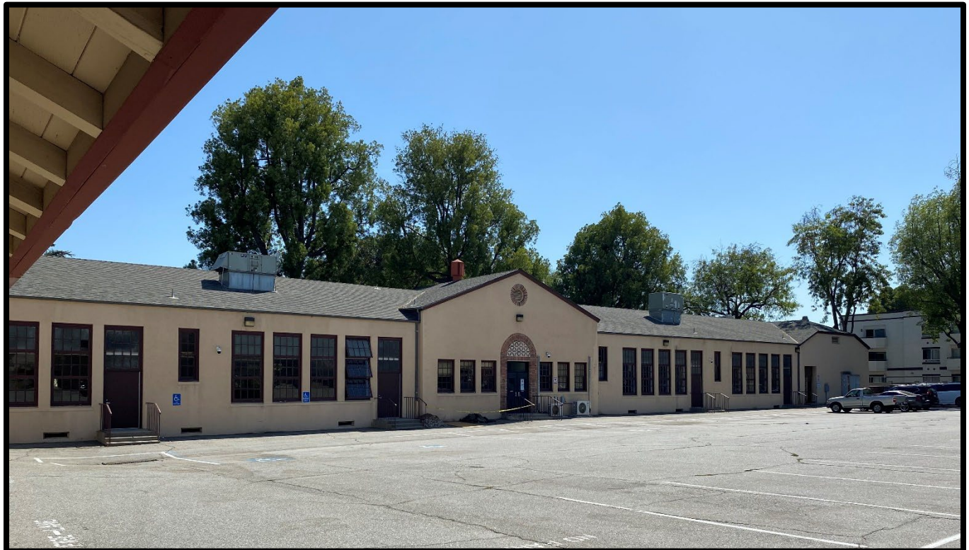
Figure 3: View of the Existing Parking Lot
