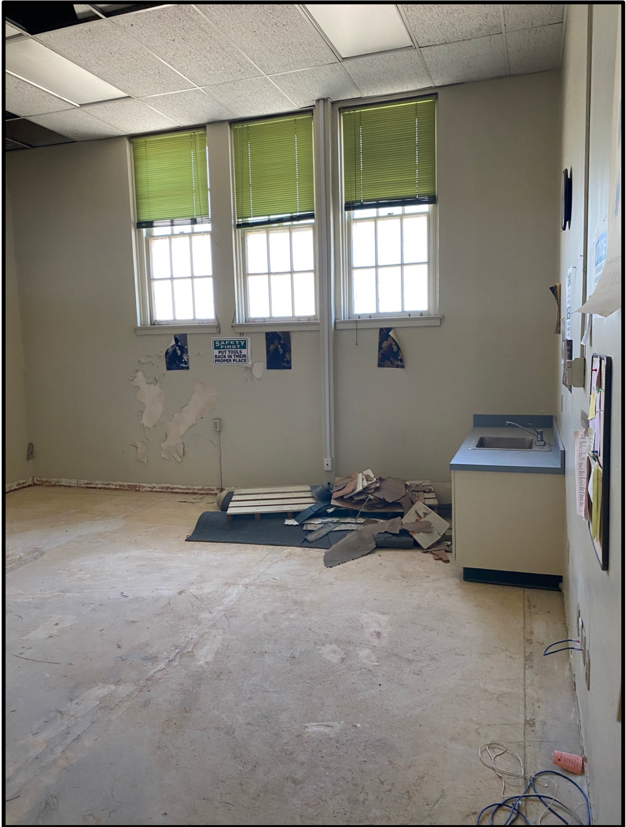
Inside Former Classroom
