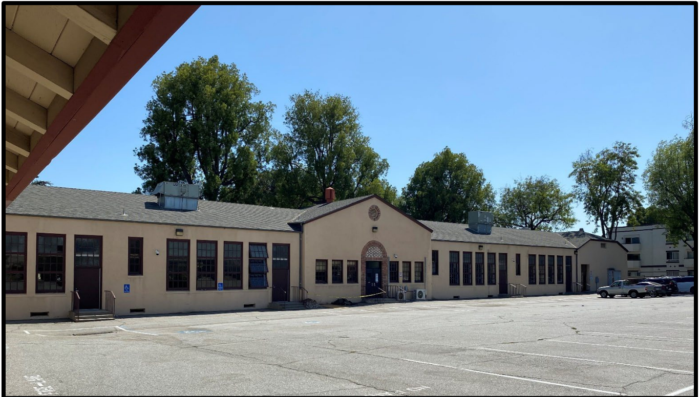
Figure 3: View of the Existing Parking Lot
