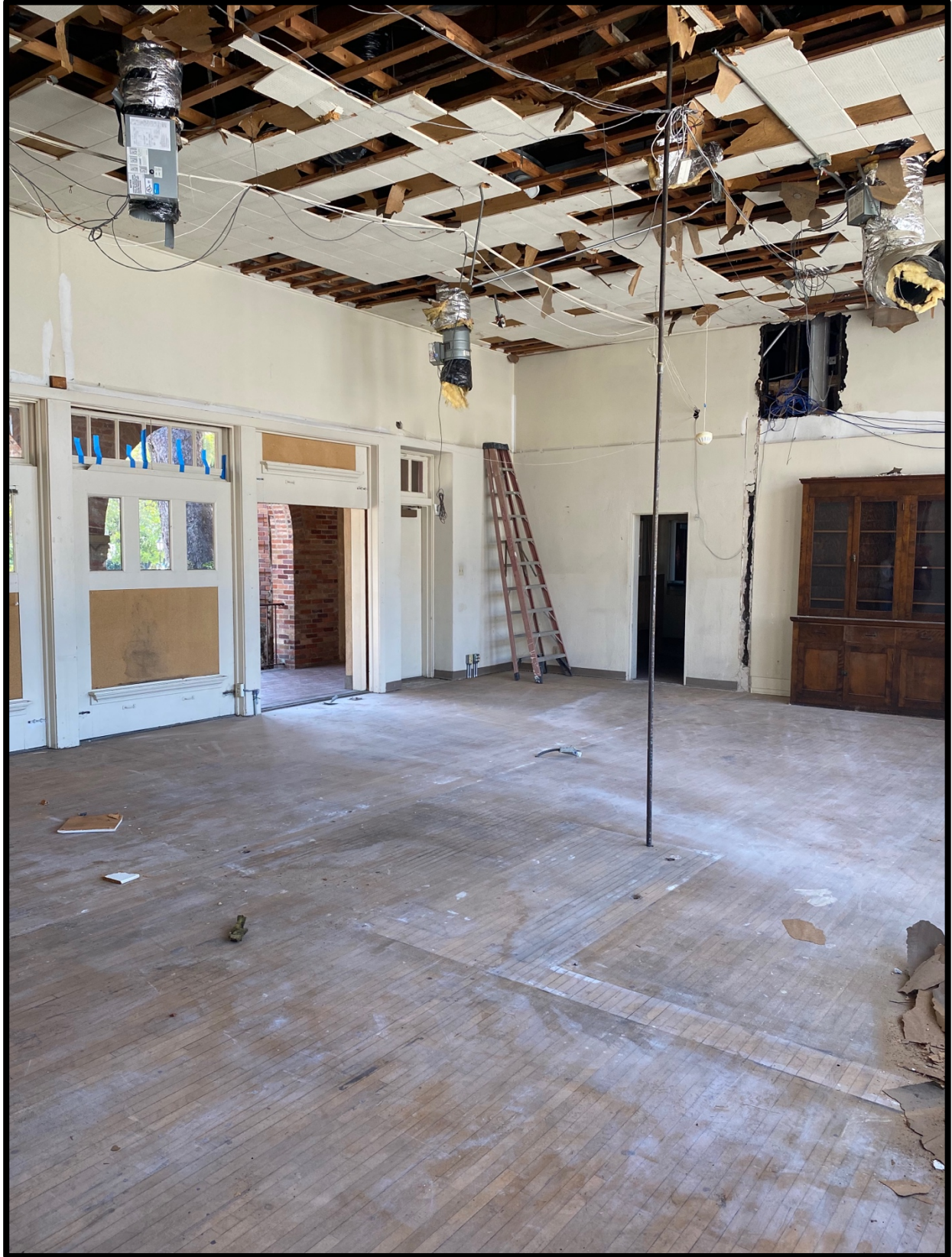
Inside Former Classroom
