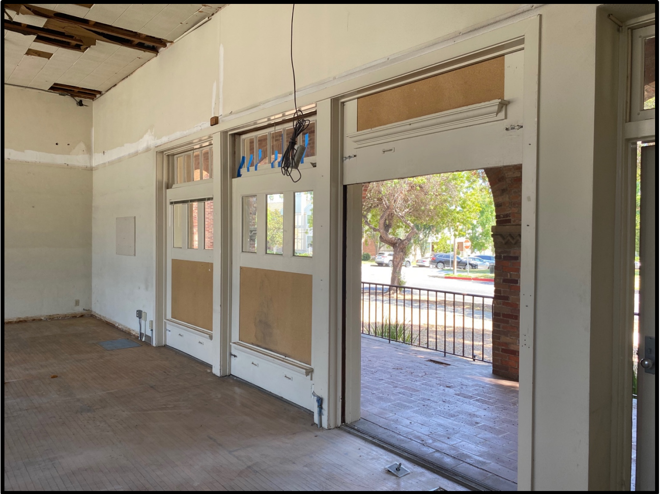
Former Classroom Doors: Interior
