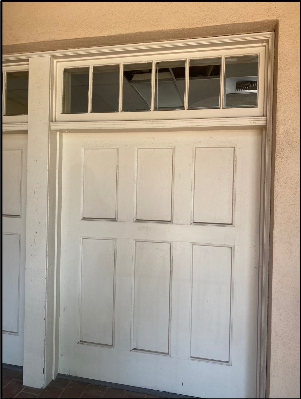
Former Classroom Door
