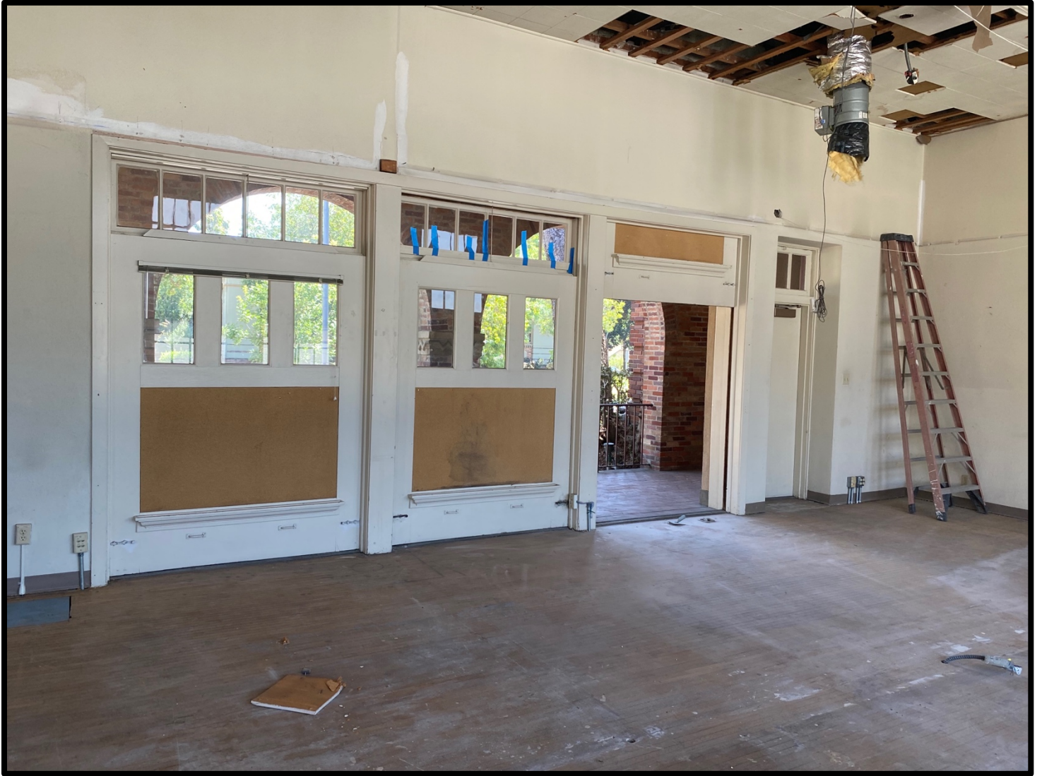
Former Classroom Doors: Interior
