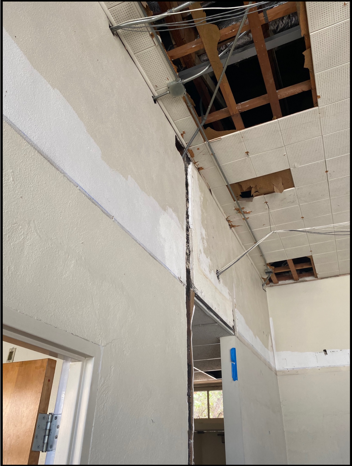
Classroom Partition Walls
