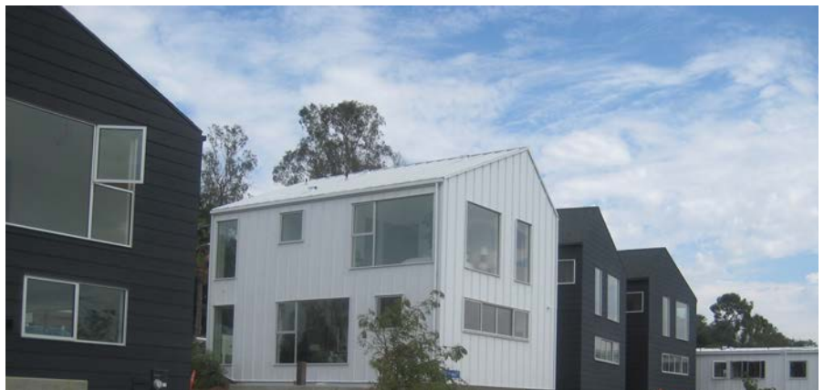
The Blackbirds Small Lot Development (below) in Echo Park features a pitched roof.
