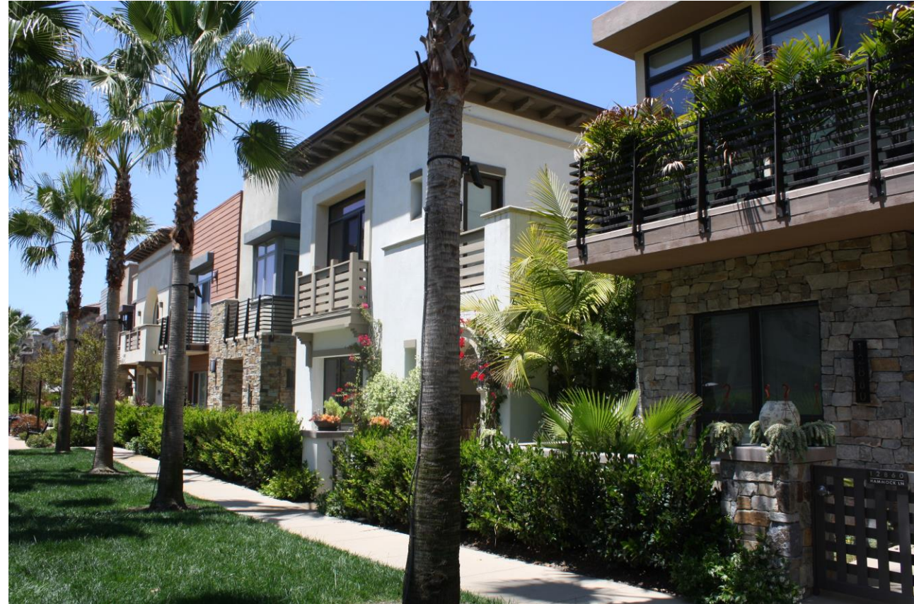
Ground floor apartment windows recessed over 2 inches and glazing that maintains transparency to the street. Landscaping is used in this example to provide privacy.
