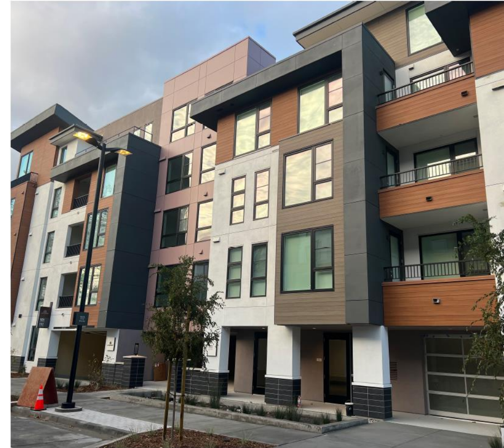
A façade using modulation, recessing and materials to create visual interest.
