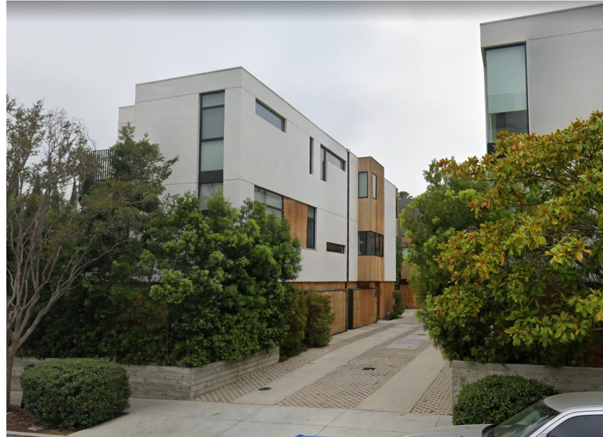
A multi-use driveway providing common open space for residents.
