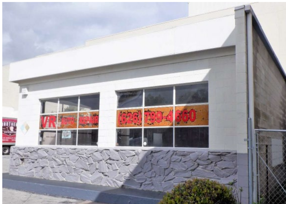
Figure 4: Repair Service Garage
