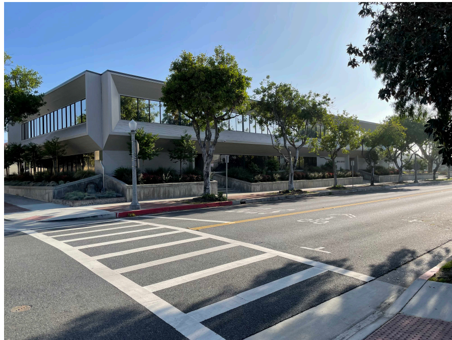
15) ADJACENT BUILDING @ EL CENTRO & FAIRVIEW
