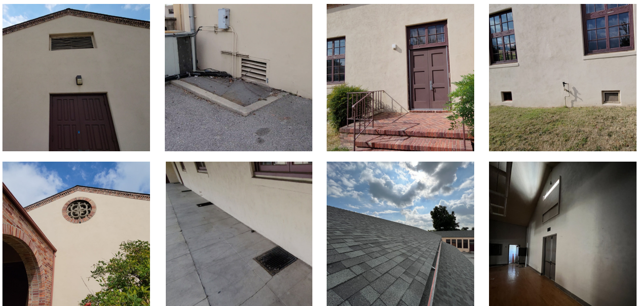
Figure 4.2 - Observed Site Conditions Noted As Being Sound Paths For Noise Egress
