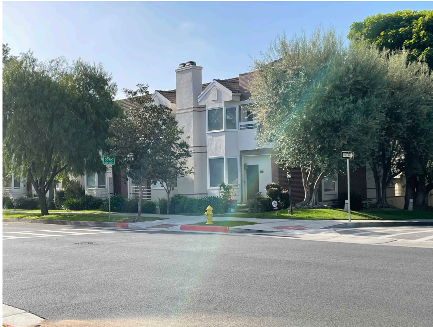
14) ADJACENT BUILDING @ EL CENTRO & FAIRVIEW
