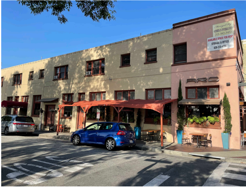
18) ADJACENT BUILDING @ DIAMOND & MISSION
