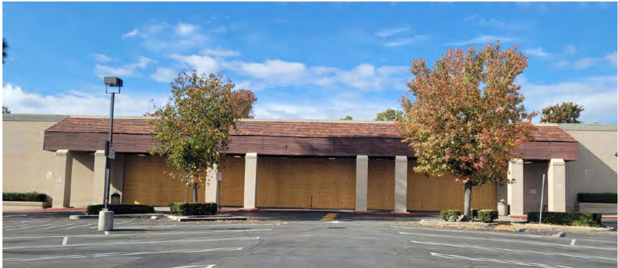
Figure 3: Street View of Project Building
